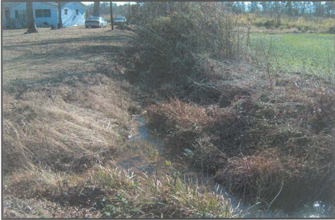
Photo 1 – Beginning of restoration reach, looking south.
