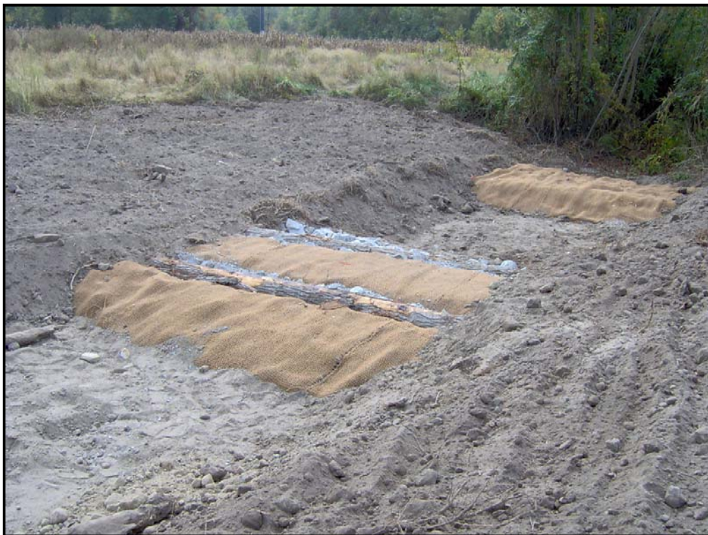
Grade Transition – Facing upstream
