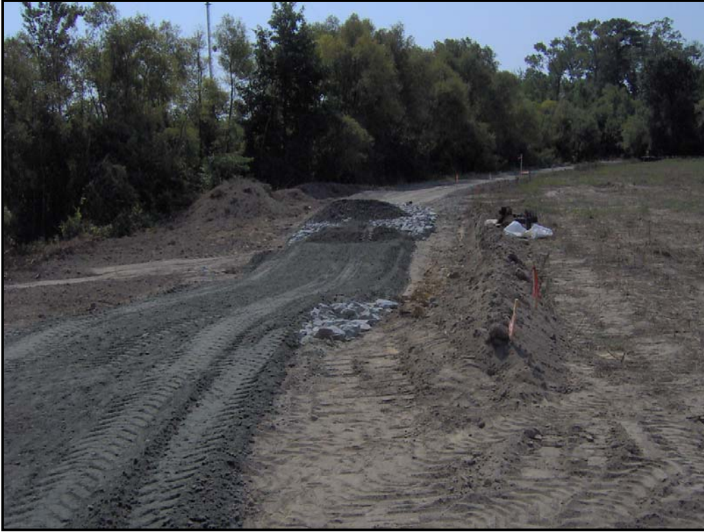
Road Crossing Type B – Station 30+50 – Immediately after completion
