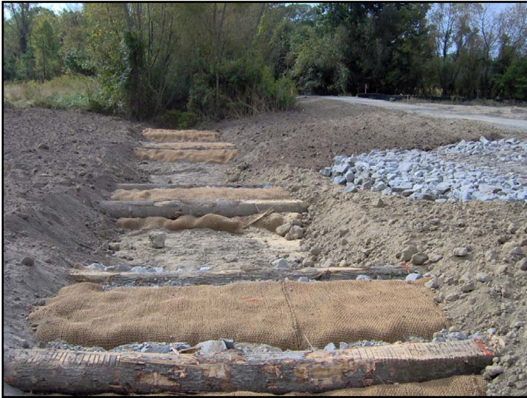
Grade Transition – Facing downstream
