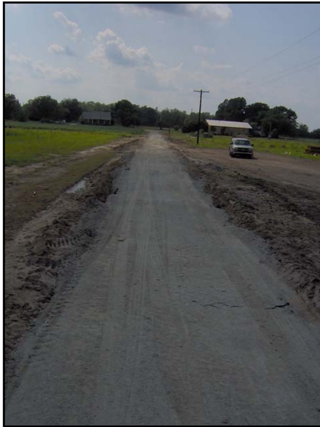
Second Road Crossing Type A – Station 17+75 – Facing east toward Macedonia Rd.
