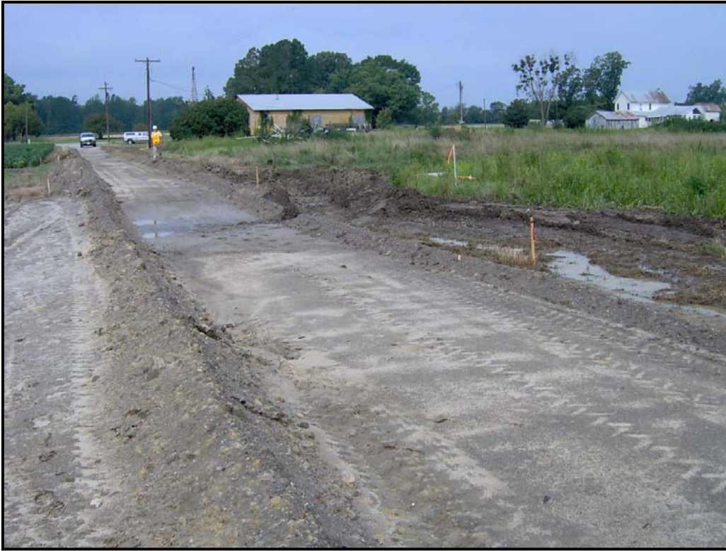
First Road Crossing Type A – Station 50+75 - Facing east toward Macedonia Rd.
