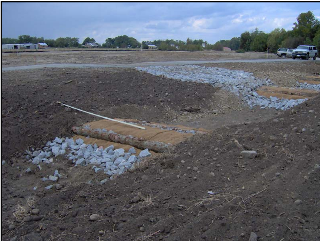
Road Crossing Type C – Station 32+50 – In background, immediately after completion
