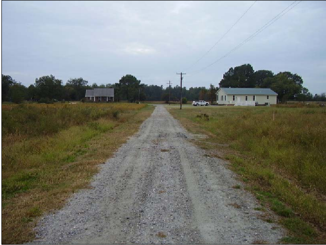
First Road Crossing Type A - Station 50+75 - Facing east toward Macedonia Road
