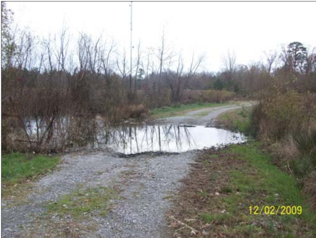
Photo Point 8 – 12/2/09 - MY 02 – Road Crossing Type B – Station 30+50
