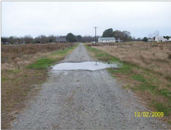
Photo Point 4 – 12/2/09 - MY 02 – Road Crossing Type A – Station 17+75 – Facing west toward Macedonia Road.
