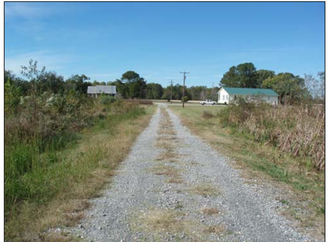
Photo Point 5 – 10/30/12 - MY 05 – Road Crossing Type A – Station 50+75 – Facing west toward Macedonia Road.
