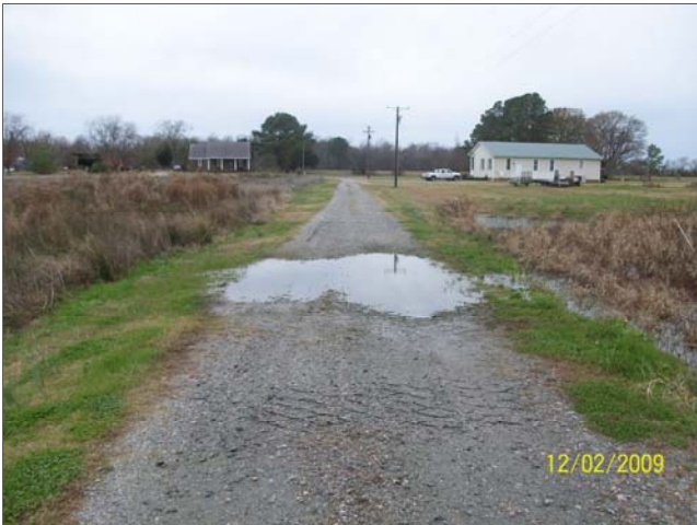
Photo Point 5 – 12/2/09 - MY 02 – Road Crossing Type A – Station 50+75 – Facing west toward Macedonia Road.
