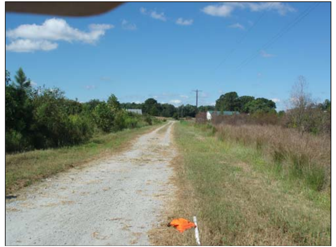
Photo Point 4 – 9/17/13 - MY 06 – Road Crossing Type A – Station 17+75 – Facing west toward Macedonia Road.
