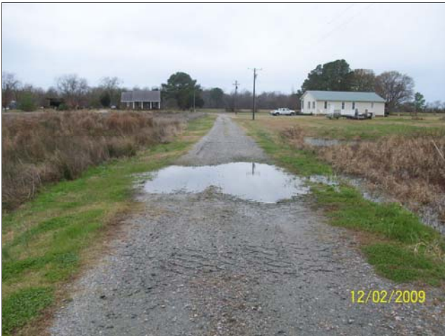
Photo Point 5 – 12/2/09 - MY 02 – Road Crossing Type A – Station 50+75 – Facing west toward Macedonia Road.
