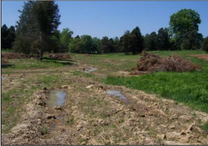
As-Built Surveys, April 2008
