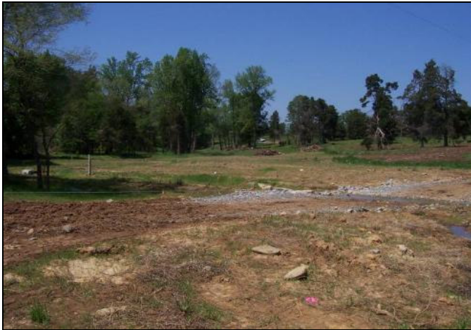
As-Built Surveys, April 2008
