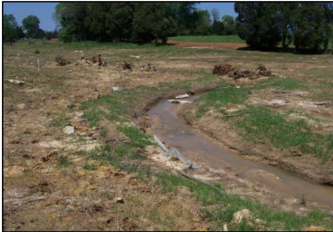
As-Built Surveys, April 2008
