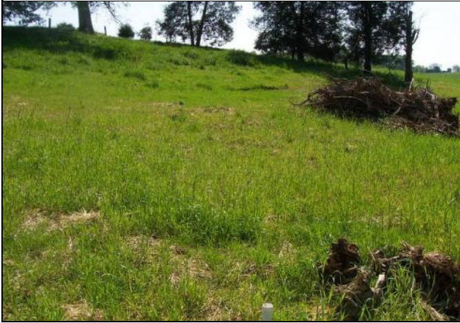
As-Built Surveys, April 2008
