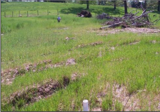
As-Built Surveys, April 2008
