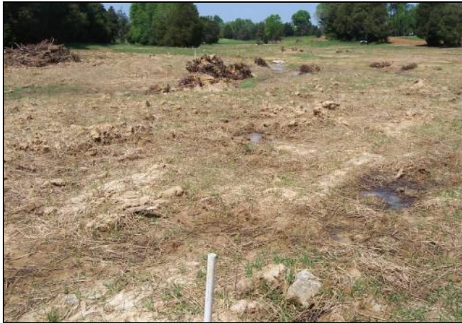
As-Built Surveys, April 2008
