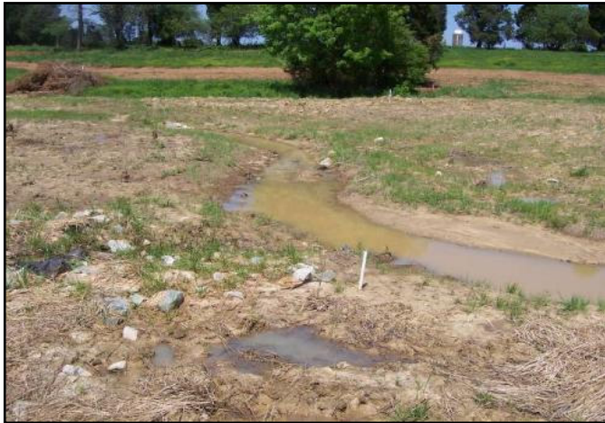
As-Built Surveys, April 2008
