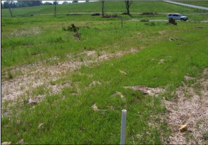
As-Built Surveys, April 2008
