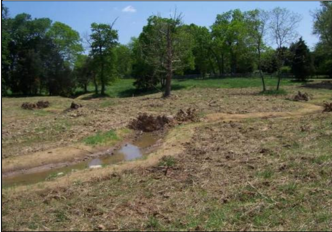
As-Built Surveys, April 2008
