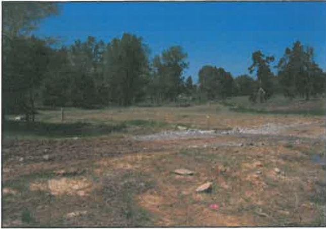
As-Built Surveys, April 2008
