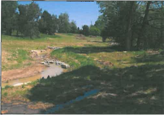
As-Built Surveys, April 2008
