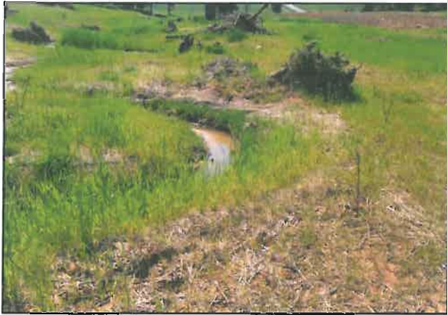
As-Built Surveys, April 2008
