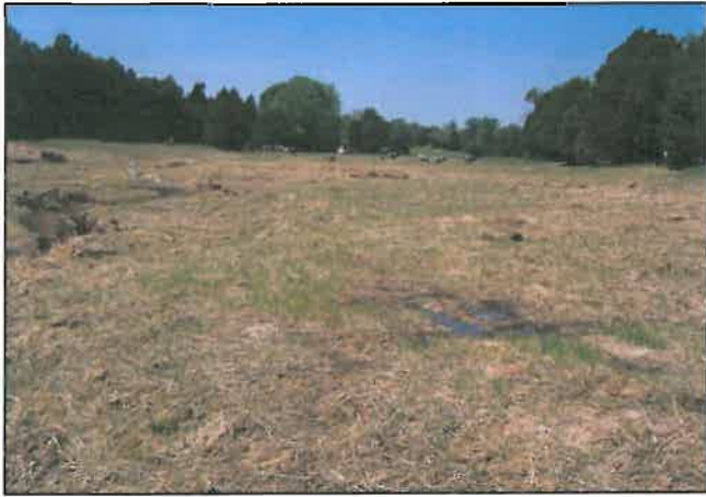
As-Built Surveys, April 2008
