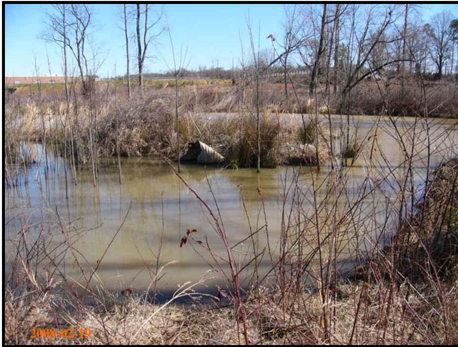
Sediment basin inline with UT Rocky River's channel. Also, beavers have built a large dam that can be seen on far right side of picture.
