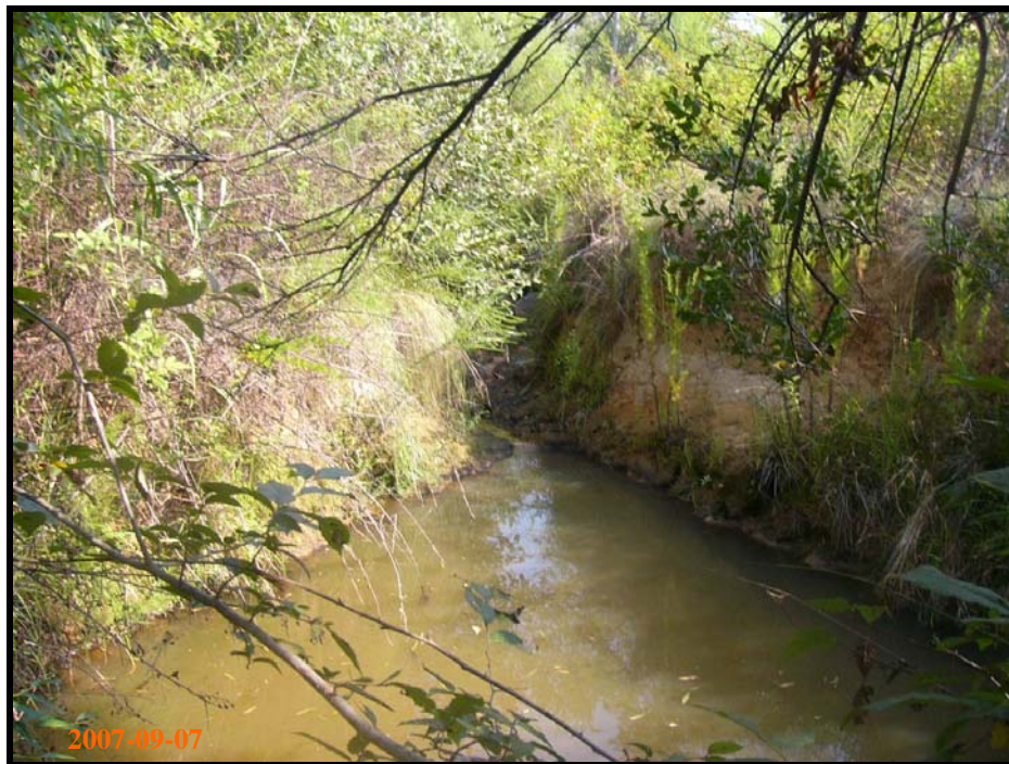
Mass wasting of channel banks through a gully reach.
