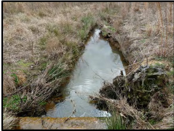
3.21 Eroded bank downstream of log sill near 20+90
