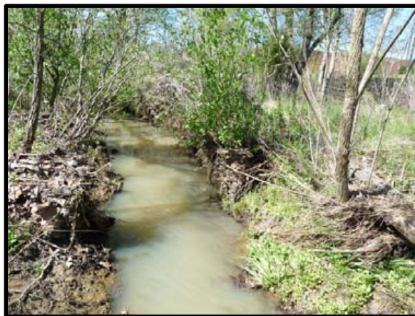
3.20 Minor erosion at 15+00
