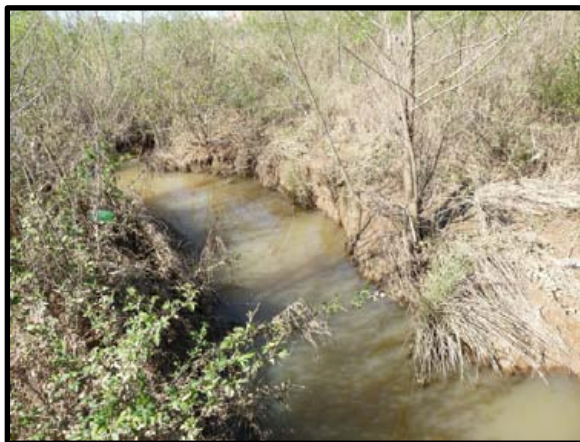
3.19 Moderate erosion above 35+00
