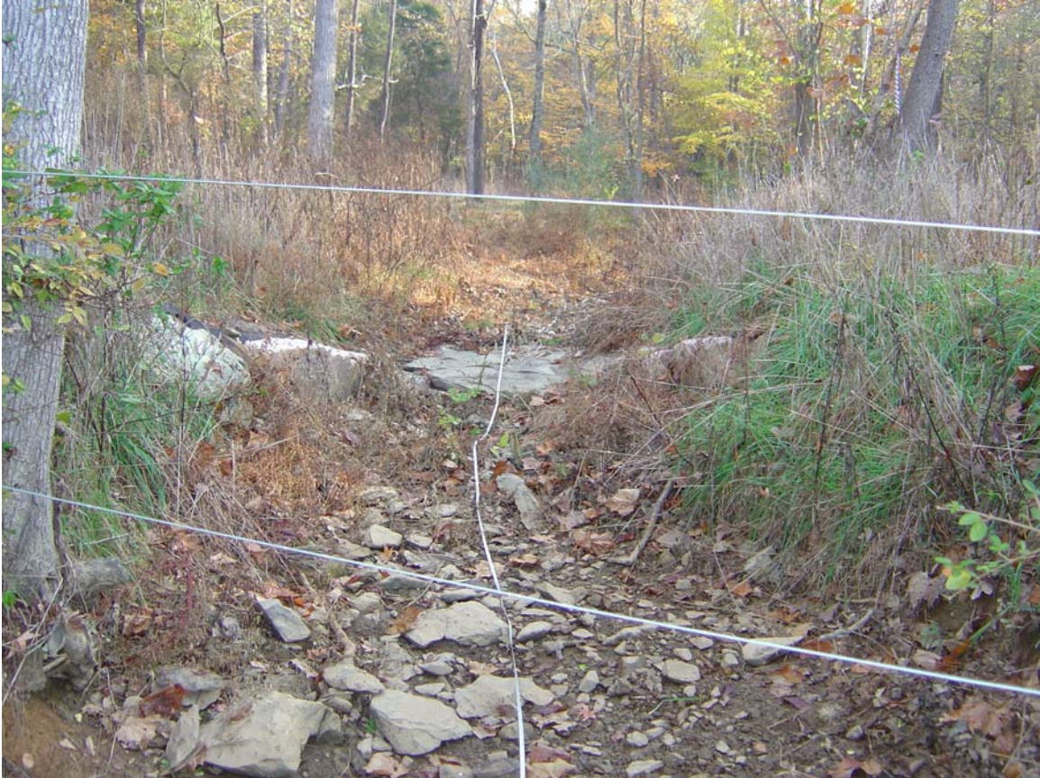
Photo 382 - looking upstream at cross vane Reach 1
