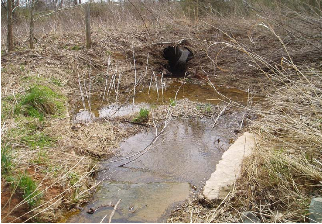
SP2. Aggradation/bar formation downstream of last cross vane at Station 1096. Looking upstream.
