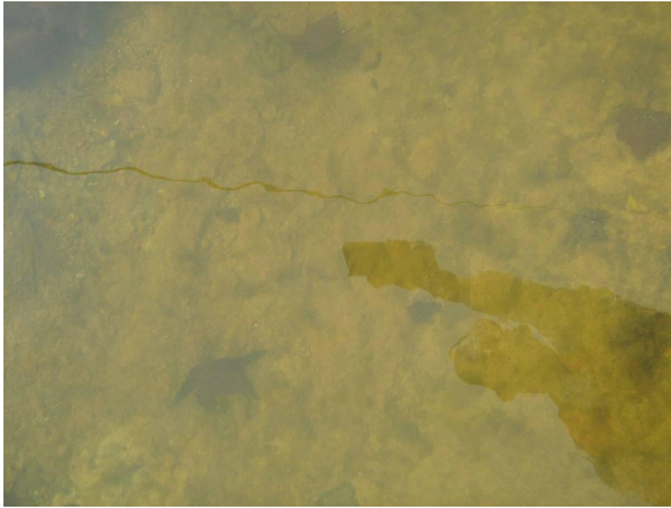
Photograph 52: Cross Section 2 looking at the substrate composition.
