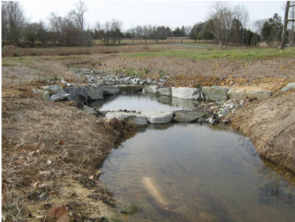
Photograph 30: "A" Vane. STA: 117+58.
