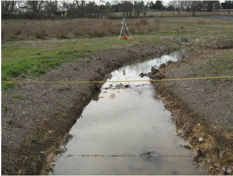
Photograph 53: Cross Section 3 looking upstream.
