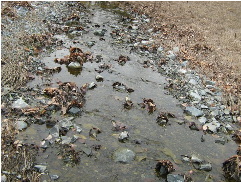
Photograph 4: Constructed Riffle. STA: 101+09.
