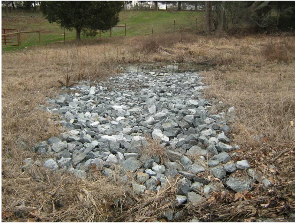
Photograph 9: Armored Outlet Swale from Wetland.
