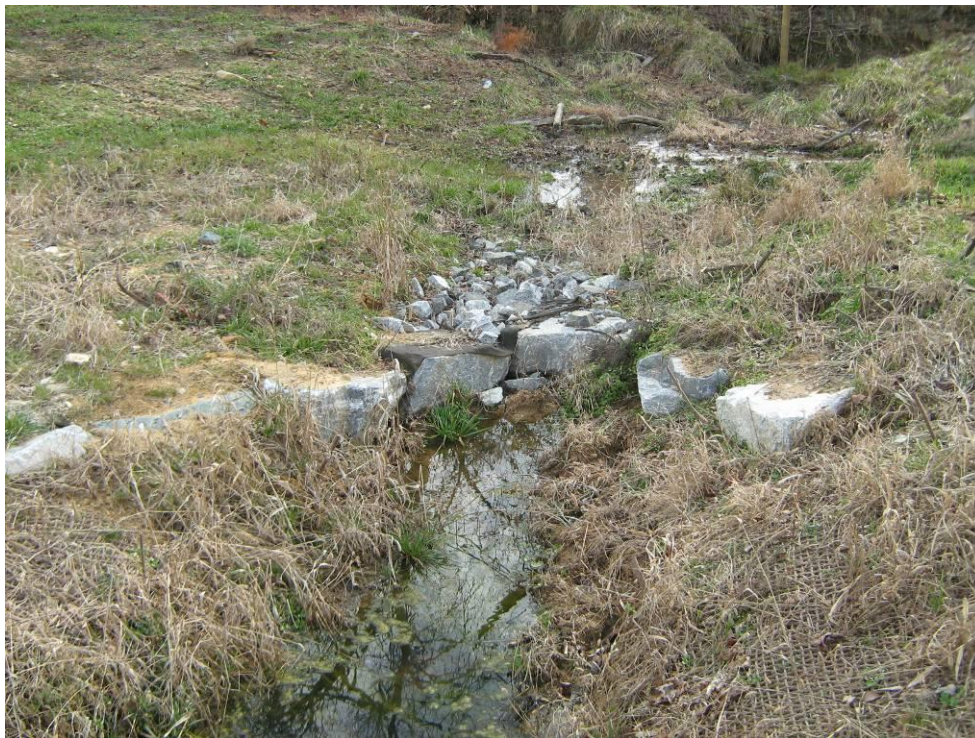
Photograph 38: Cross Vane. STA: 200+57.
