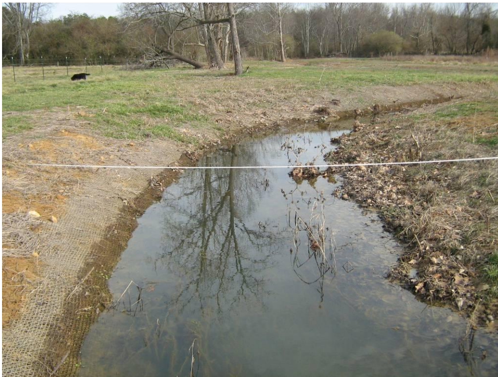
Photograph 59: Cross Section 4 looking downstream.
