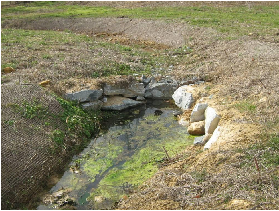
Photograph 39: Cross Vane. STA: 201+16.
