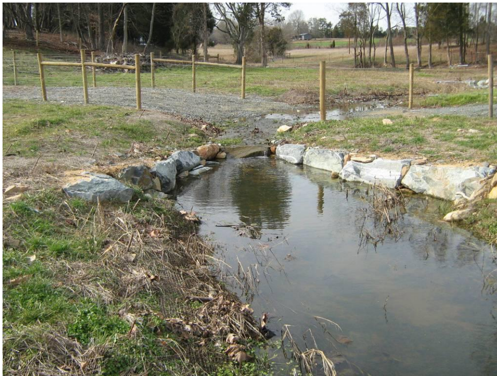
Photograph 24: Cross Vane. STA: 111+66.
