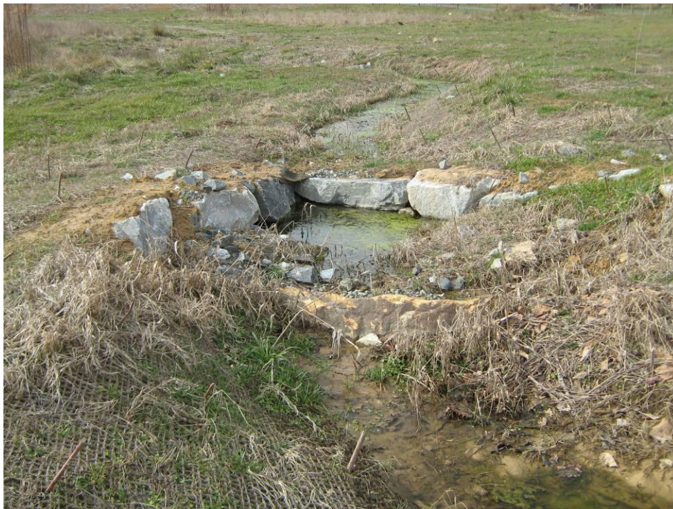
Photograph 42: Cross Vane. STA: 203+58.
