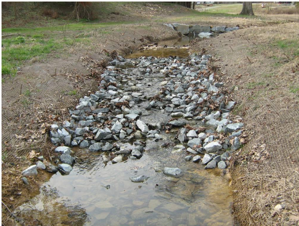
Photograph 20: Constructed Riffle. STA: 109+58.
