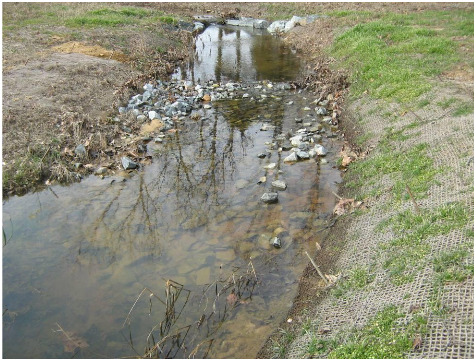
Photograph 22: Constructed Riffle. STA: 110+58.
