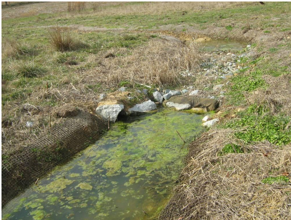
Photograph 40: Cross Vane. STA: 202+64.
