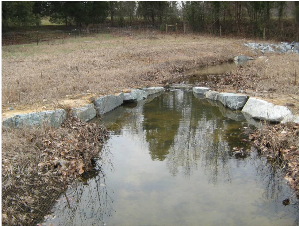
Photograph 3: Cross Vane. STA: 100+73.
