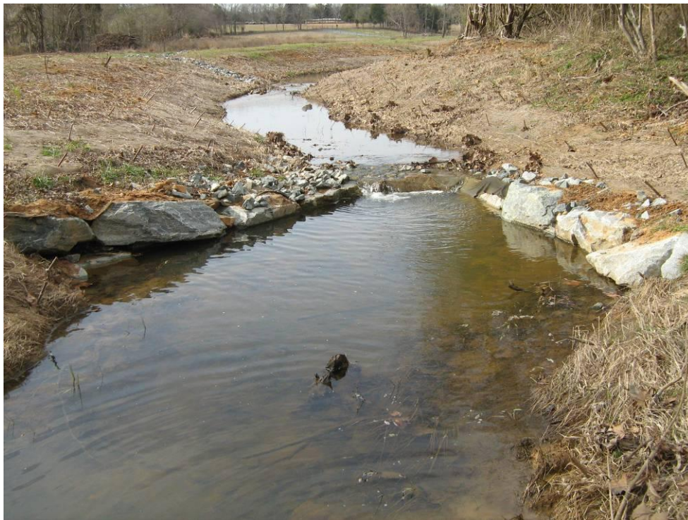
Photograph 36: Cross Vane. STA: 121+92
