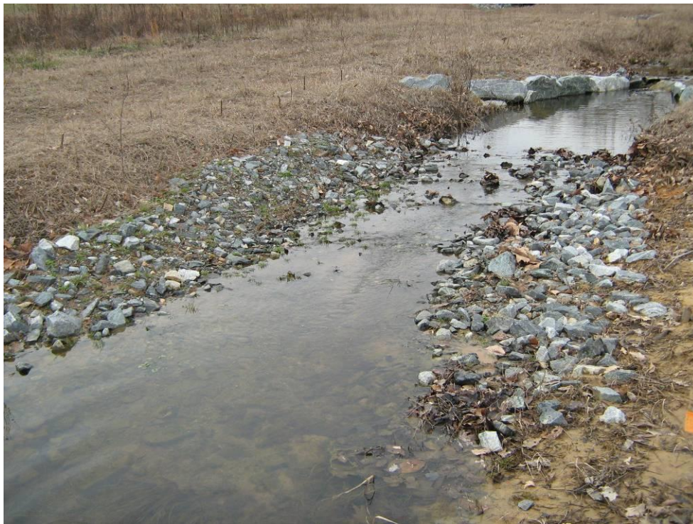
Photograph 8: Constructed Riffle. STA: 103+15.
