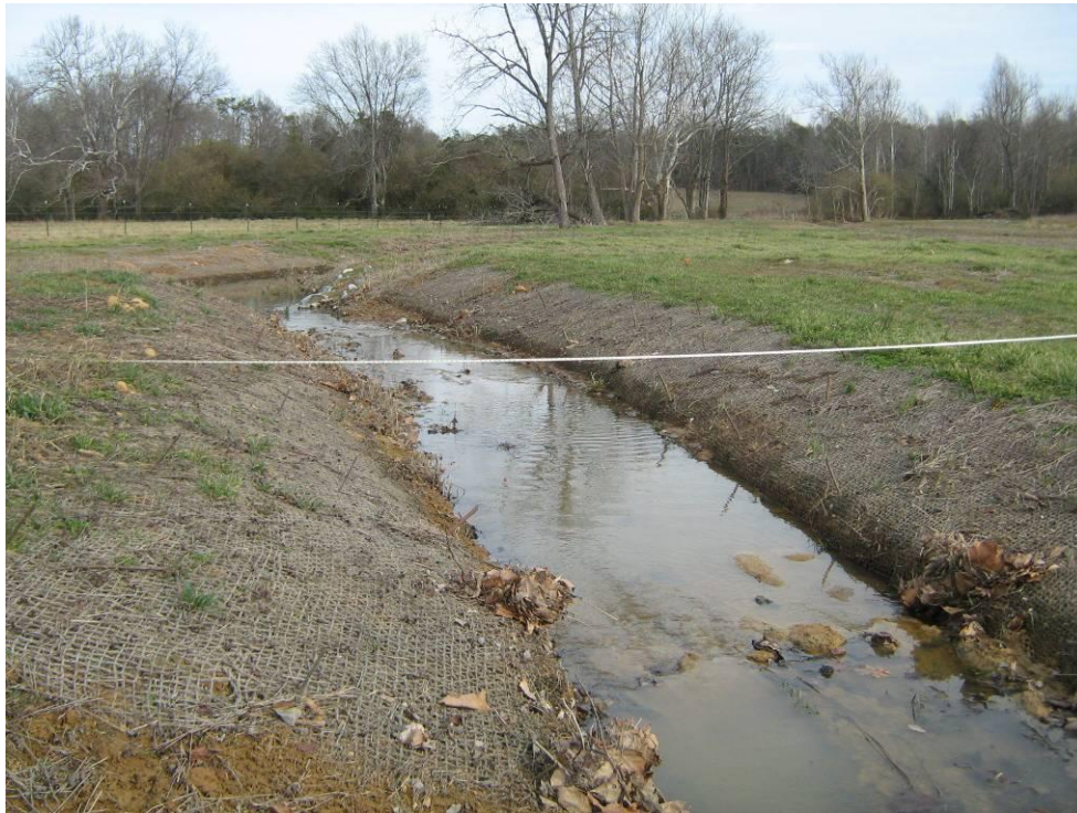
Photograph 54: Cross Section 3 looking downstream.
