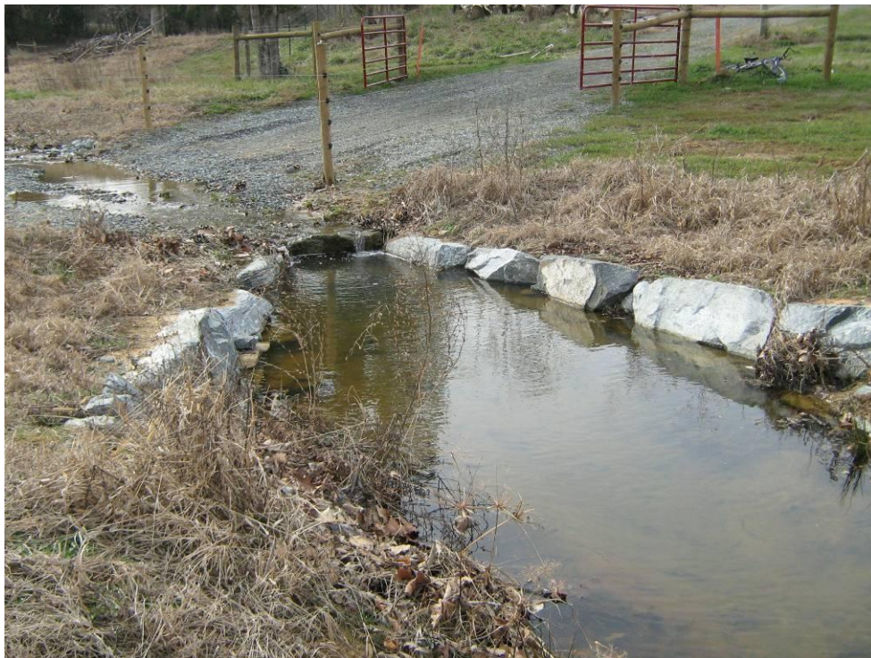
Photograph 12: Cross Vane. STA: 104+75.
