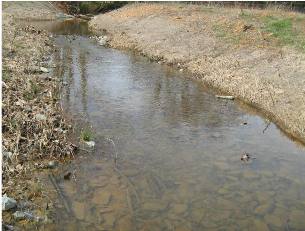
Photograph 33: Constructed Riffle. STA: 120+00
