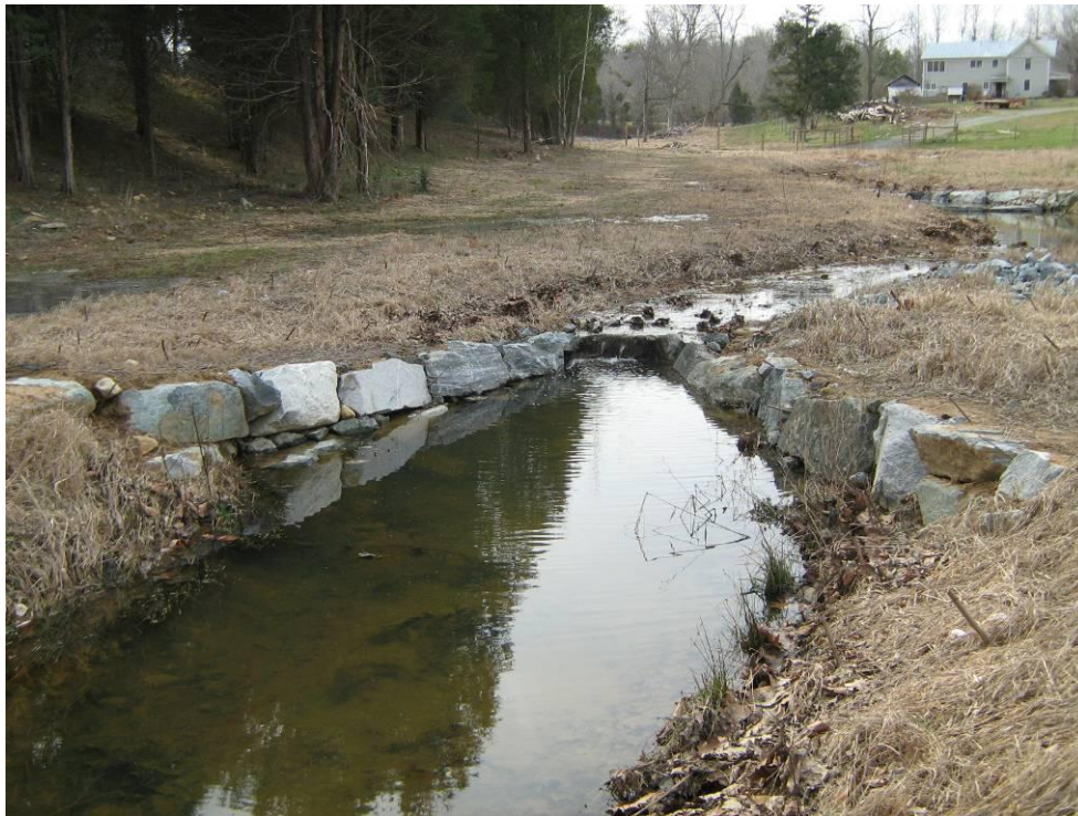
Photograph 16: Cross Vane. STA: 107+49.
