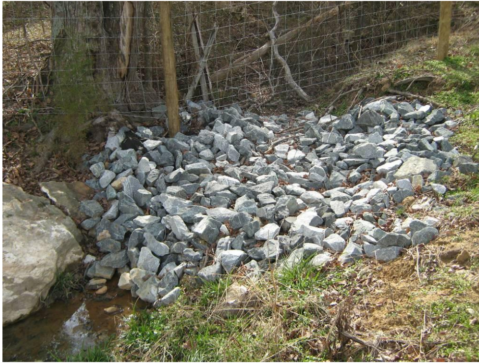
Photograph 37: Rip-Rap. Head of UT-2.
