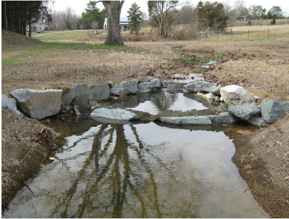
Photograph 19: "A" Vane. STA: 109+14.
