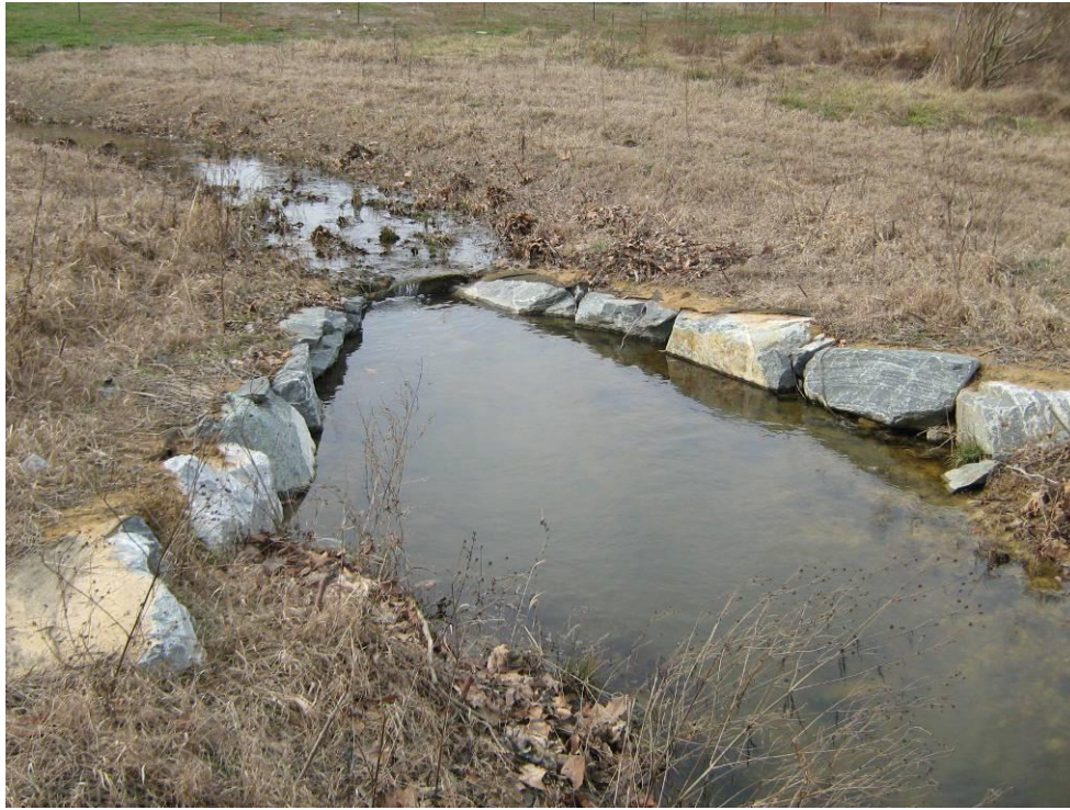
Photograph 13: Cross Vane. STA: 105+62.
