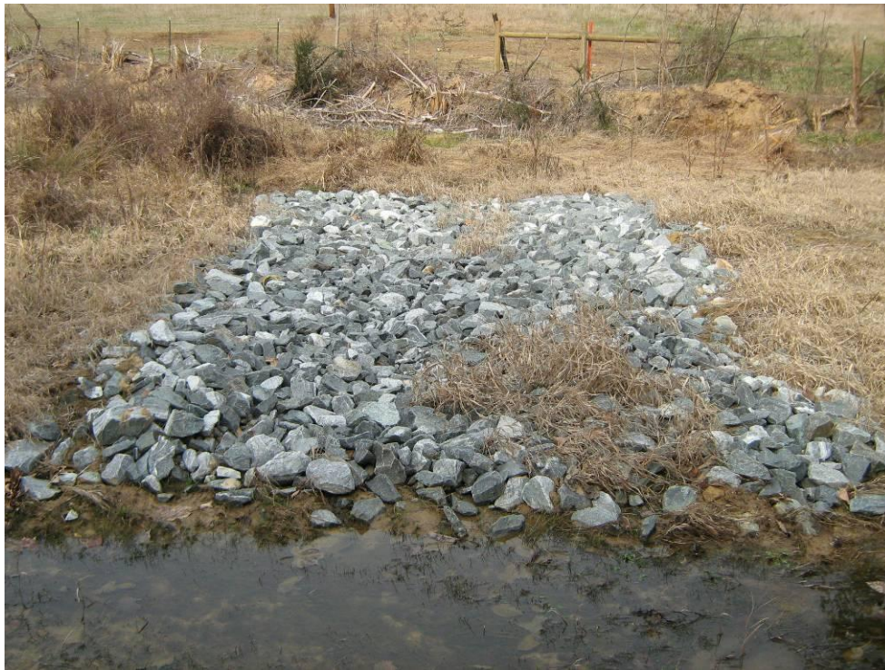
Photograph 15: Armored Swale Entering Channel.
