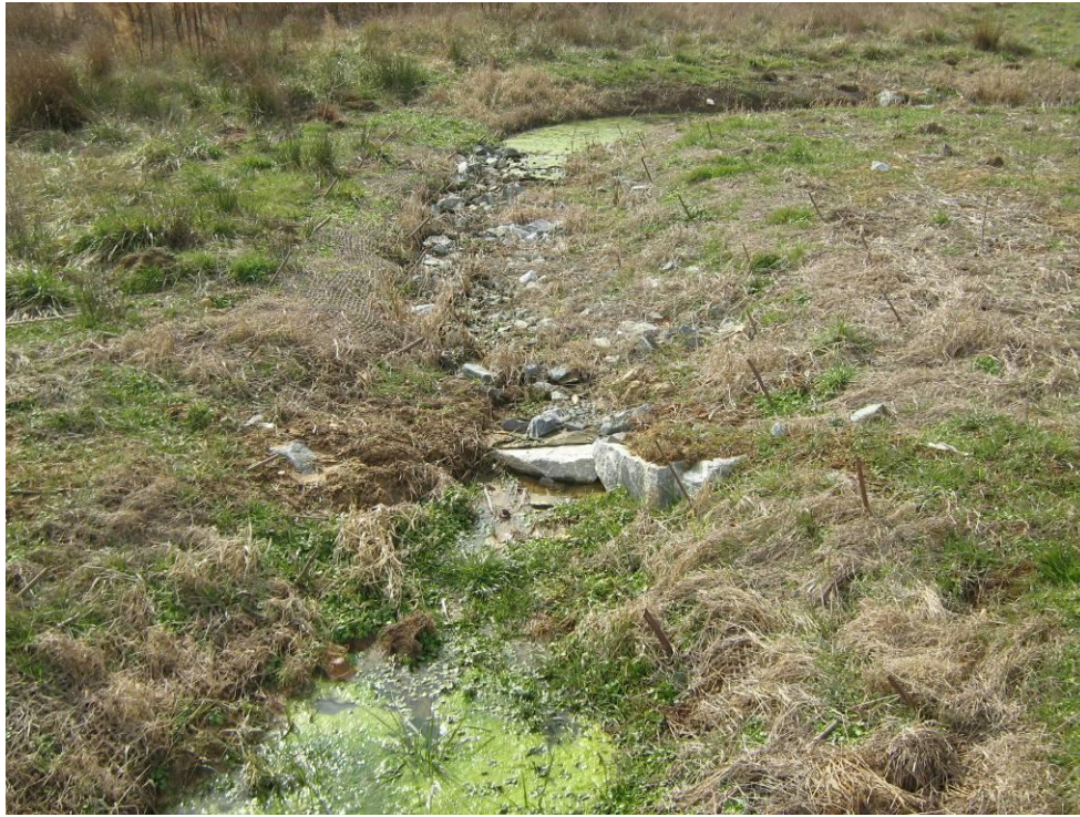
Photograph 41: Cross Vane. STA: 203+15.
