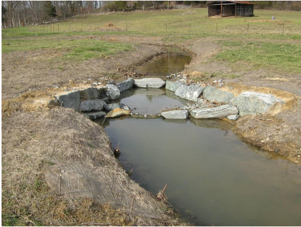
Photograph 29: "A" Vane. STA: 116+29.
