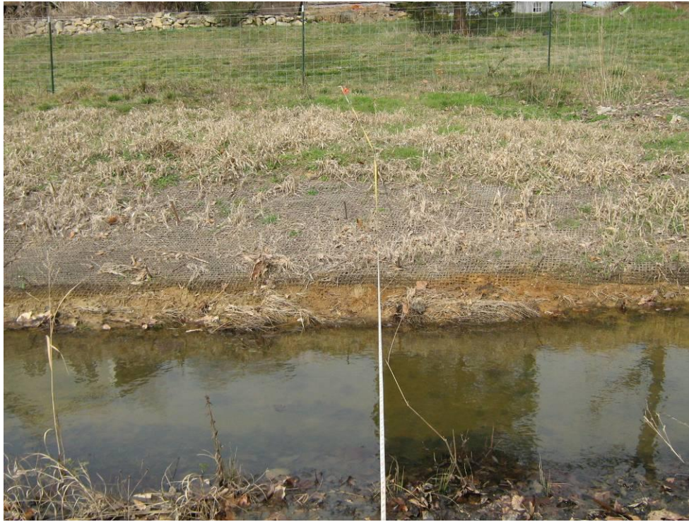
Photograph 50: Cross Section 2 looking at the left bank.
