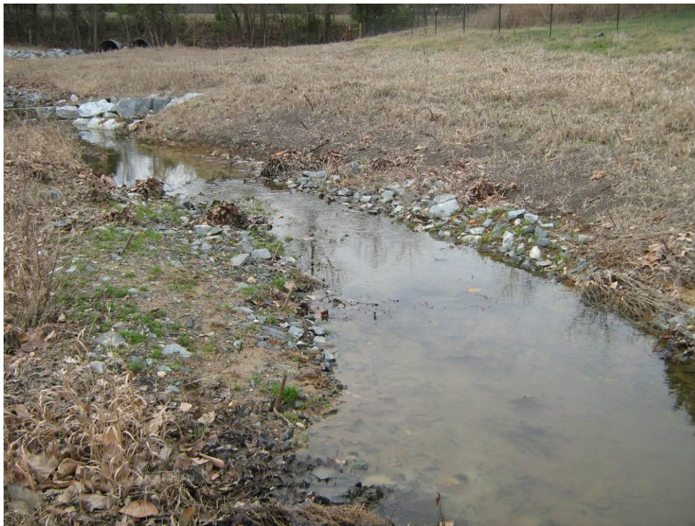
Photograph 6: Constructed Riffle. STA: 102+25.
