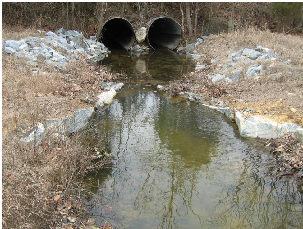
Photograph 2: Cross Vane. STA: 100+12.
