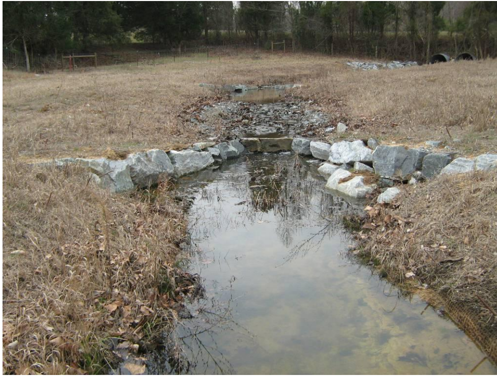
Photograph 5: Cross vane. STA: 101+40.
