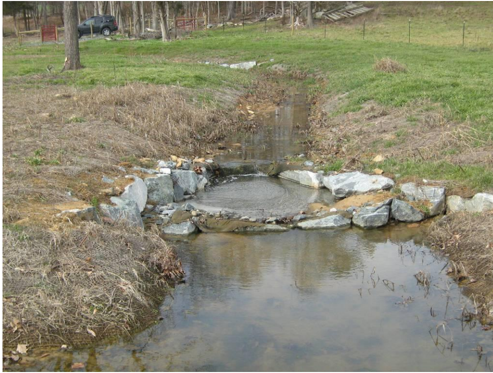
Photograph 27: "A" Vane. STA: 113+80.
