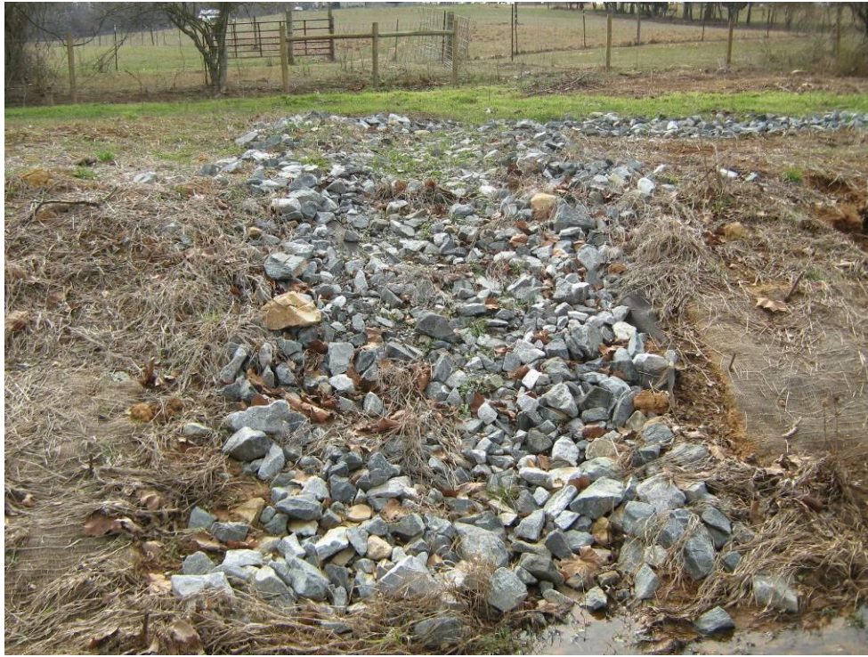
Photograph 35: Rip-Rap. Wetland drainage.
