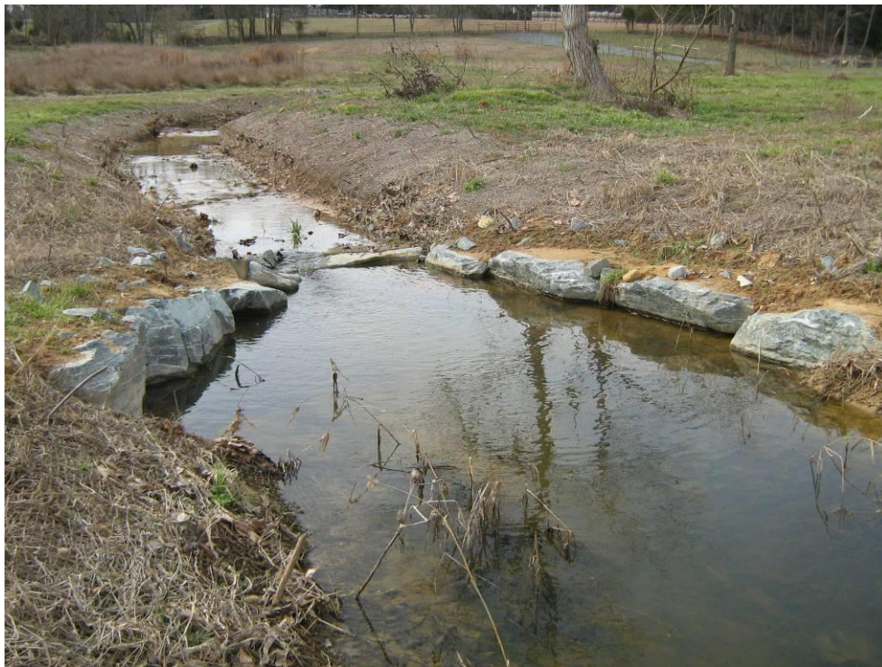
Photograph 28: Cross Vane. STA: 115+15.
