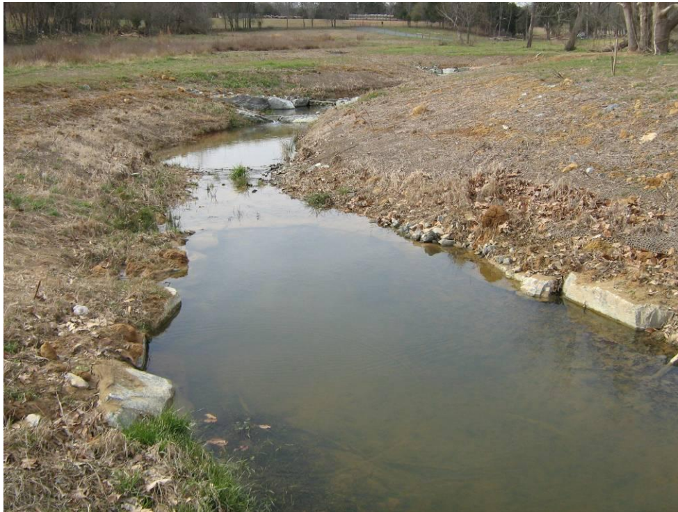
Photograph 32: Cross Vane. STA: 119+07.
