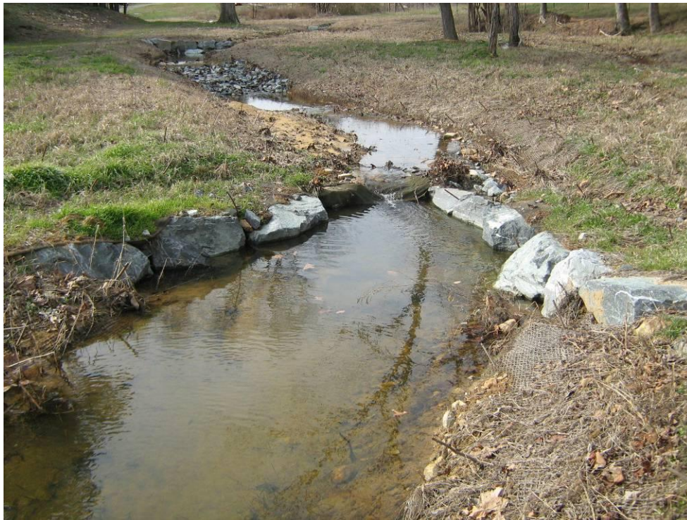
Photograph 21: Cross Vane. STA: 110+26.
