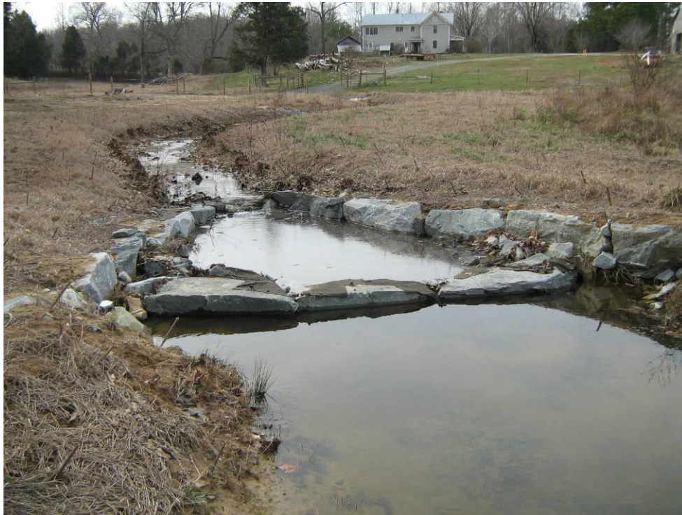
Photograph 14: "A" Vane. STA: 106+60.
