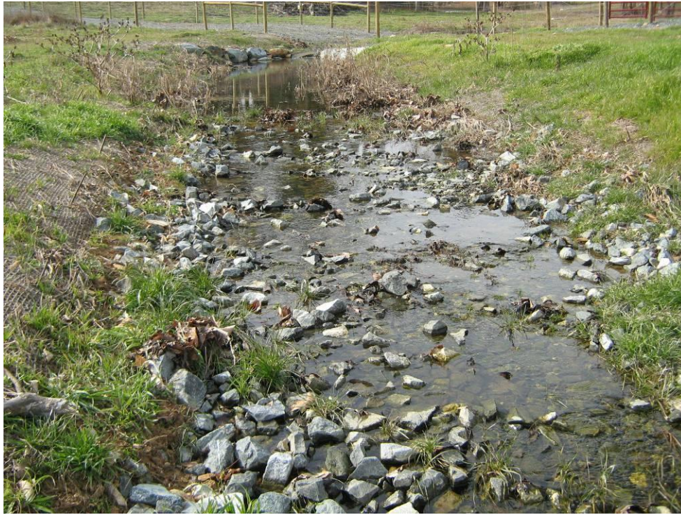
Photograph 25: Constructed Riffle. STA: 112+15.
