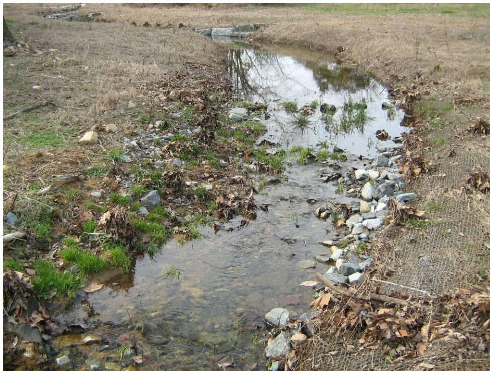
Photograph 18: Constructed Riffle. STA: 108+77.
