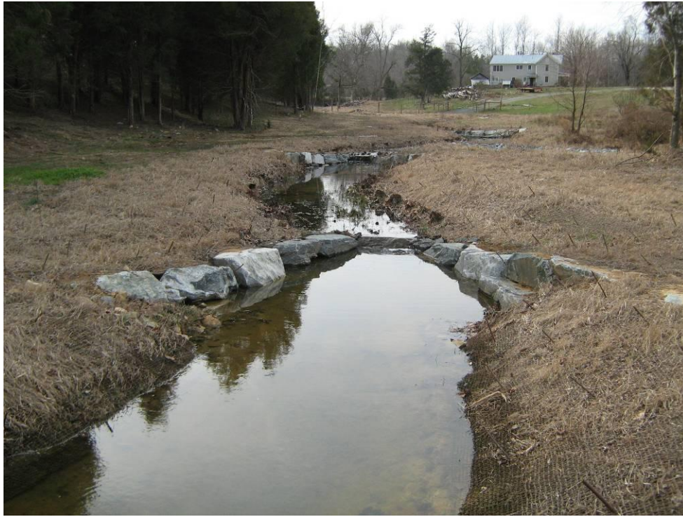
Photograph 17: Cross Vane. STA: 108+11.
