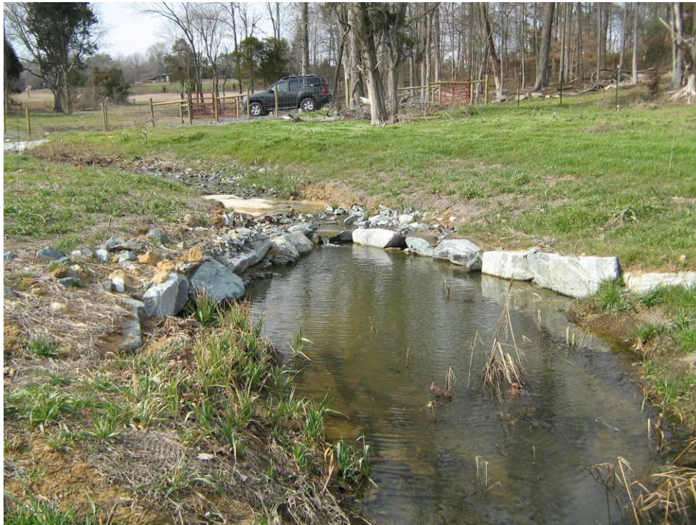
Photograph 26: Cross Vane. STA: 112+70.
