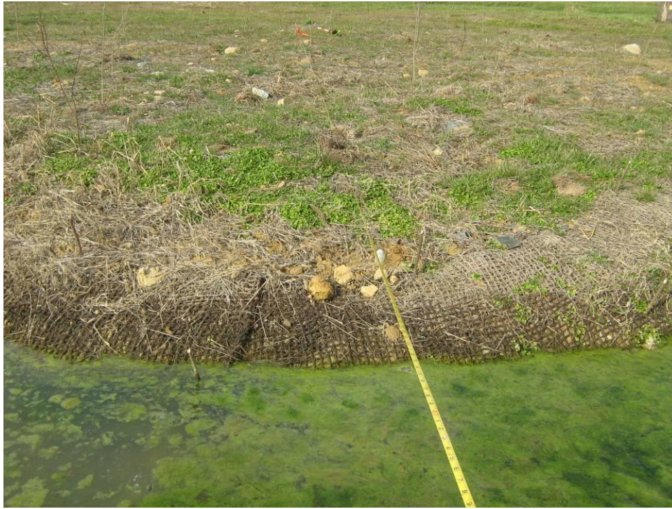
Photograph 70: Cross Section 6 looking at the left bank.
