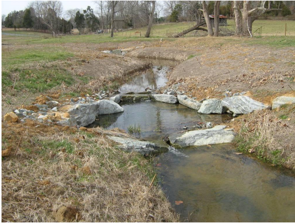
Photograph 31: “A” Vane. STA: 118+46.
