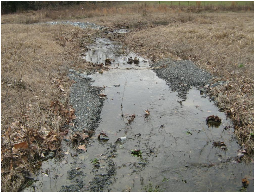
Photograph 10: Constructed Riffle. STA: 103+88.
