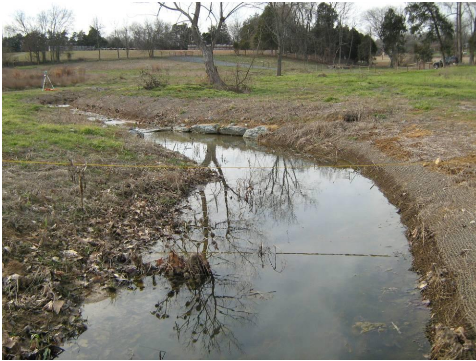
Photograph 58: Cross Section 4 looking upstream.
