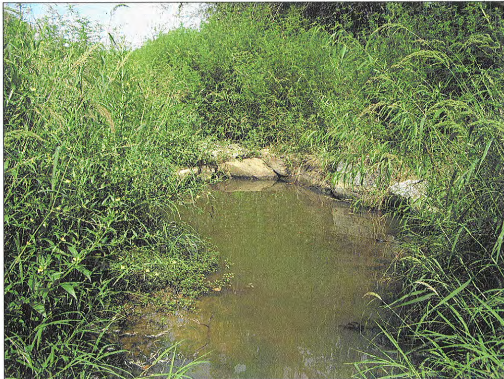
PHOTOGRAPH 36: CROSS VANE. STA: 122+00.
