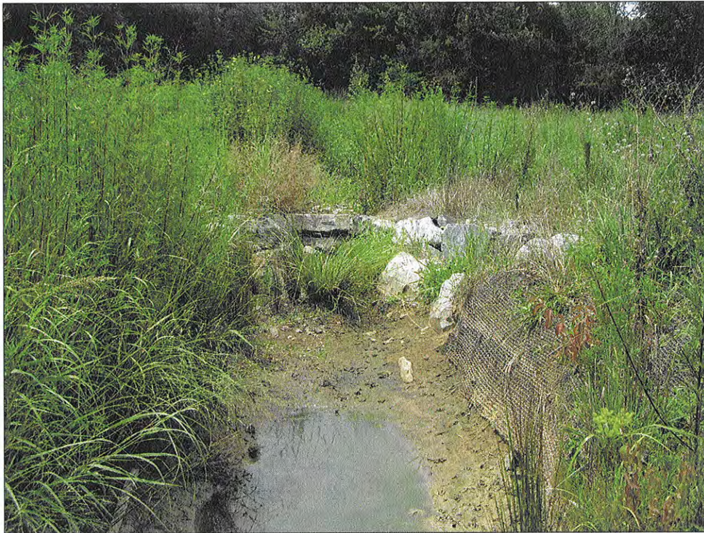
PHOTOGRAPH 5: CROSS VANE. STA: 101+40.
