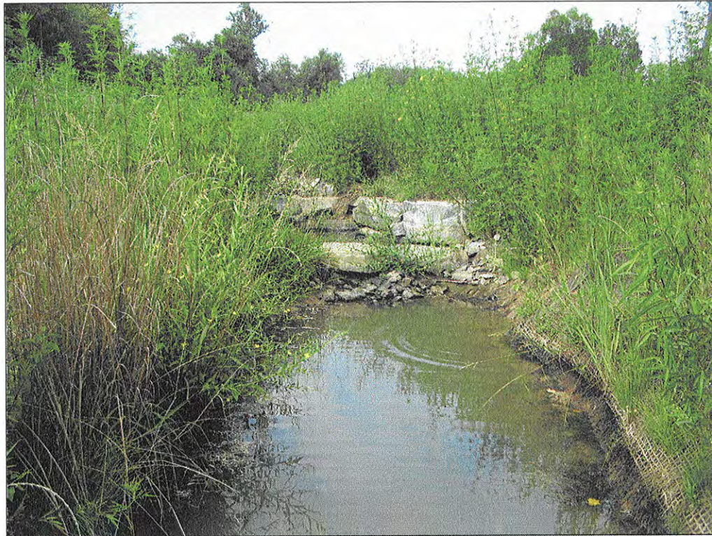
PHOTOGRAPH 30: "A" VANE. STA: 117+58.
