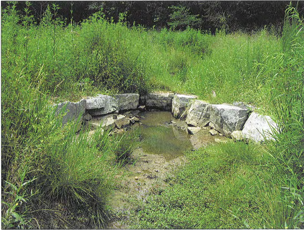
PHOTOGRAPH 3: CROSS VANE. STA: 100+73.
