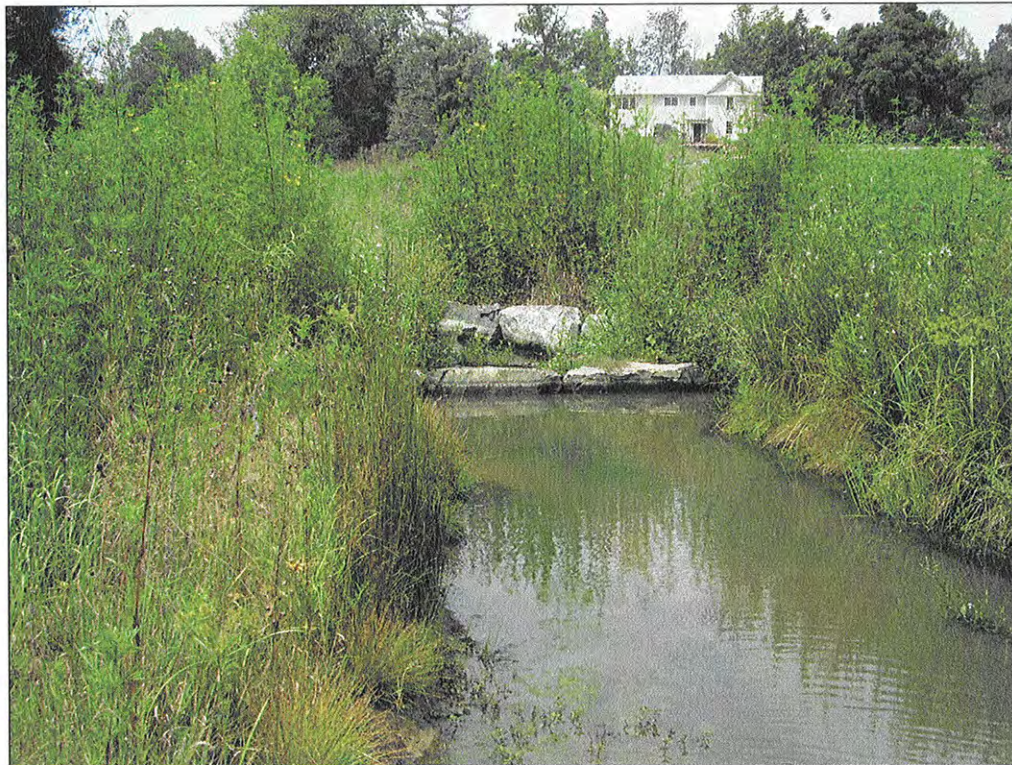
PHOTOGRAPH 14: "A" VANE. STA: 106+60.
