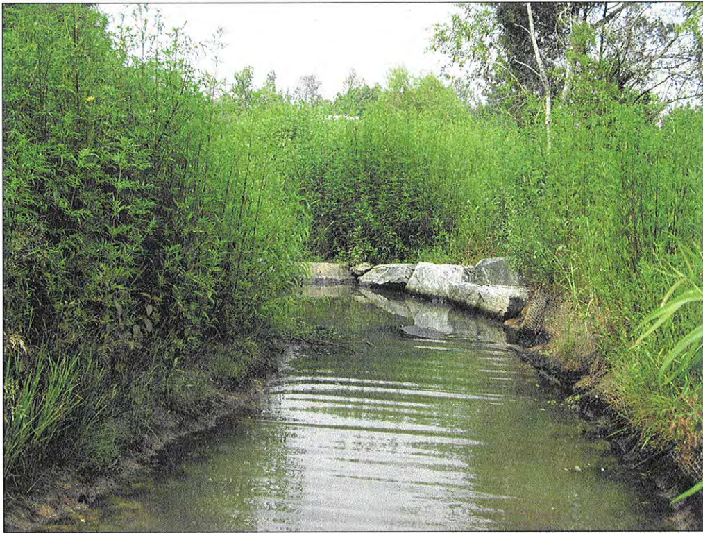
PHOTOGRAPH 17: CROSS VANE. STA: 108+11.
