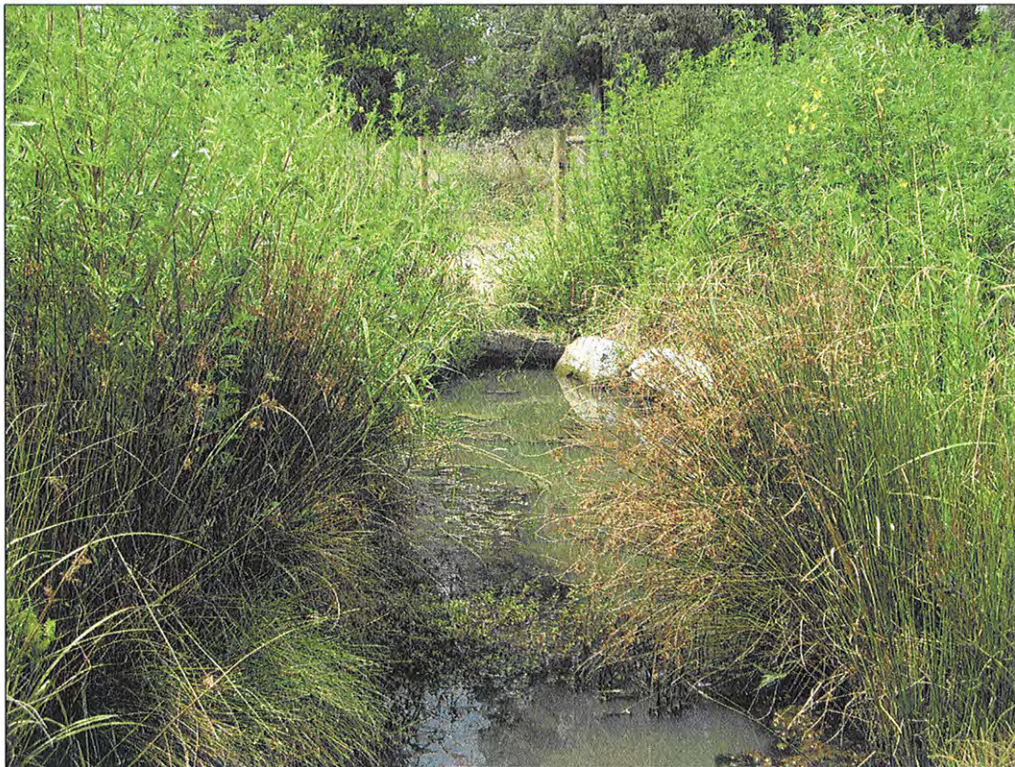
PHOTOGRAPH I2: CROSS VANE. STA: 104+75.
