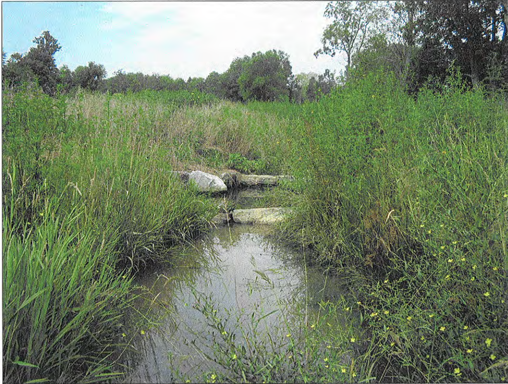
PHOTOGRAPH 31: "A" VANE. STA: 118+46.
