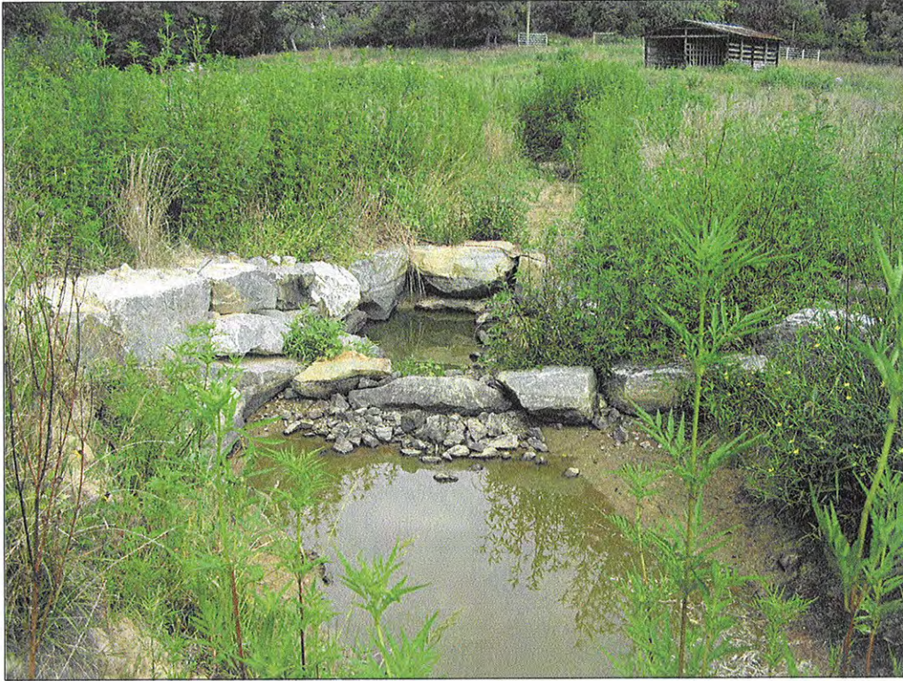
PHOTOGRAPH 29: "A" VANE. STA: 116+29.
