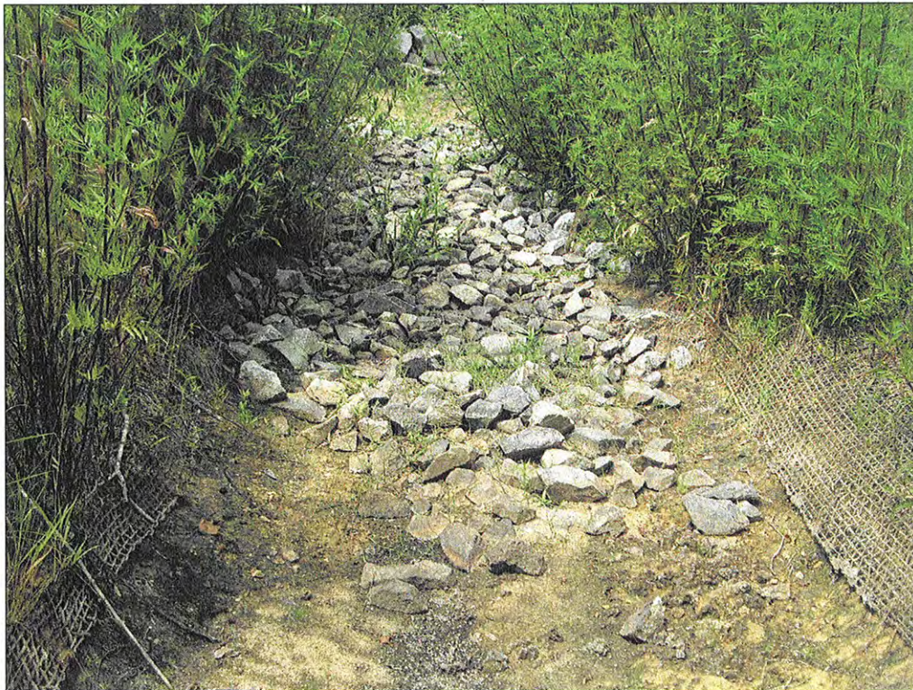
PHOTOGRAPH 20: CONSTRUCTED RIFFLE. STA: 109+58.
