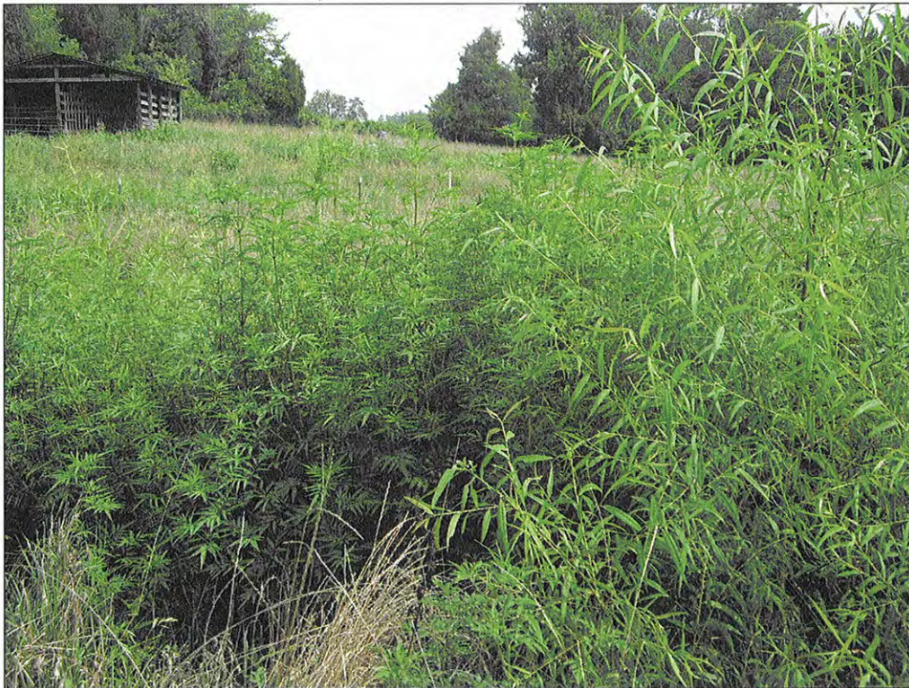
PHOTOGRAPH 60: CROSS SECTION 4 LOOKING AT THE LEFT BANK.
