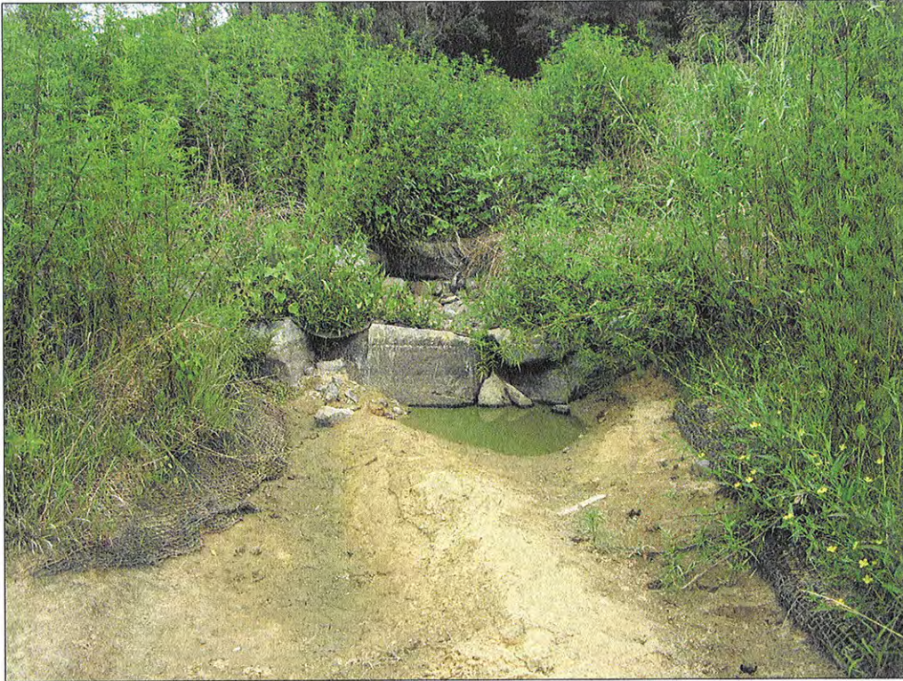
PHOTOGRAPH 27: "A" VANE. STA: 113+80.
