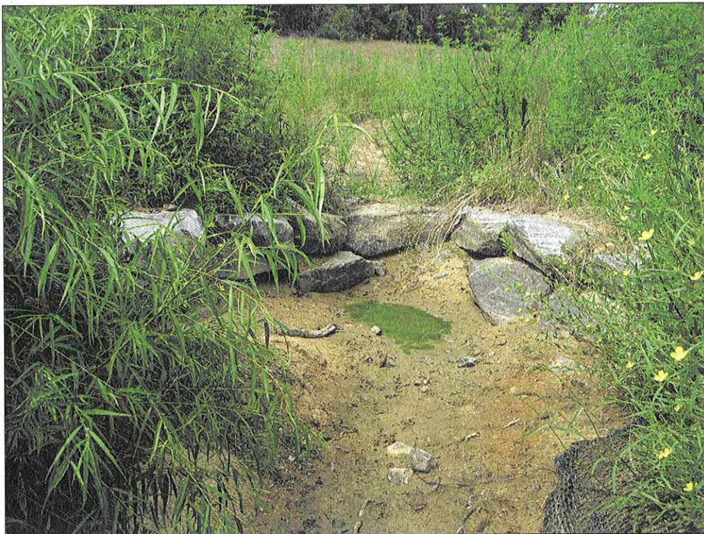
PHOTOGRAPH 28: CROSS VANE. STA: 115+15.
