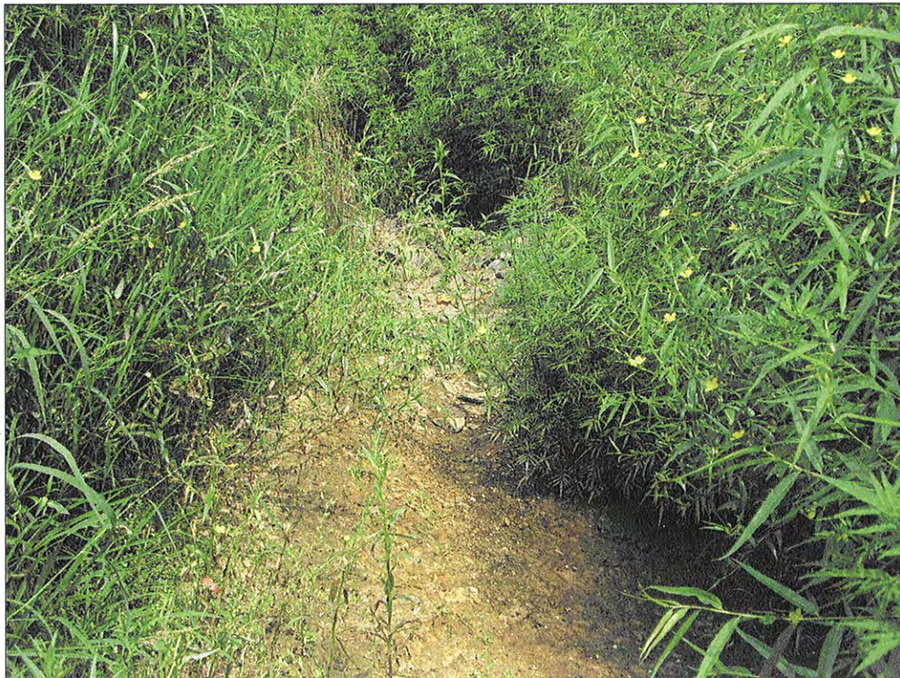
PHOTOGRAPH 22: CONSTRUCTED RIFFLE. STA: 110+58.
