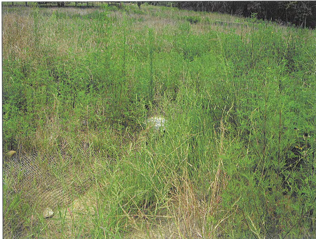
PHOTOGRAPH 40: CROSS VANE. STA: 202+64.
