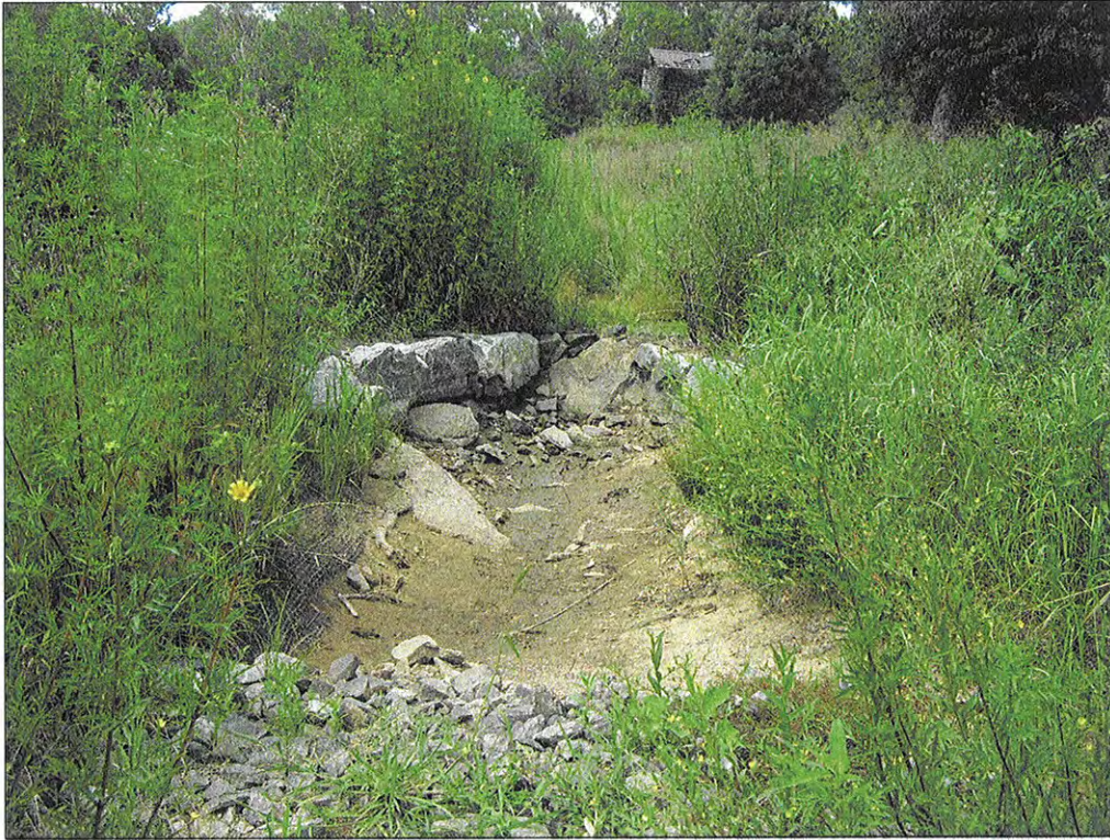
PHOTOGRAPH 7: CROSS VANE. STA: 102+85.
