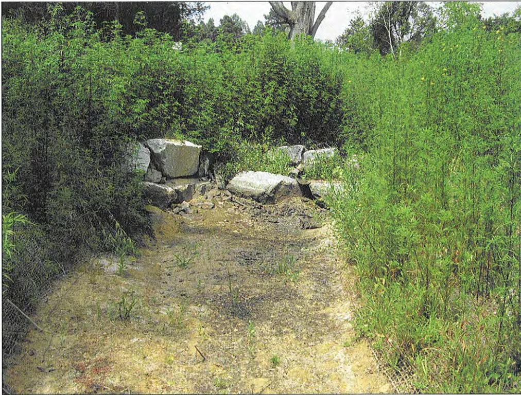
PHOTOGRAPH 19: "A" VANE. STA: 109+14.
