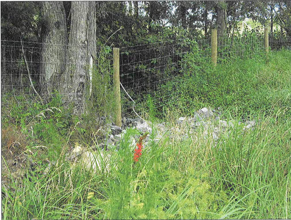
PHOTOGRAPH 37: RIP-RAP. HEAD OF UT-2.
