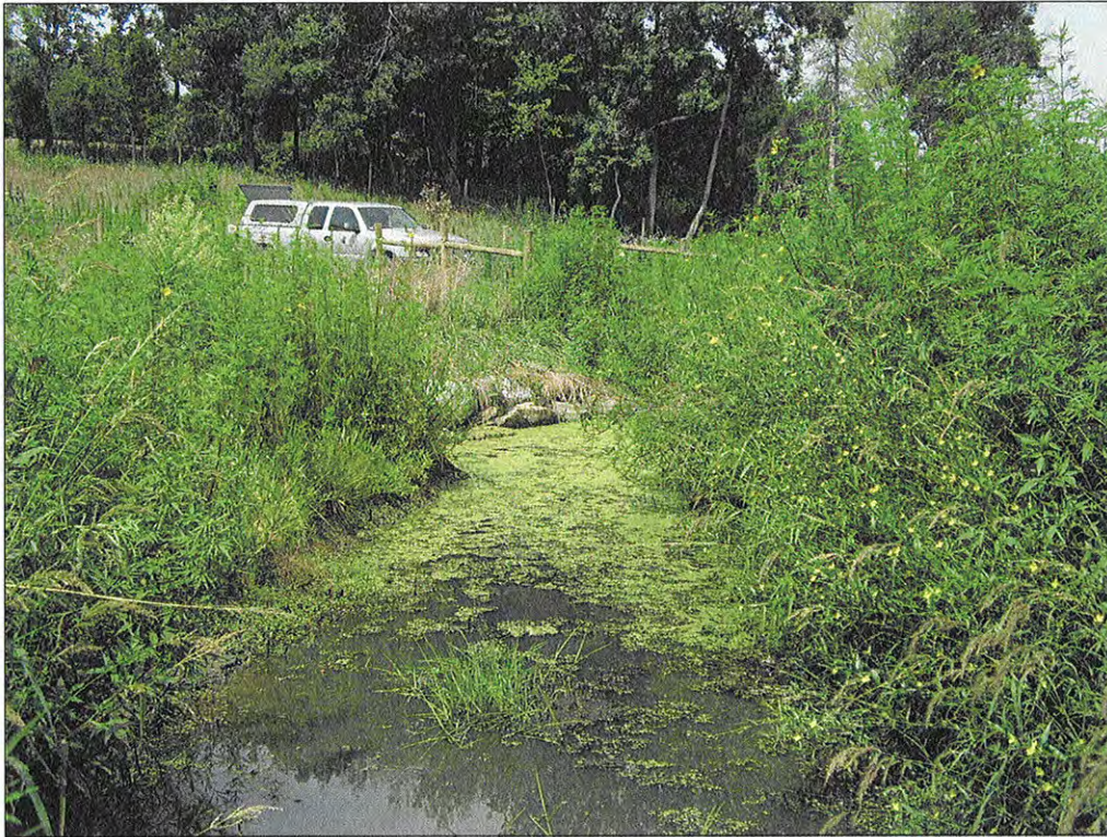
PHOTOGRAPH 25: CONSTRUCTED RIFFLE. STA: 112+15.
