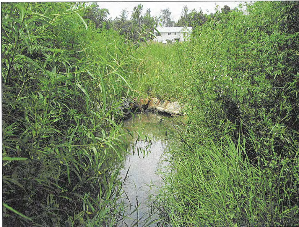
PHOTOGRAPH 16: CROSS VANE. STA: 107+49.
