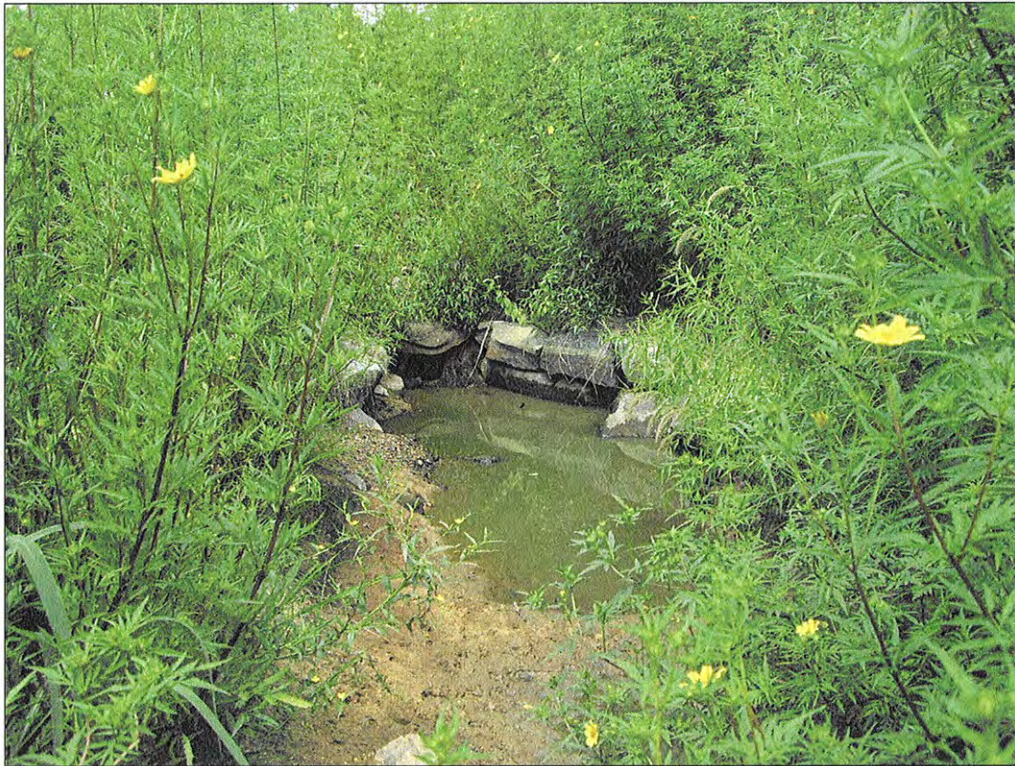
PHOTOGRAPH 21: CROSS VANE. STA: 110+26.
