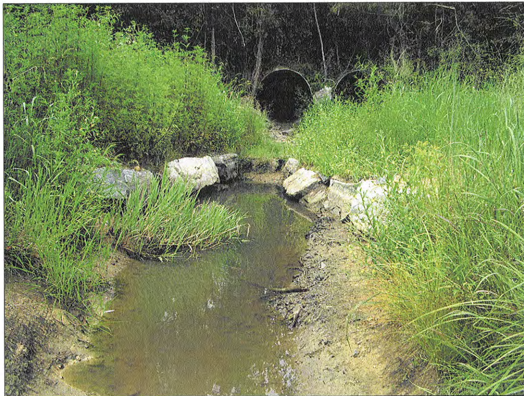
PHOTOGRAPH 2: CROSS VANE. STA: 100+12.
