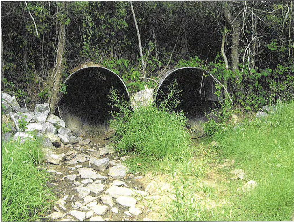
PHOTOGRAPH 1: RIP-RAP. HEAD OF UT-I.
