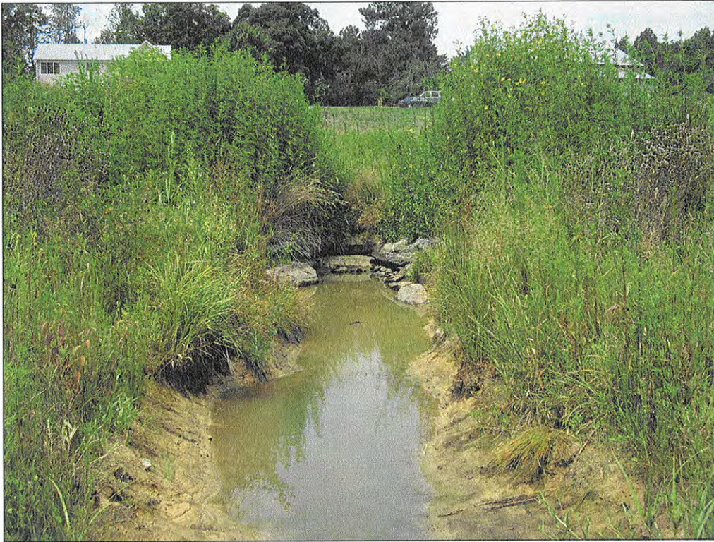
PHOTOGRAPH 13: CROSS VANE. STA: 105+62.
