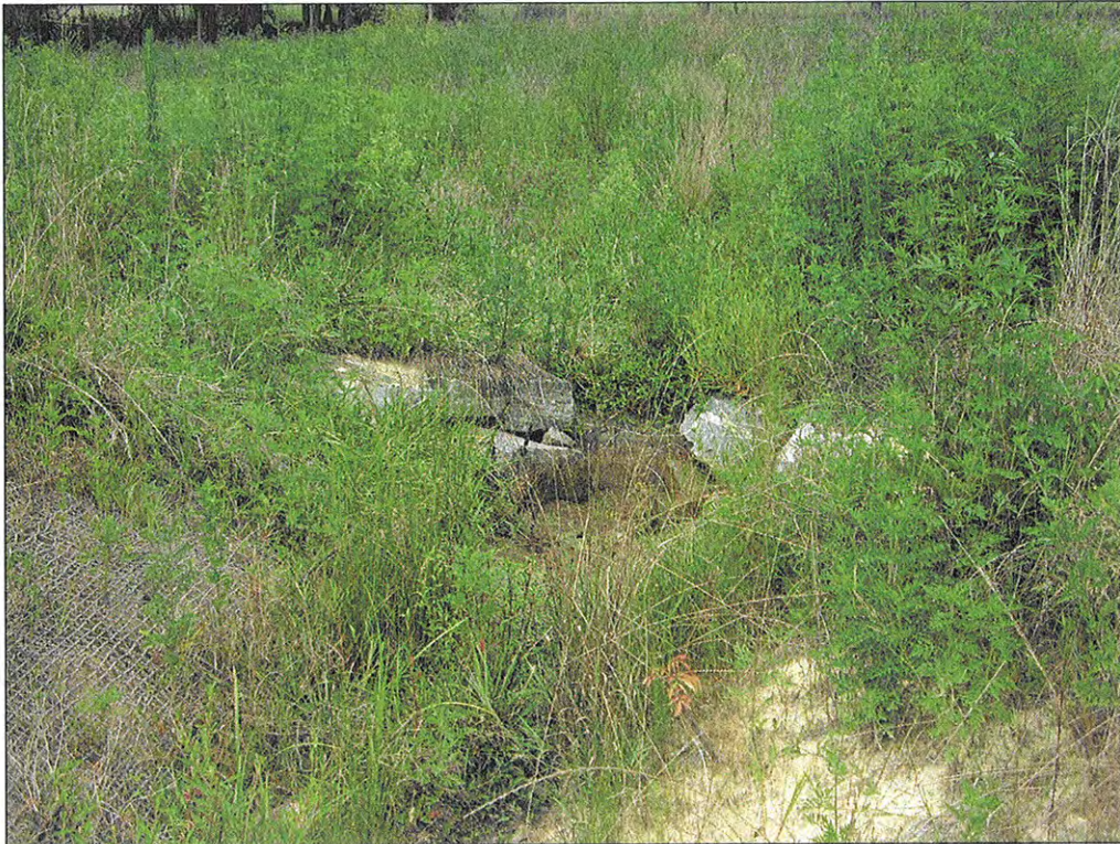
PHOTOGRAPH 39: CROSS VANE. STA: 201+16.
