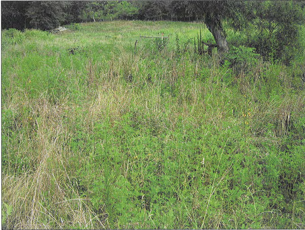
PHOTOGRAPH 55: CROSS SECTION 3 LOOKING AT THE BANK.
