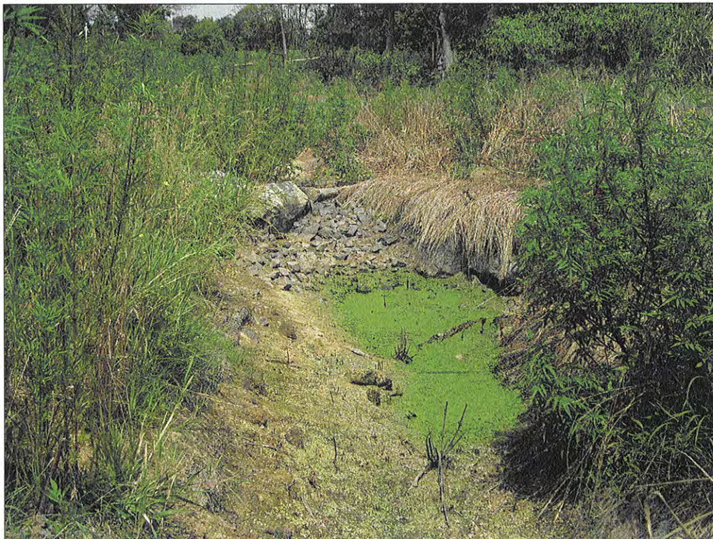
PHOTOGRAPH 26: CROSS VANE. STA: 112+70.
