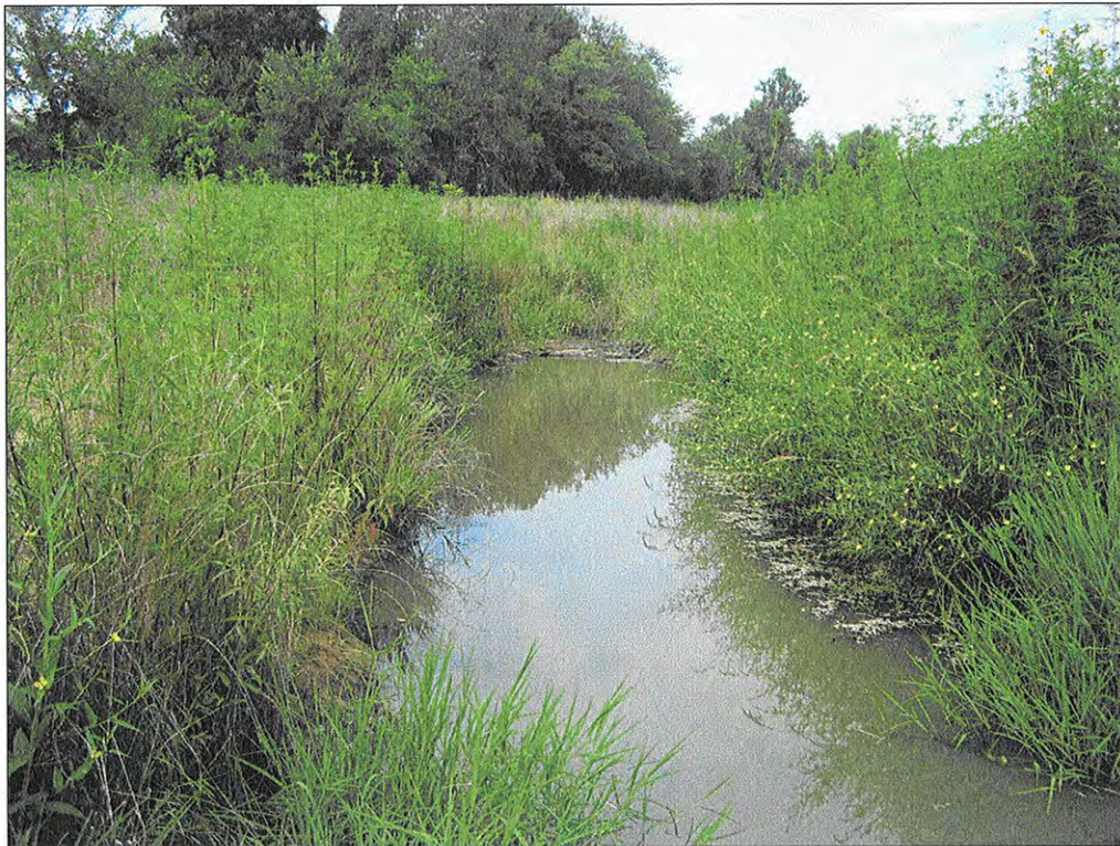
PHOTOGRAPH 32: CROSS VANE. STA: 119+07.
