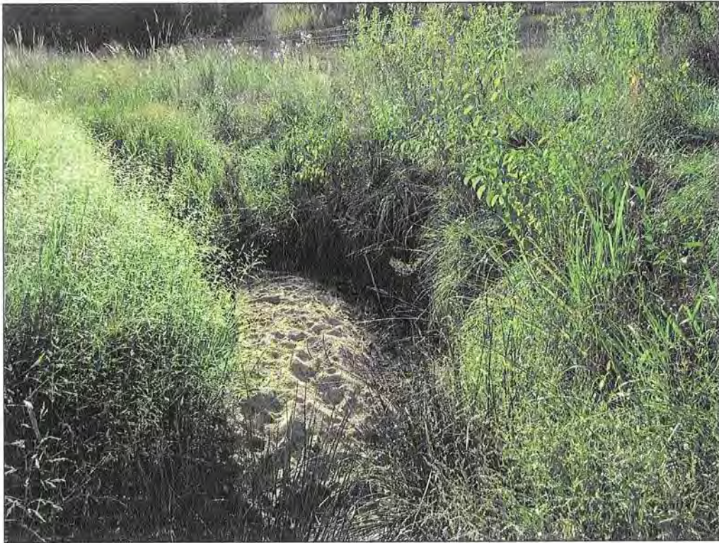
PHOTOGRAPH 48: CROSS SECTION 2 LOOKING UPSTREAM.
