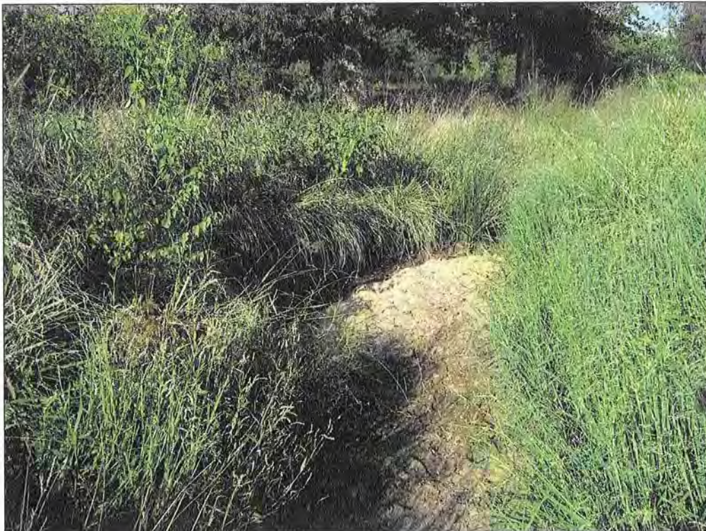
PHOTOGRAPH 49: CROSS SECTION 2 LOOKING DOWNSTREAM.
