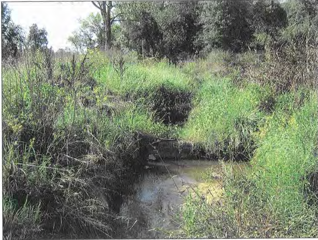
PHOTOGRAPH 27: "A" VANE. STA: 113+80.
