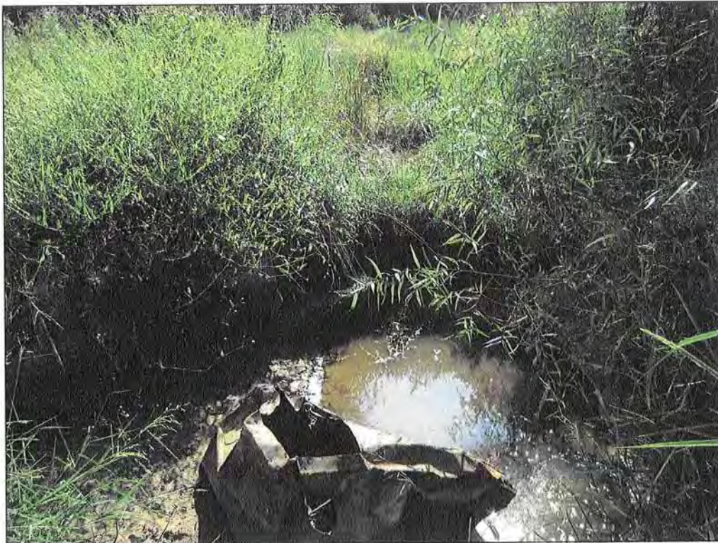
PHOTOGRAPH 28: CROSS VANE. STA: 115+15.
