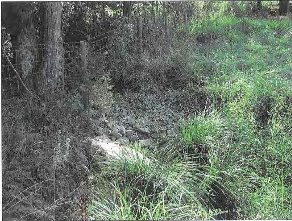
PHOTOGRAPH 37: RIP-RAP. HEAD OF UT-2.
