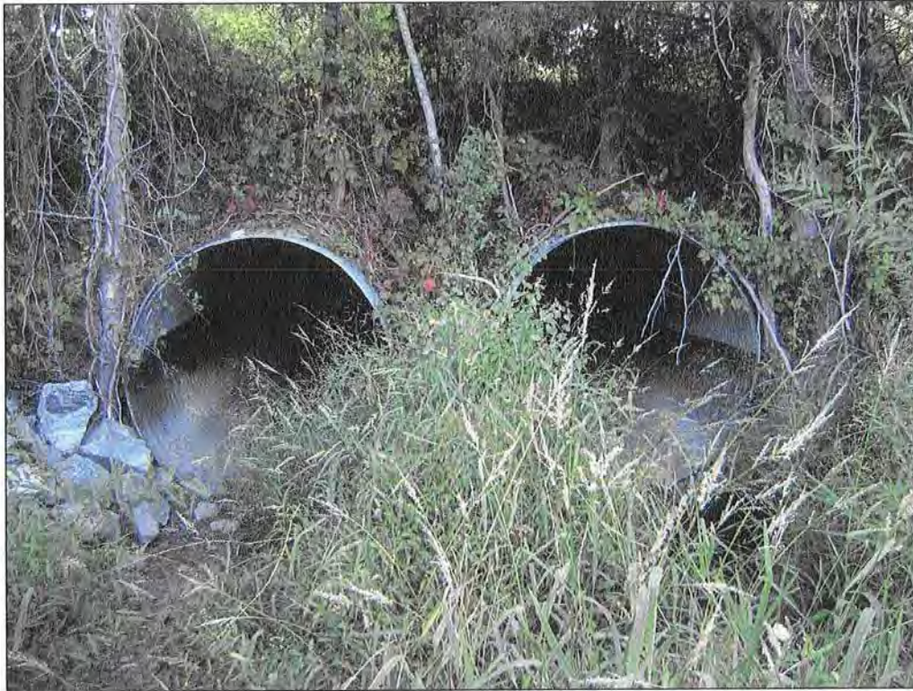
PHOTOGRAPH 1: RIP-RAP. HEAD OF UT-1.
