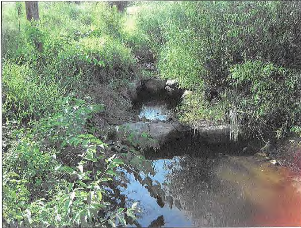
PHOTOGRAPH 19: "A" VANE. STA: 109+14.
