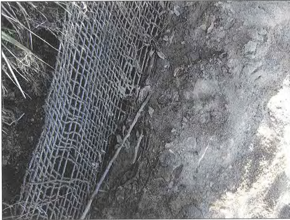
PHOTOGRAPH 52: CROSS SECTION 2 LOOKING AT THE SUBSTRATE COMPOSITION.
