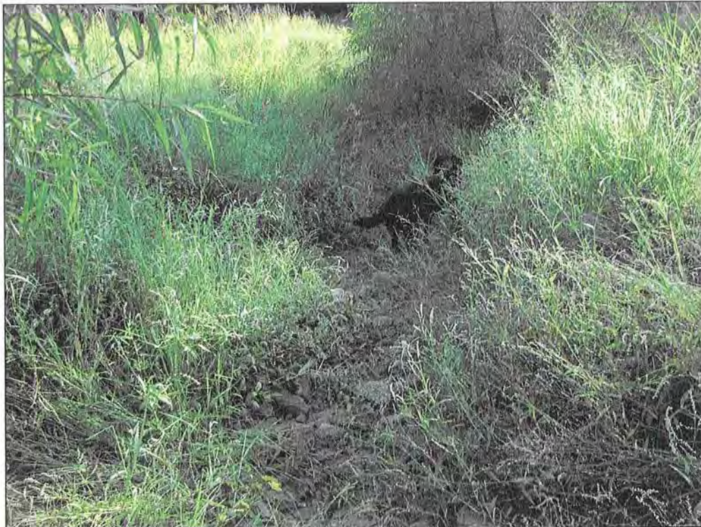
PHOTOGRAPH 4: CONSTRUCTED RIFFLE. STA: 101+09.
