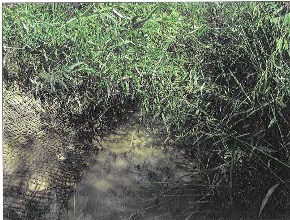
PHOTOGRAPH 59: CROSS SECTION 4 LOOKING DOWNSTREAM.
