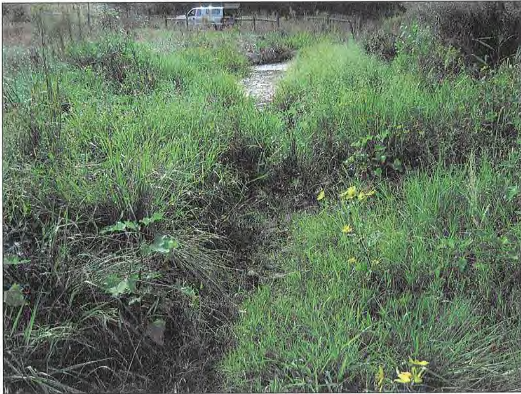
PHOTOGRAPH 25: CONSTRUCTED RIFFLE. STA: 112+15.
