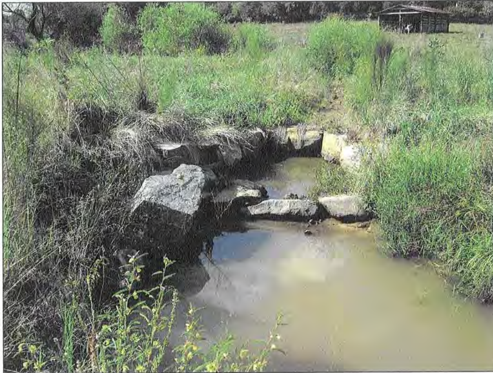
PHOTOGRAPH 29: "A" VANE. STA: 116+29.
