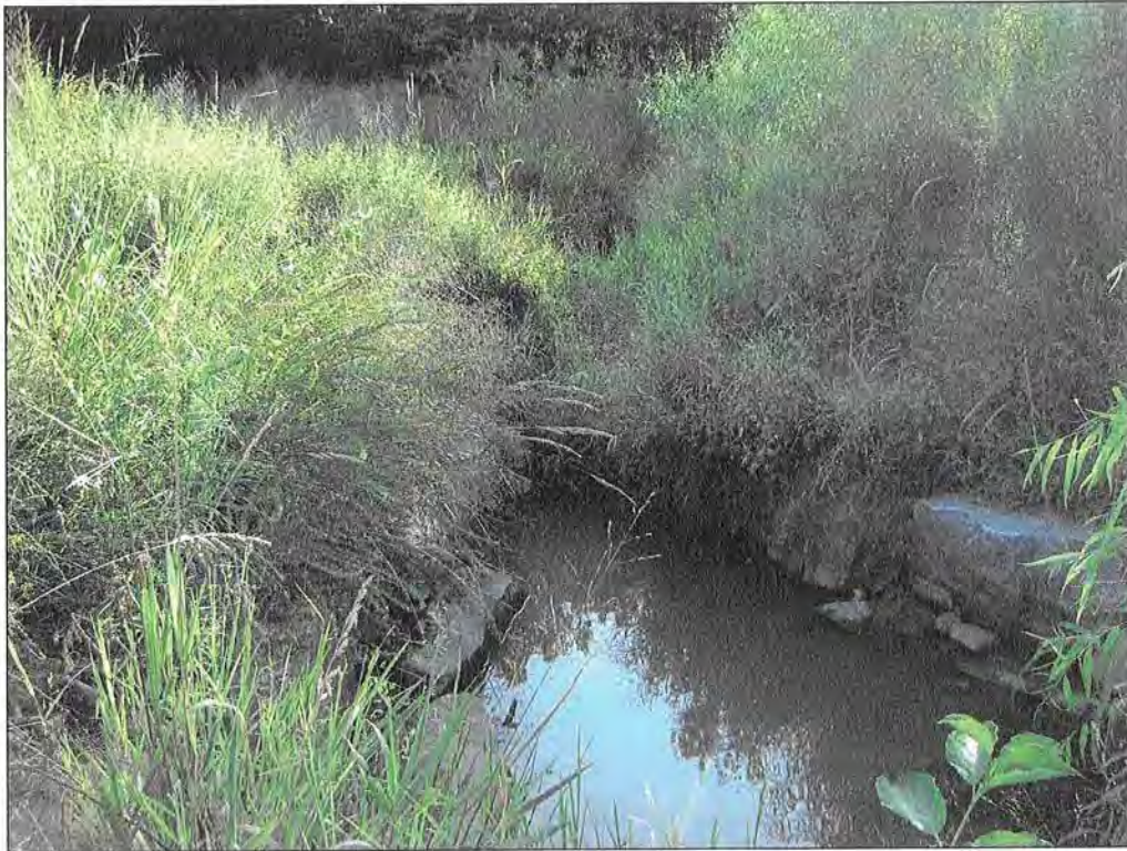
PHOTOGRAPH 3: CROSS VANE. STA: 100+73.
