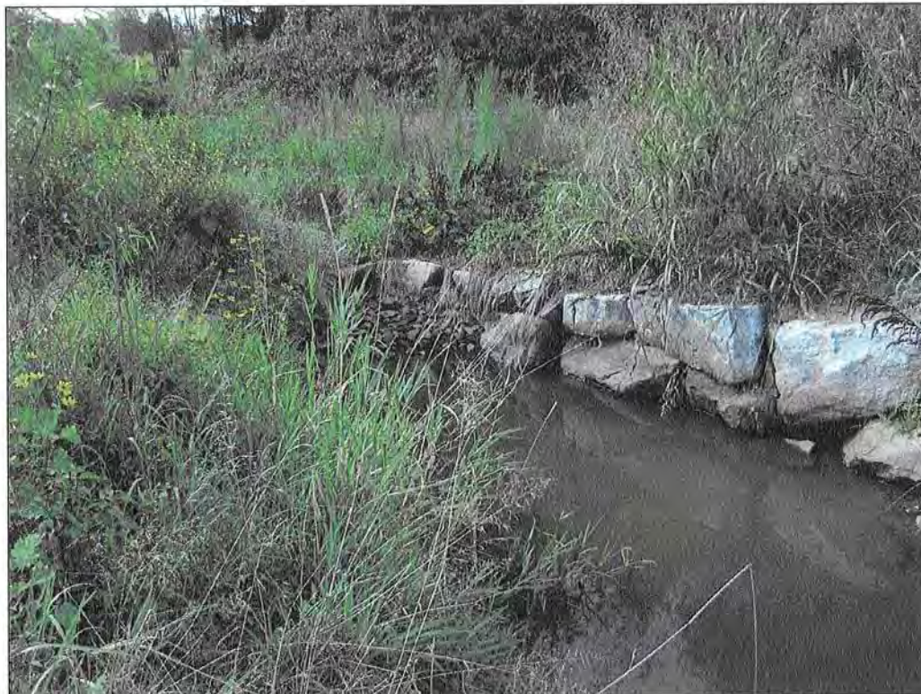
PHOTOGRAPH 26: CROSS VANE. STA: 112+10.
