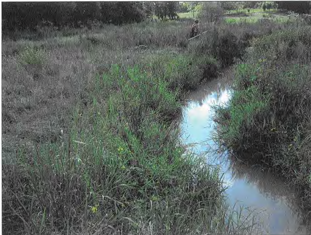
STREAM PROBLEM AREA 7. ERODING BANKS AT STATION 116+92 - 117+10.
