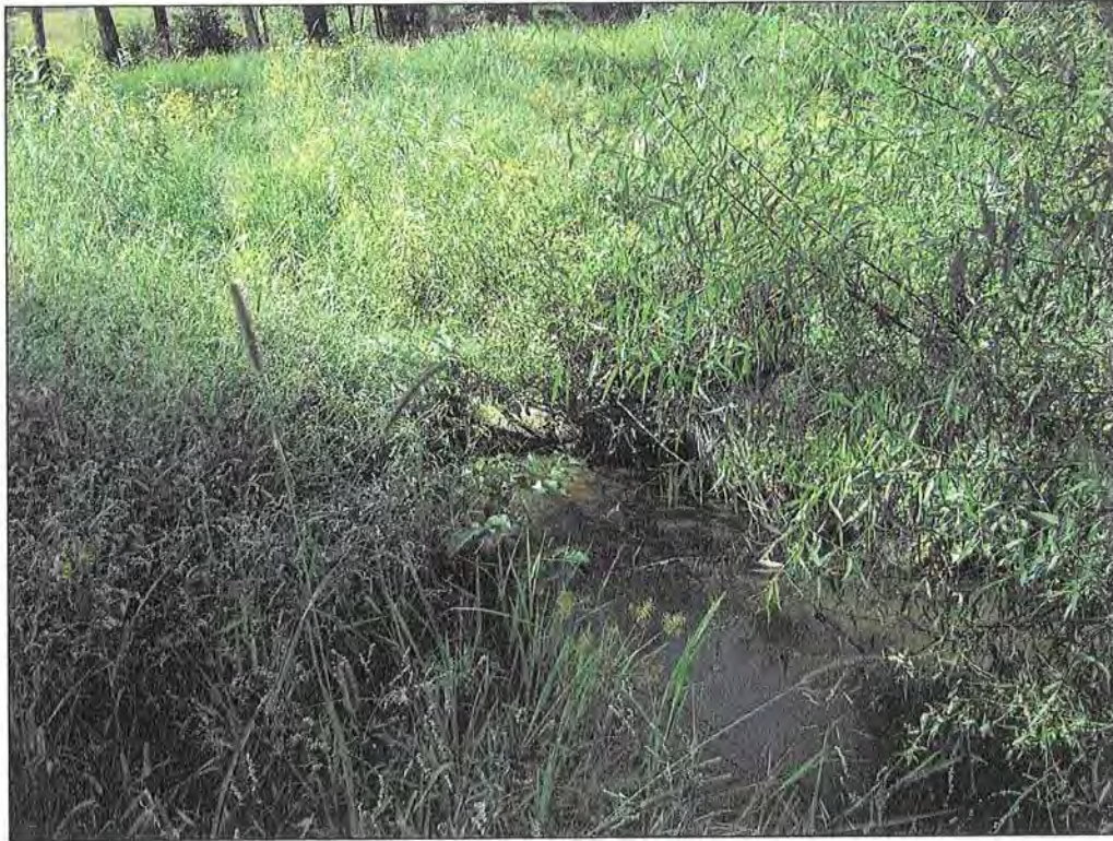
PHOTOGRAPH 21: CROSS VANE. STA: 110+26.
