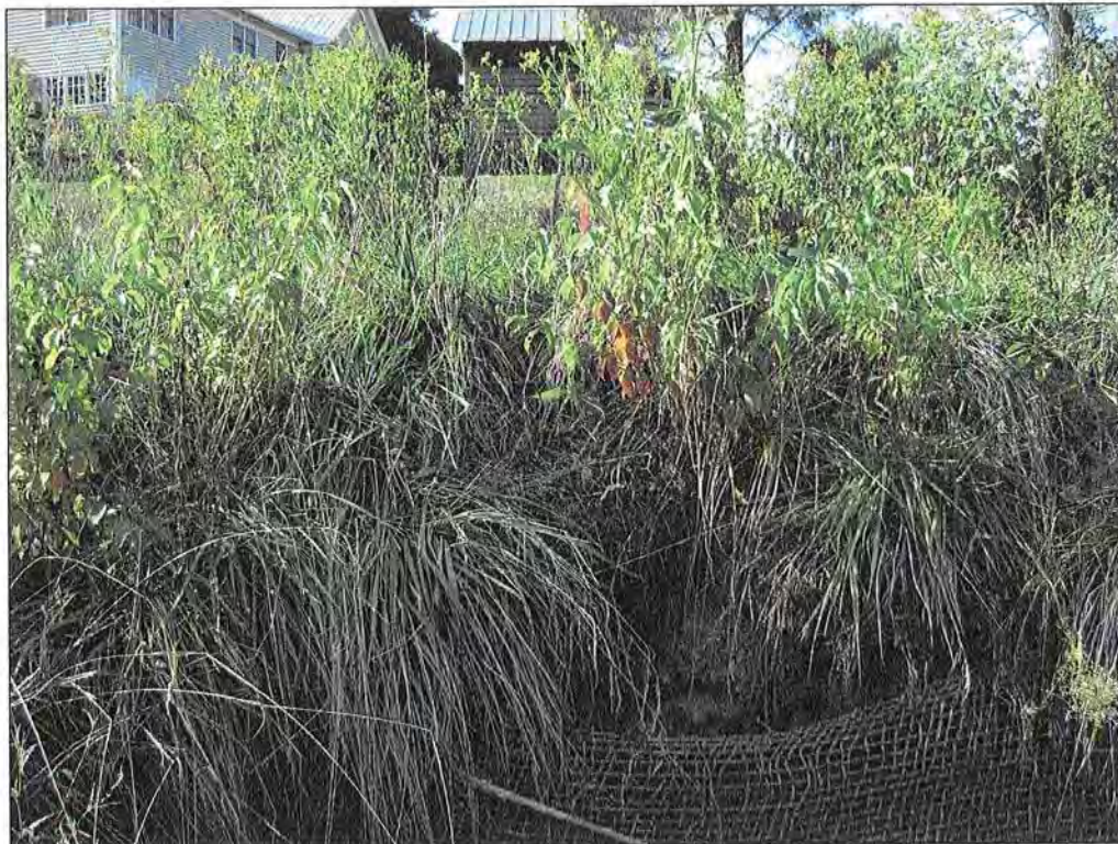
PHOTOGRAPH 51. CROSS SECTION 2 LOOKING AT THE RIGHT BANK.
