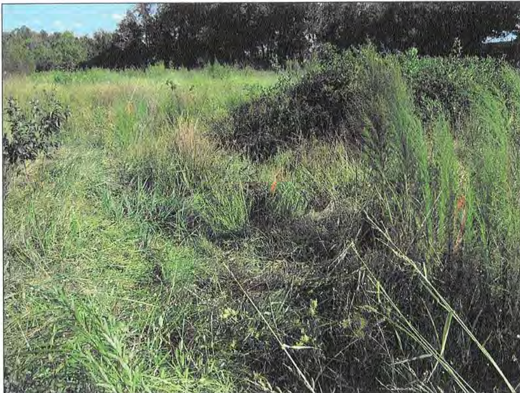
PHOTOGRAPH 64: CROSS SECTION 5 LOOKING DOWNSTREAM.
