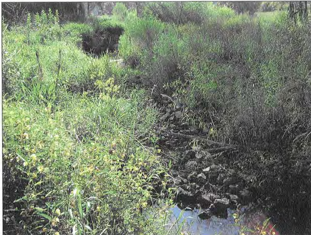
PHOTOGRAPH 20: CONSTRUCTED RIFFLE. STA:109+58.
