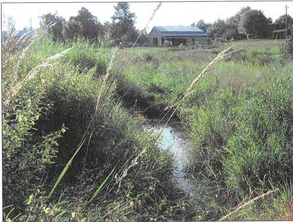
PHOTOGRAPH 13: CROSS VANE. STA: 105+62.
