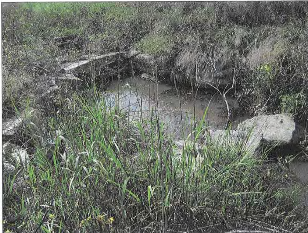
PHOTOGRAPH 30: "A" VANE. STA: 117+58.
