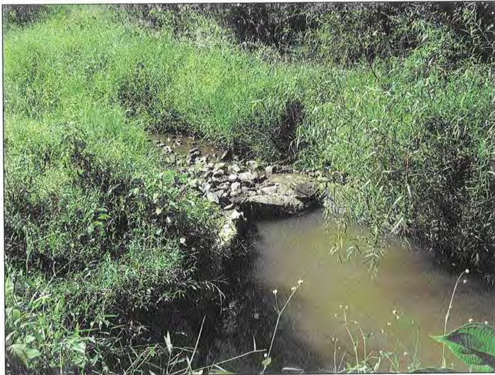
PHOTOGRAPH 36: CROSS VANE. STA: 122+00.
