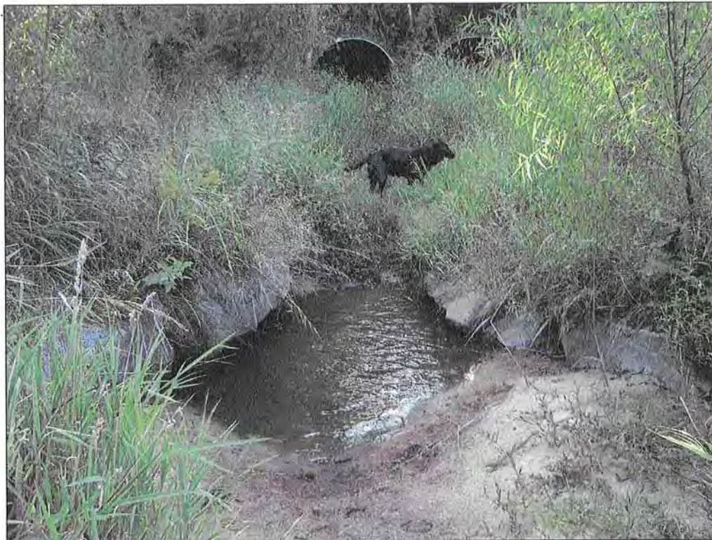
PHOTOGRAPH 2: CROSS VANE. STA: 100+12.
