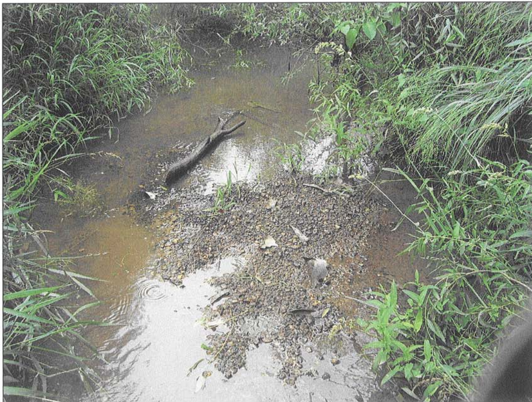
PHOTOGRAPH 33: CONSTRUCTED RIFFLE. STA: 120+25.
