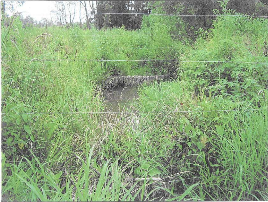
PHOTOGRAPH 23: CROSSING. STA: III+32.
