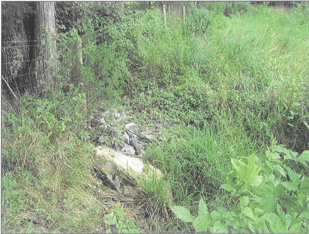
PHOTOGRAPH 37: RIP-RAP. HEAD OF UT-2.
