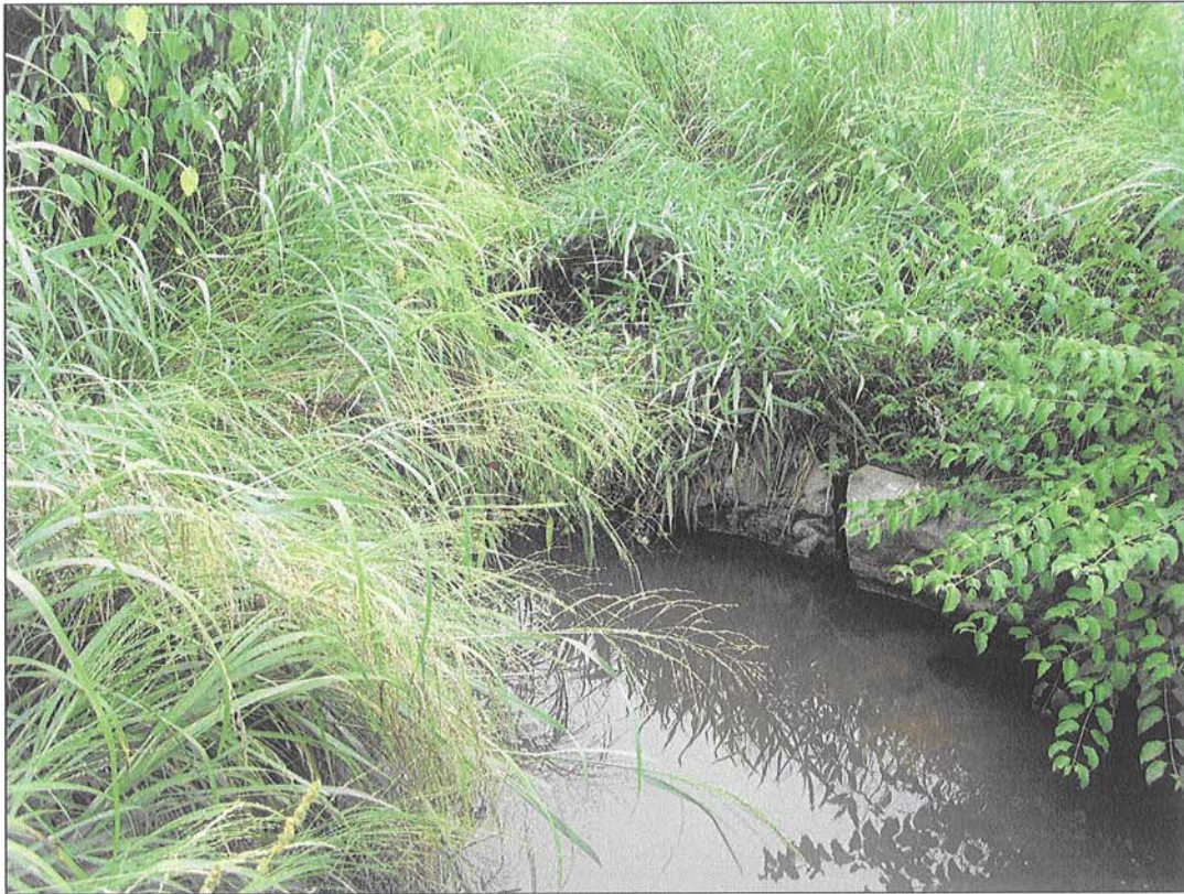
PHOTOGRAPH 13: CROSS VANE. STA: 105+62.
