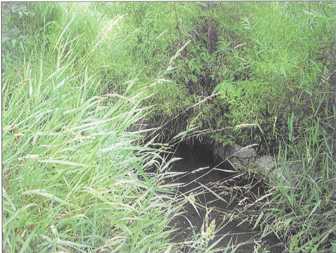
PHOTOGRAPH 14: "A" VANE. STA: 106+60.
