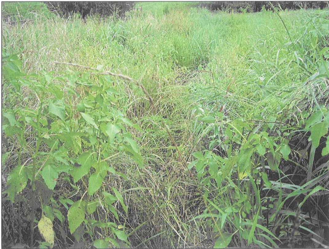
PHOTOGRAPH 9: RIP-RAP FOR WETLAND AREA.
