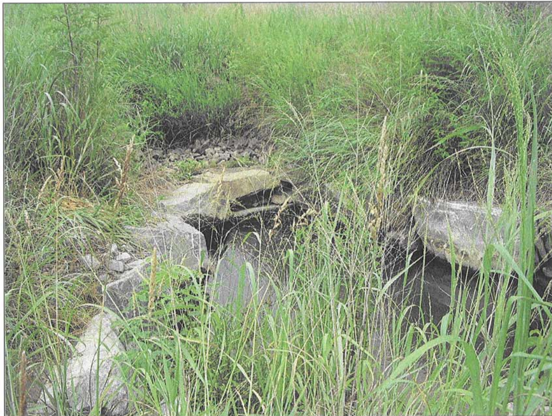
PHOTOGRAPH 30: "A" VANE. STA: 117+58.
