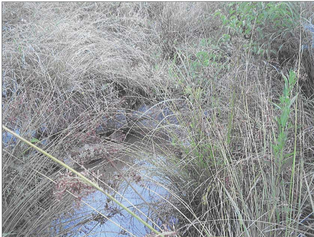
PHOTOGRAPH 38: CROSS VANE. STA: 200+57.
