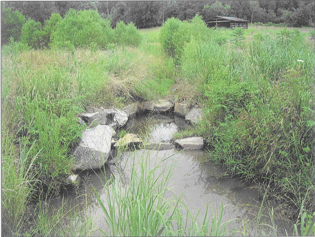
PHOTOGRAPH 29: "A" VANE. STA: 116+29.
