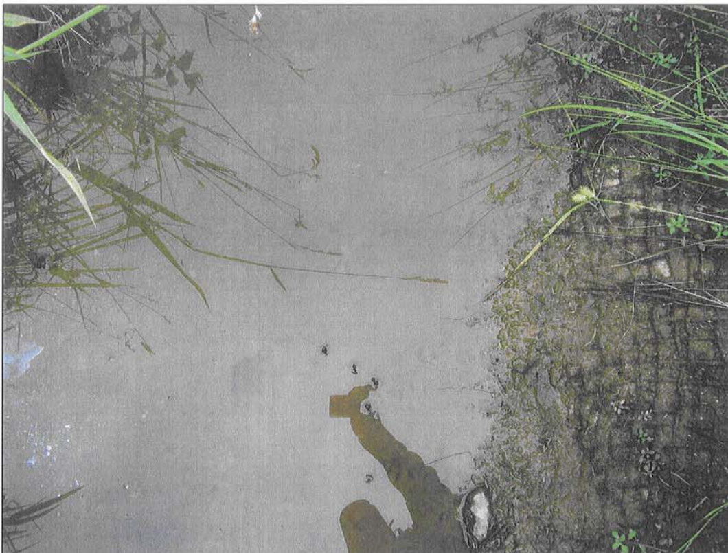
PHOTOGRAPH 72: CROSS SECTION 6 LOOKING AT THE SUBSTRATE COMPOSITION.
