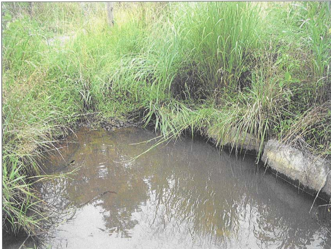
PHOTOGRAPH I2: CROSS VANE, STA: 104+75.
