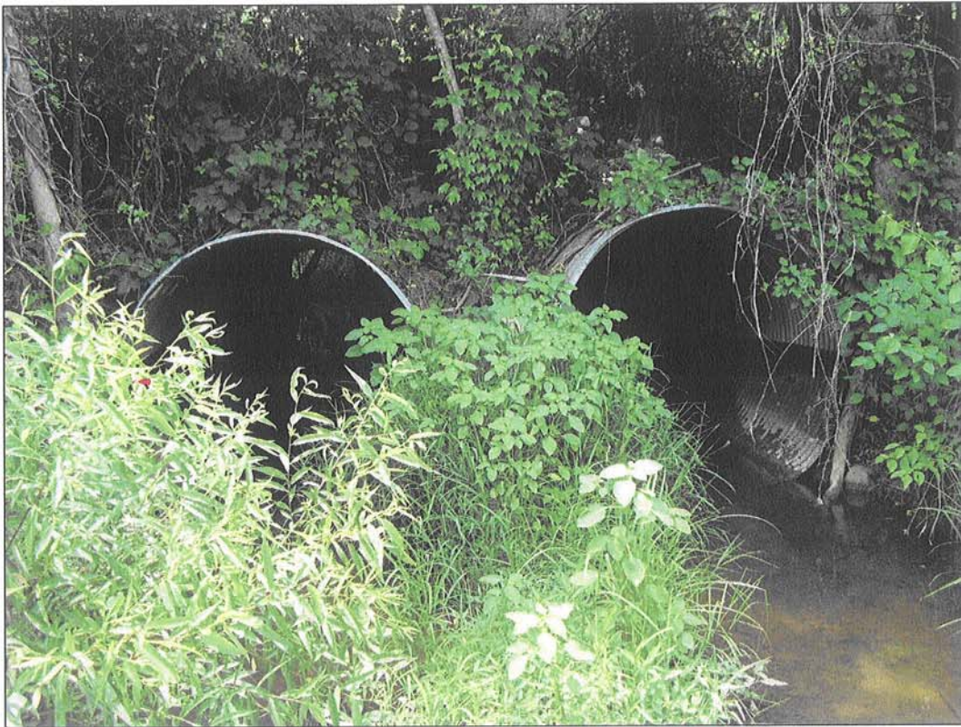
PHOTOGRAPH 1: RIP-RAP. HEAD OF UT-I.
