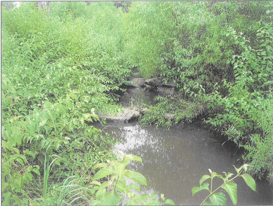
PHOTOGRAPH 19: "A" VANE. STA: 109+14.
