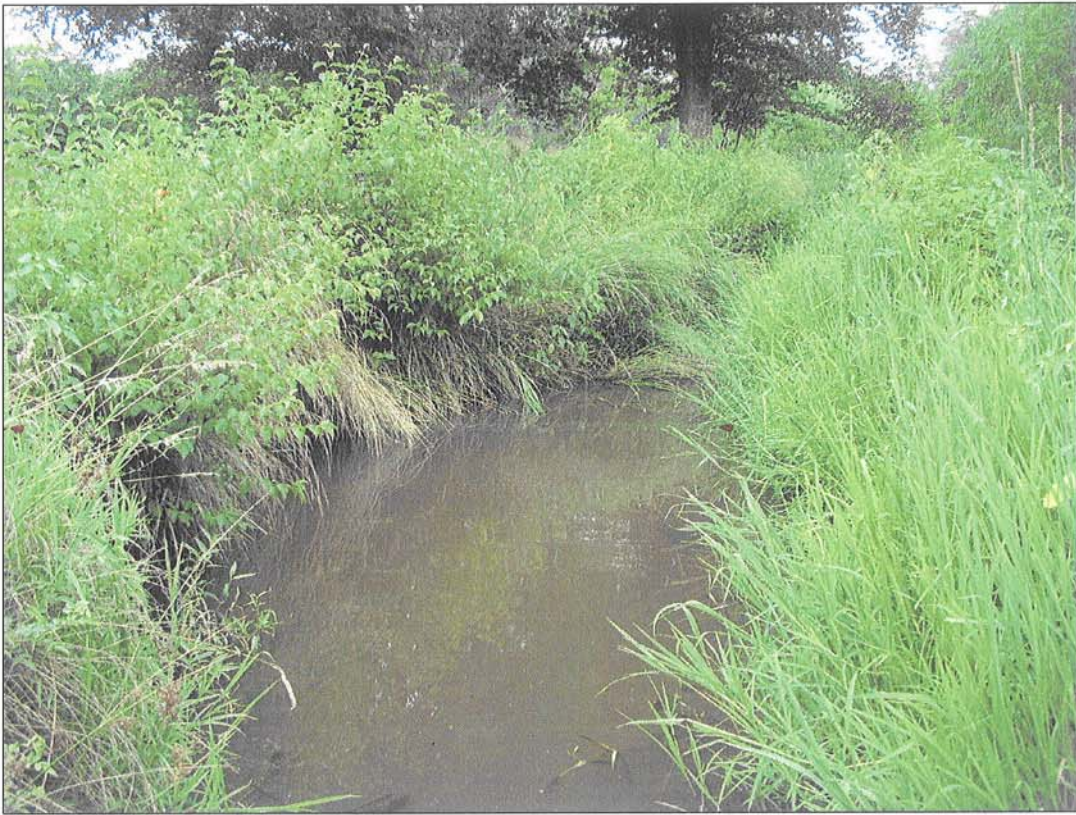
PHOTOGRAPH 5: CROSS VANE. STA: 101+40.
