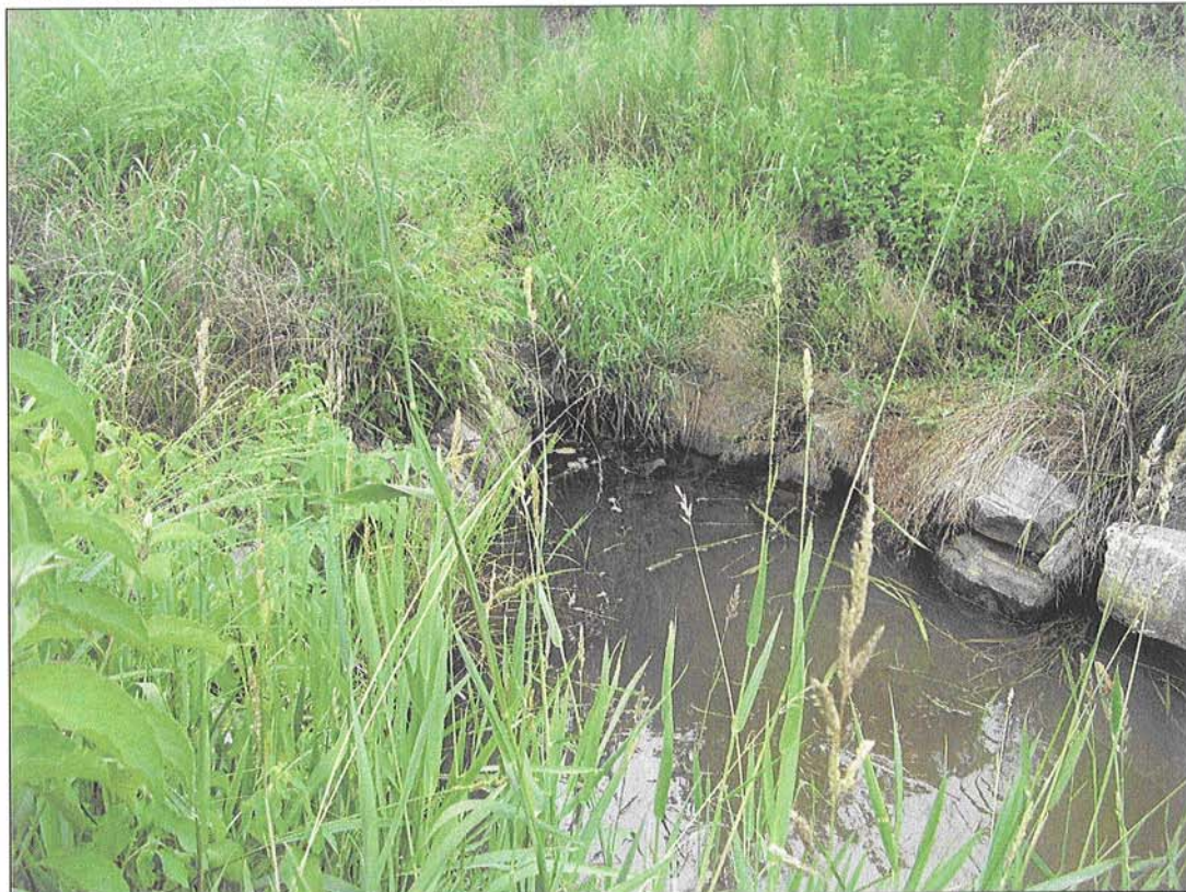
PHOTOGRAPH 26: CROSS VANE. STA: 112+10.
