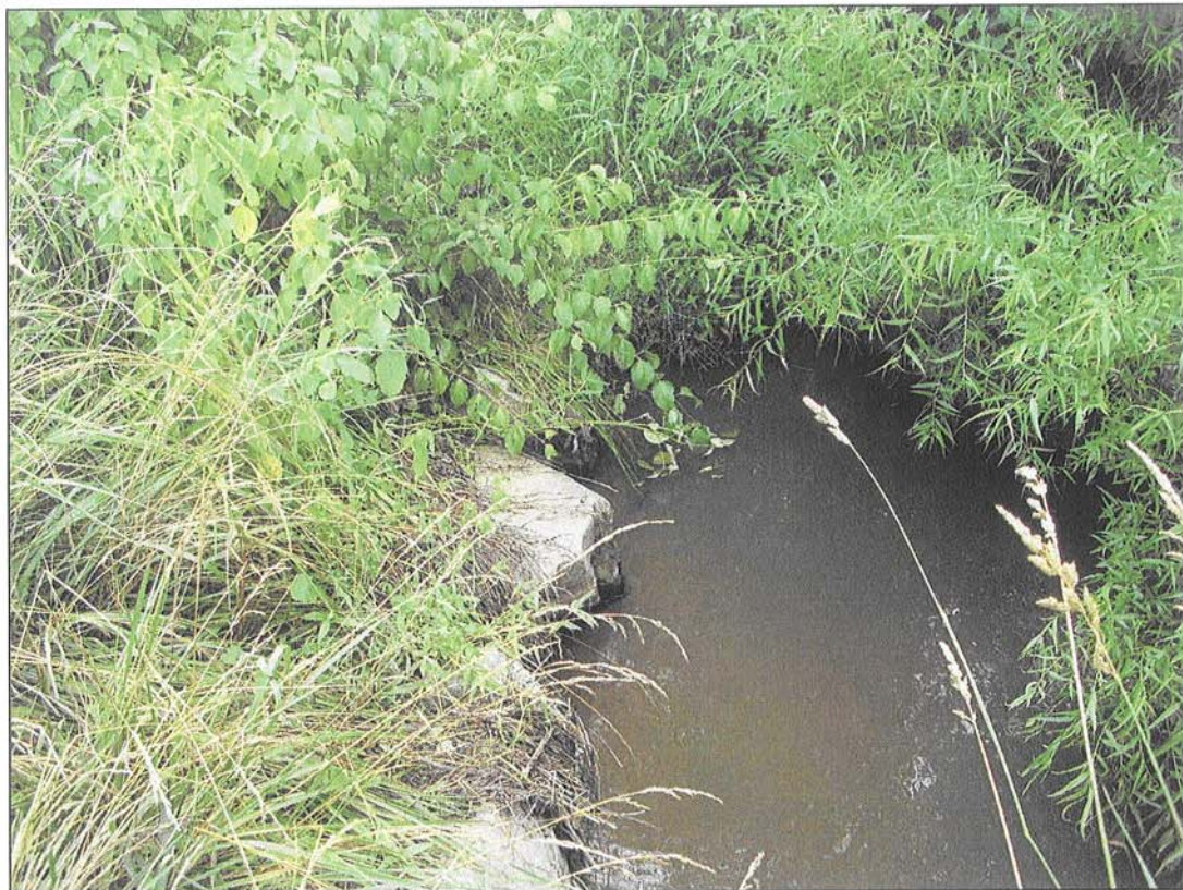
PHOTOGRAPH 28: CROSS VANE. STA: 115+15.
