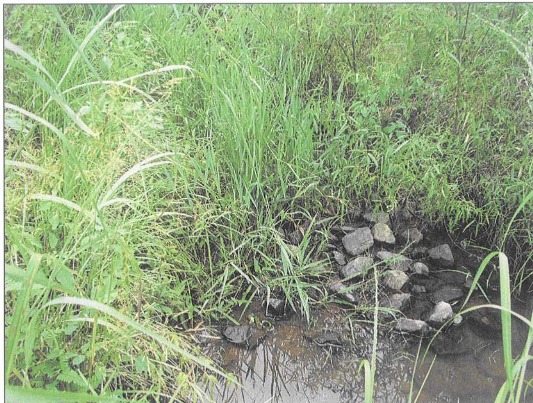
PHOTOGRAPH 20: CONSTRUCTED RIFFLE. STA:109+58.
