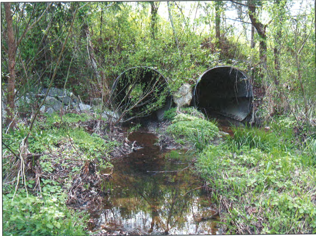
PHOTOGRAPH 1: RIP-RAP. HEAD OF UT-1.
