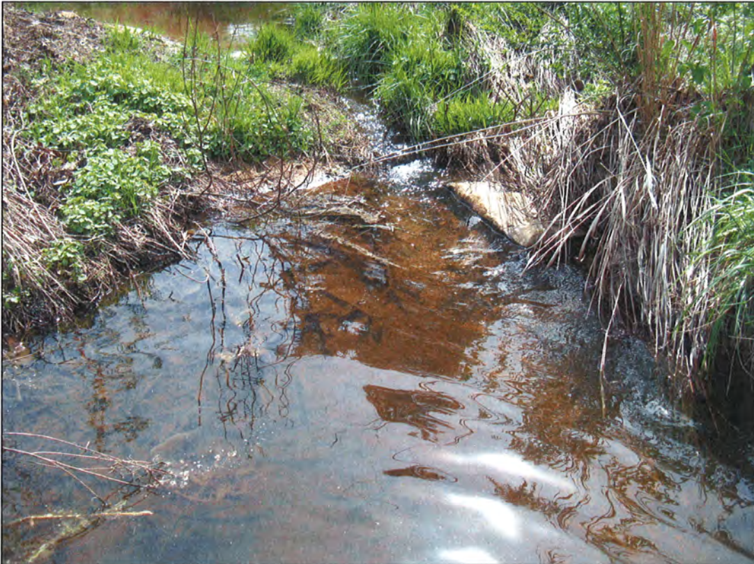
PHOTOGRAPH I2: CROSS VANE. STA: 104+75.
