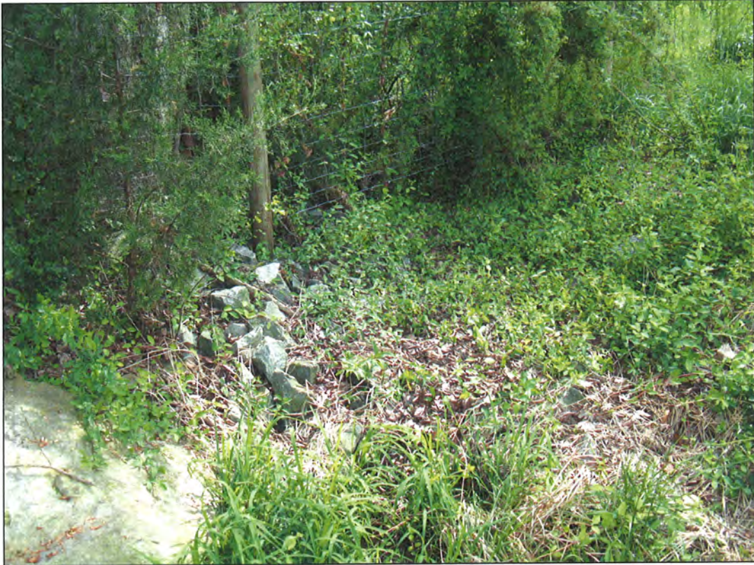
PHOTOGRAPH 37: RIP-RAP. HEAD OF UT-2.
