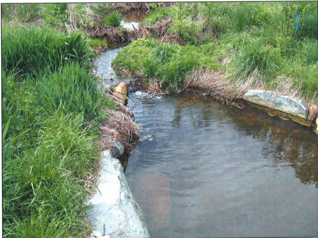
PHOTOGRAPH 24: CROSS VANE. STA: III+66.
