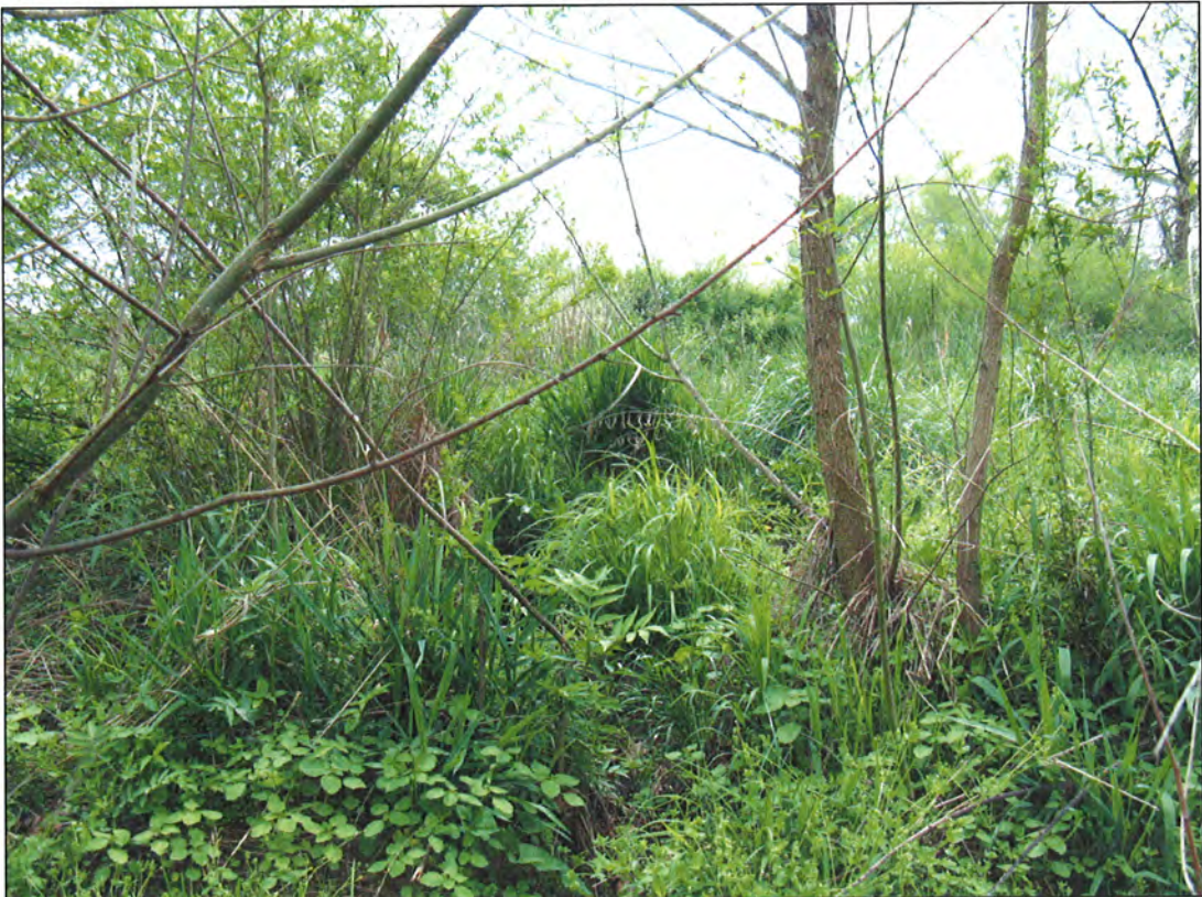
PHOTOGRAPH 34: RIP-RAP. WETLAND DRAINAGE.
