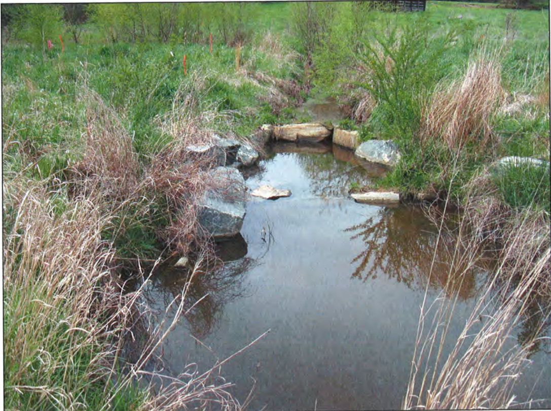
PHOTOGRAPH 29: "A" VANE. STA: 116+29.
