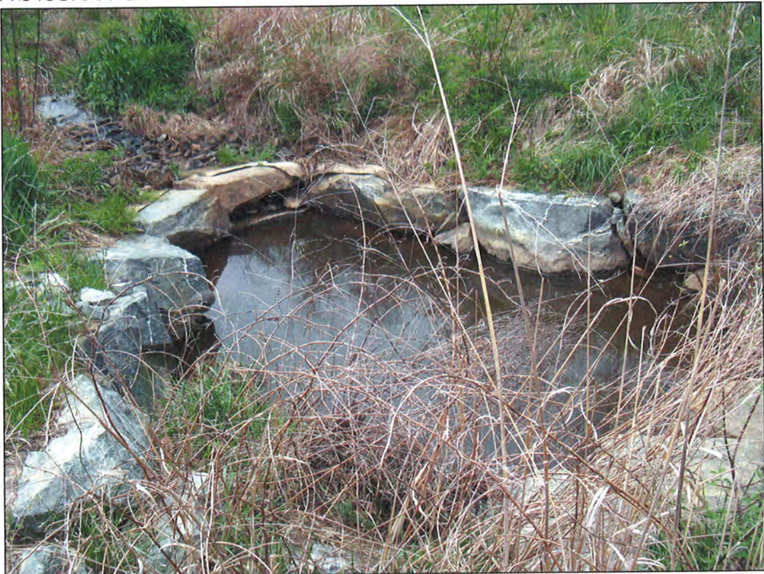
PHOTOGRAPH 30: "A" VANE. STA: 117+58.
