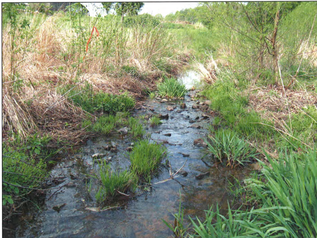
PHOTOGRAPH 4: CONSTRUCTED RIFFLE. STA: 101+09.
