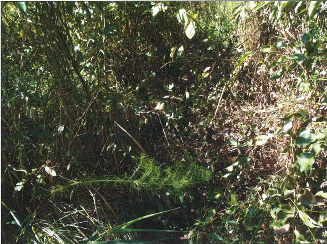
PHOTOGRAPH 42: CROSS VANE. STA: 203+58.
