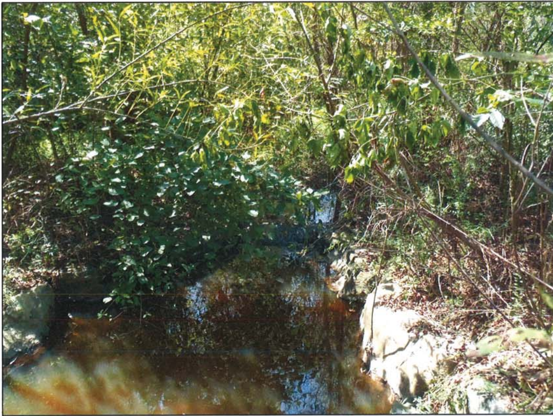
PHOTOGRAPH 17: CROSS VANE. STA: 108+11.
