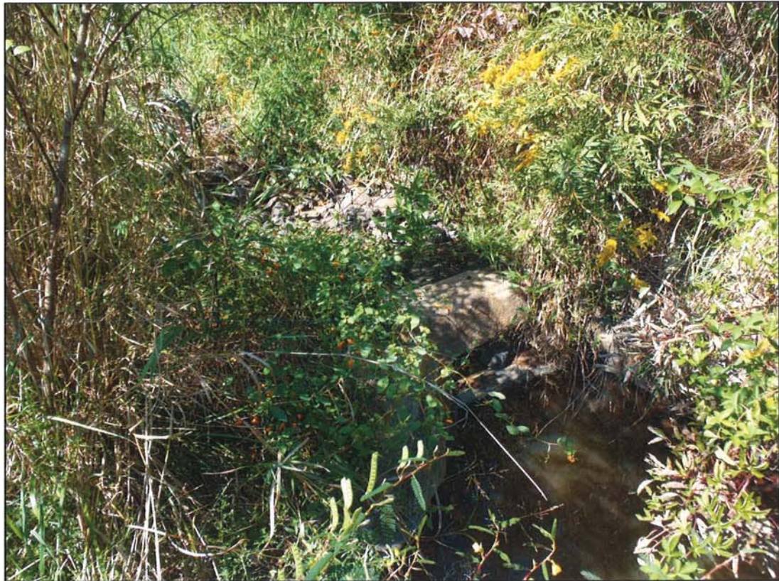
PHOTOGRAPH 30: "A" VANE. STA: 117+58.
