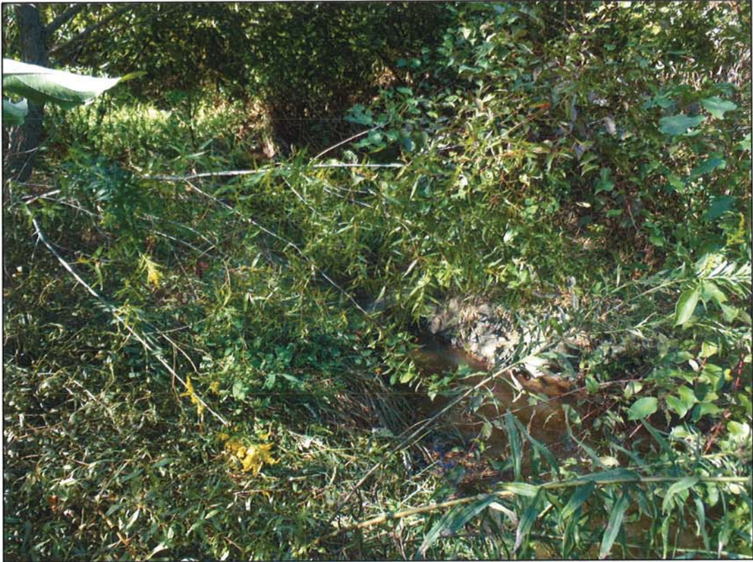
PHOTOGRAPH 13: CROSS VANE. STA: 105+62.
