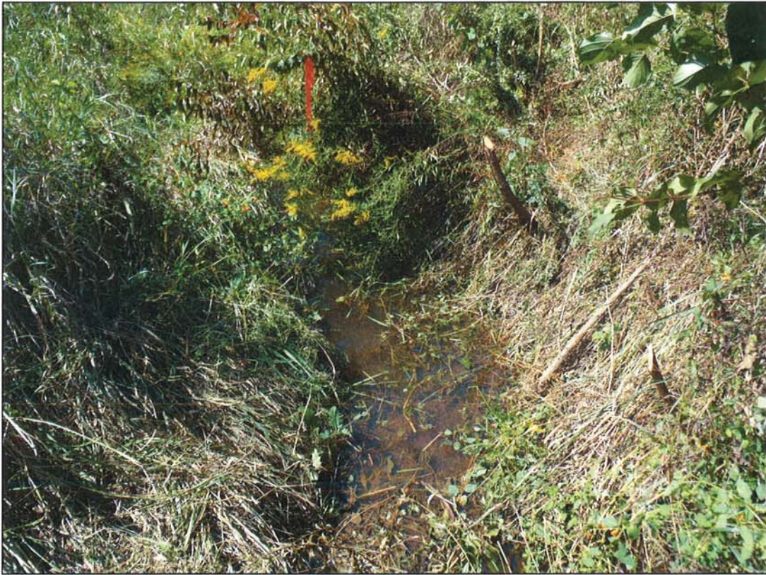
PHOTOGRAPH 53: CROSS SECTION 3 LOOKING UPSTREAM.
