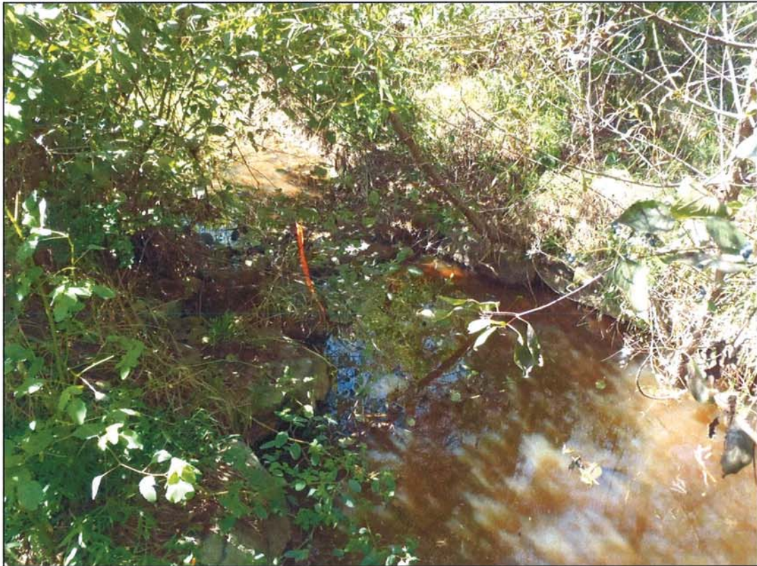
PHOTOGRAPH 28: CROSS VANE. STA: 115+15.
