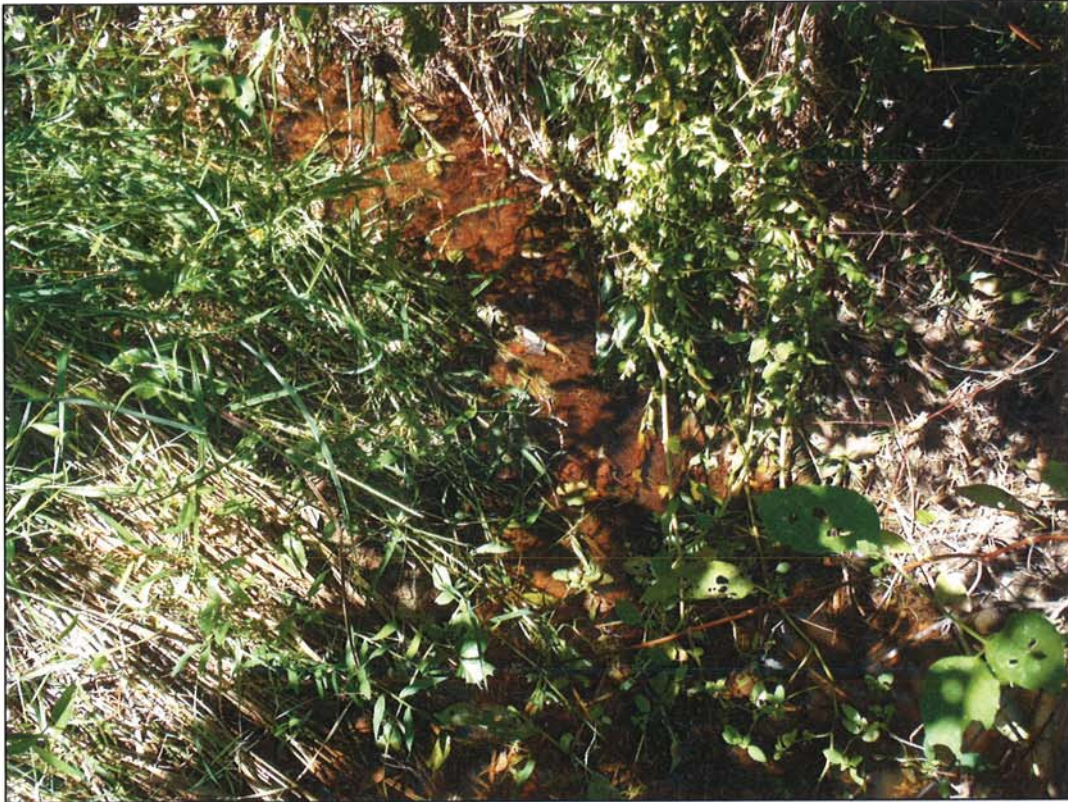
PHOTOGRAPH 7: CROSS VANE. STA: 102+85.
