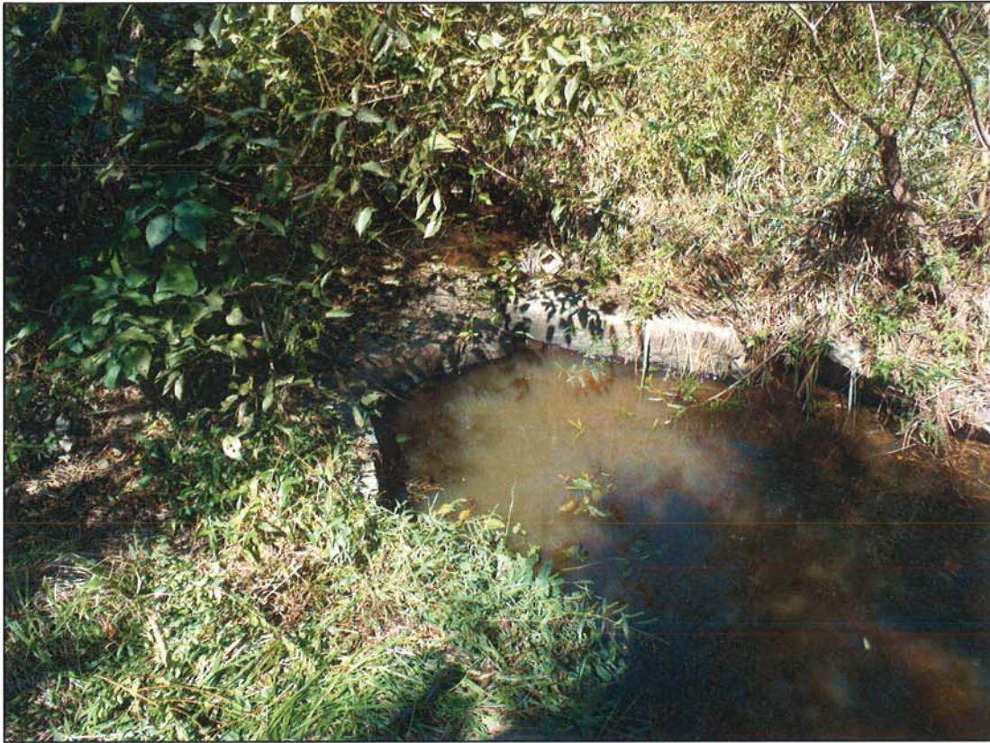
PHOTOGRAPH 31: "A" VANE. STA: 118+46.
