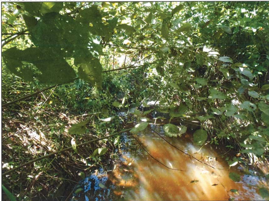
PHOTOGRAPH 12: CROSS VANE. STA: 104+75.
