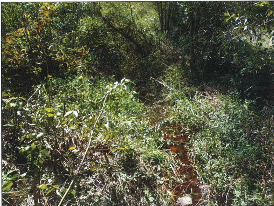
PHOTOGRAPH 4: CONSTRUCTED RIFFLE. STA: 101+09.
