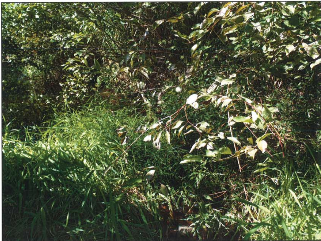
PHOTOGRAPH 8: CONSTRUCTED RIFFLE. STA: 103+15.
