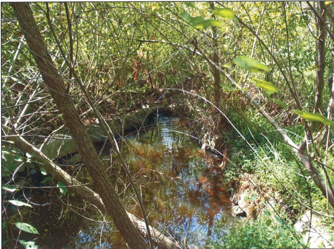
PHOTOGRAPH 16: CROSS VANE. STA: 107+49.
