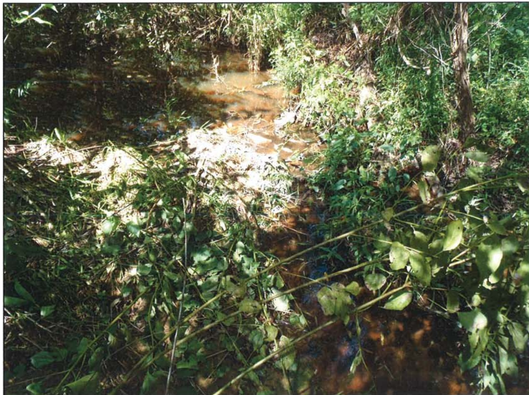
PHOTOGRAPH 22: CONSTRUCTED RIFFLE. STA: 110+58.
