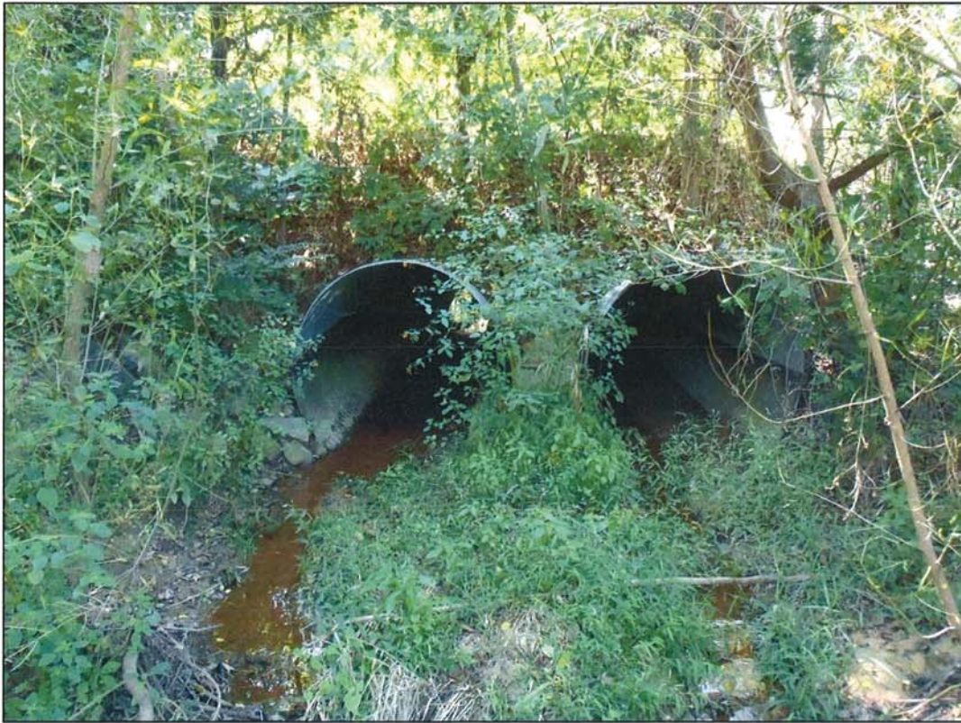
PHOTOGRAPH 1: RIP-RAP. HEAD OF UT-I.
