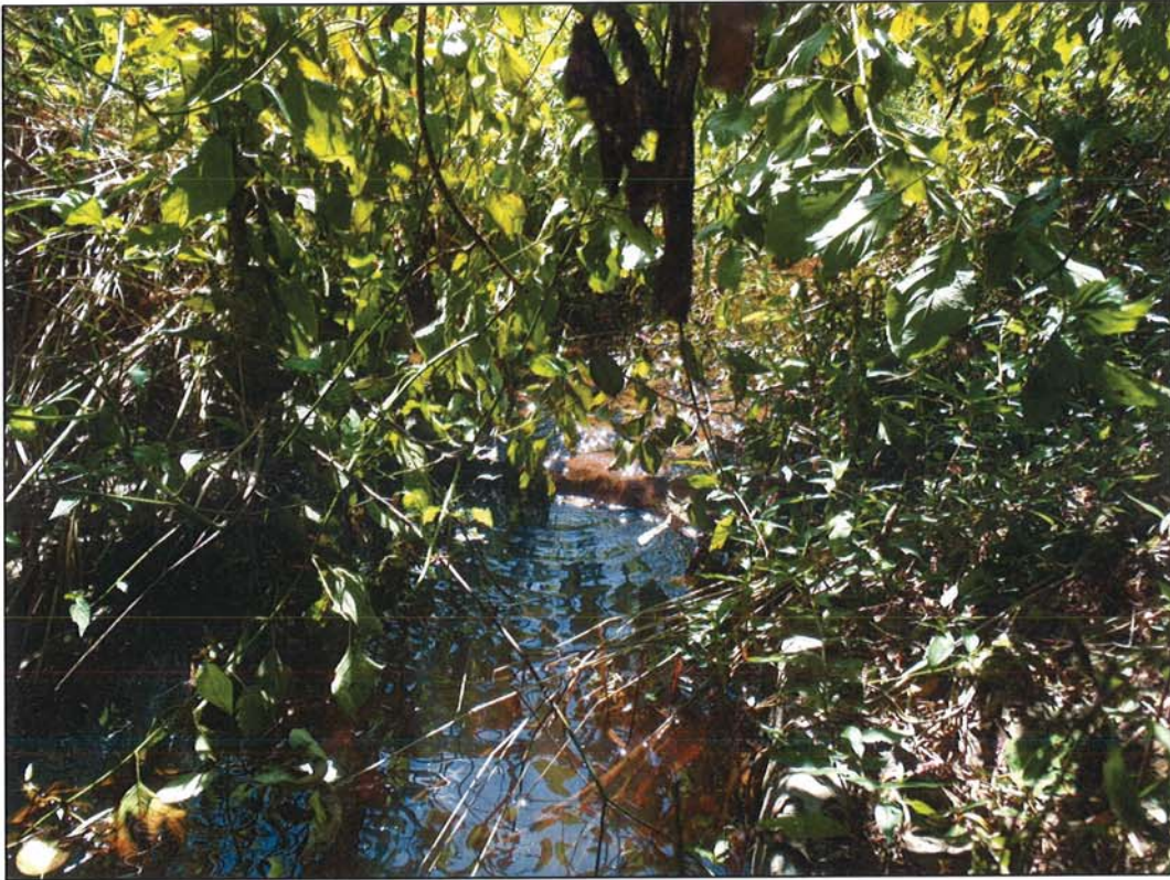
PHOTOGRAPH 3: CROSS VANE. STA: 100+73.
