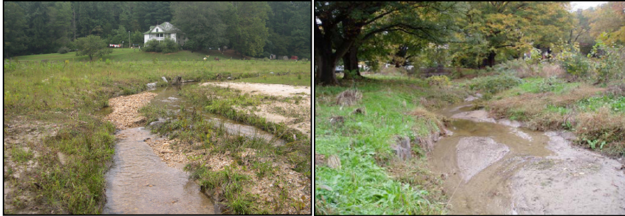
Exhibit 1. Examples of bar features warranting concern related to cataloging item 1.1.1 of the assessment
