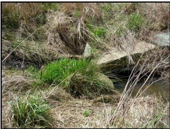
Photo point 7: Looking at Channel
