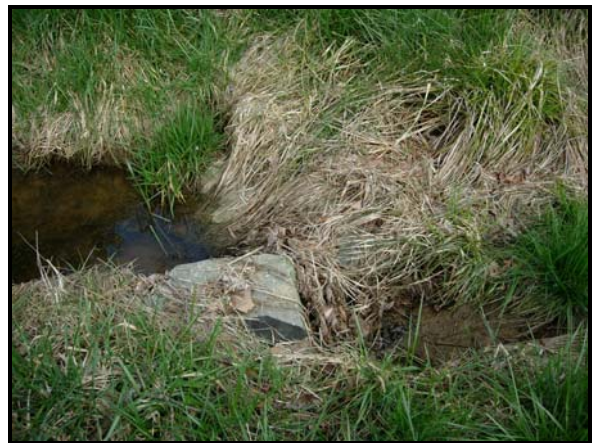
Photo point 4: Looking at Channel
