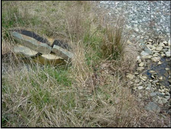
Photo point 1: Looking at Channel
