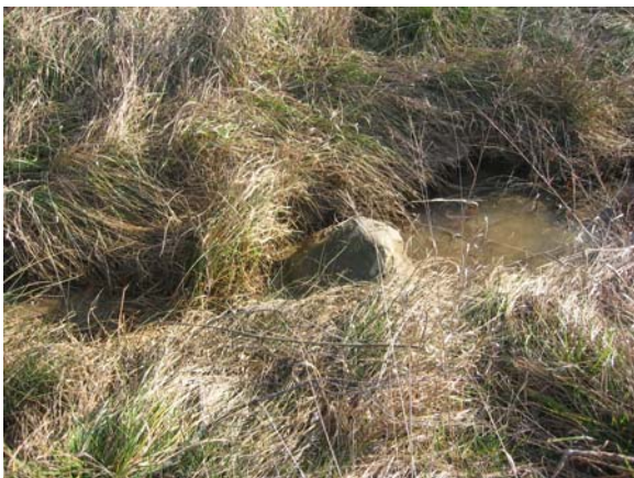
Photo point 3: Looking at Channel
