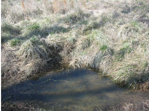
Photo 1: Representative bank erosion problem area (17+60 along plan view).
