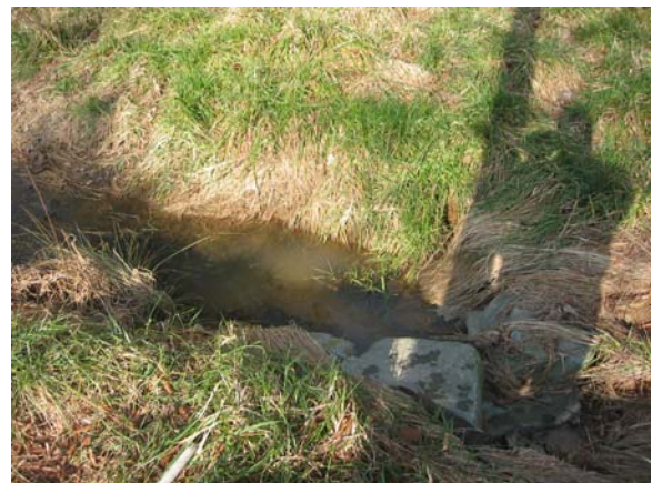
Photo point 4: Looking at Channel
