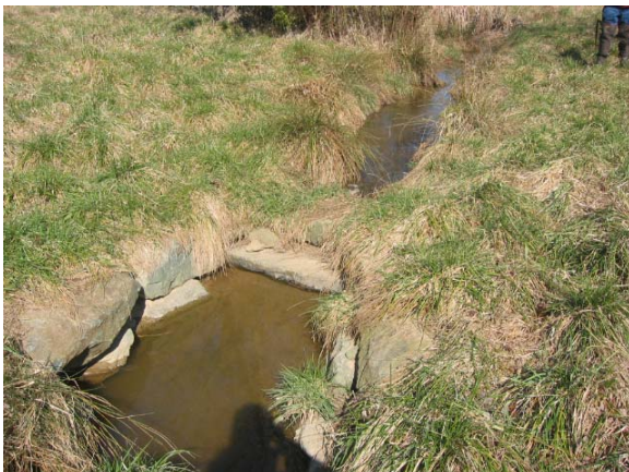
Photo 3: Representative problem cross vane (20+94 along plan view).
