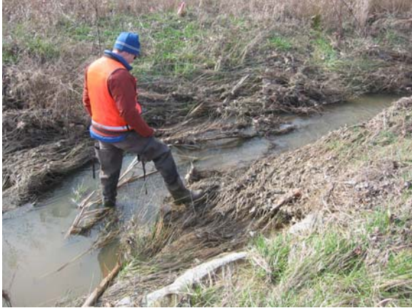
Photo 1: Representative grass aggradation problem area (Station 12+66 along plan view).
