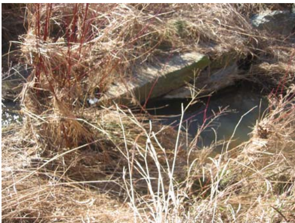
Photo point 7: Looking at Channel
