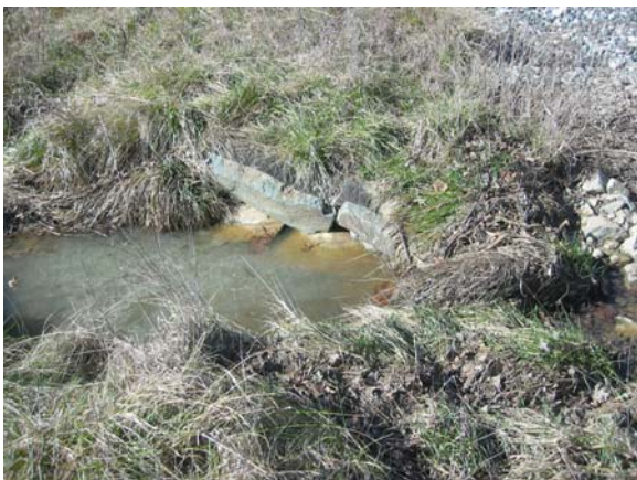
Photo point 1: Looking at Channel
