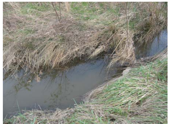
Photo point 2: looking at channel
