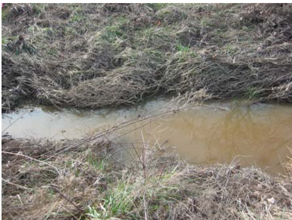
Photo point 3: looking at channel
