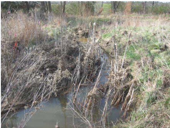
Photo 2: Representative cattail aggradation problem area (Station 10+85 along plan view).
