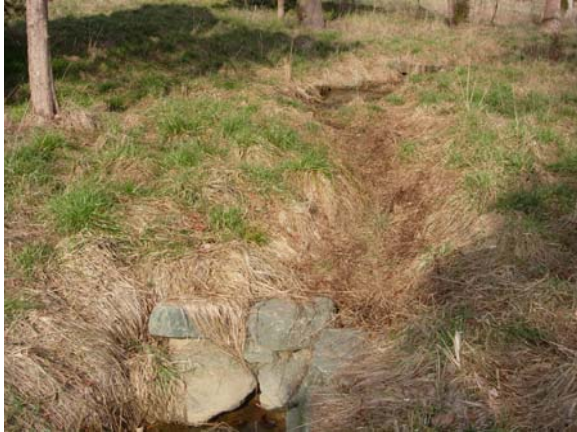
Photo 1: Representative aggradation problem area (Station No. 14+07 – 14+22; view upstream on 3-03-2008).
