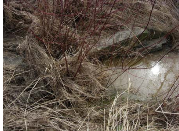
Photo 2: Representative problem cross vane (Station No. 20+34; view of left bank on 3-11-2008). Note current coming out of bank on downstream of left arm (in view), an indication of water piping around the arm.
