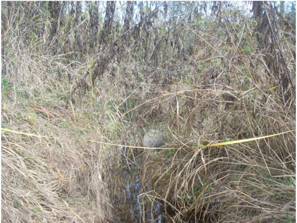
Photo point 5 (R2): View Upstream (10-28-2010)
