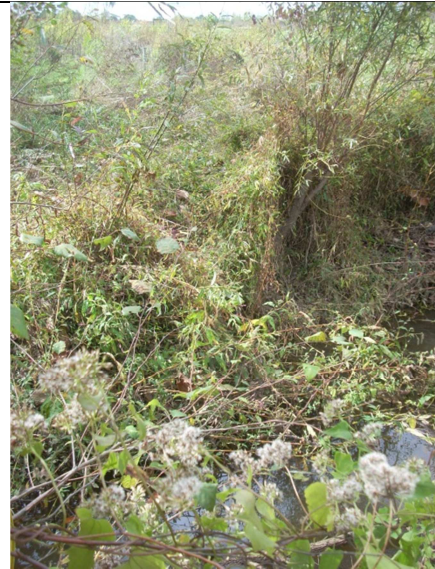
Photo point 5 (R3): Facing Channel (10-28-2010)
