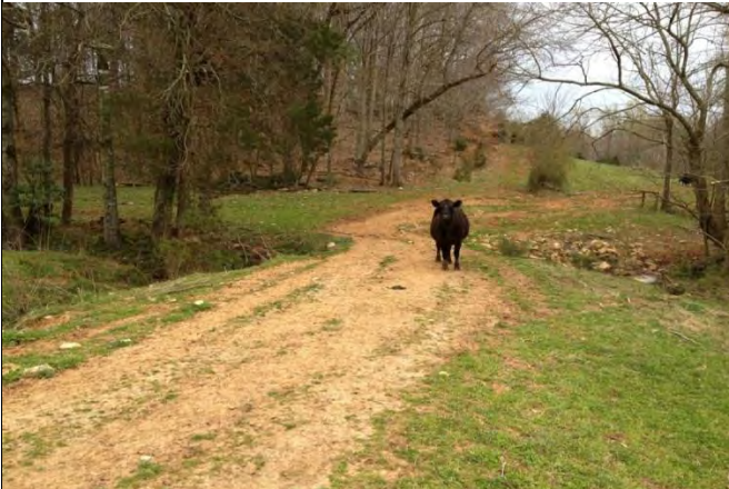
View looking at existing culvert crossing to be improved (4/5/13)
