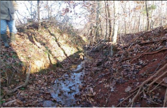
View looking downstream at incised channel near beginning of Reach R1 (2/23/12)
