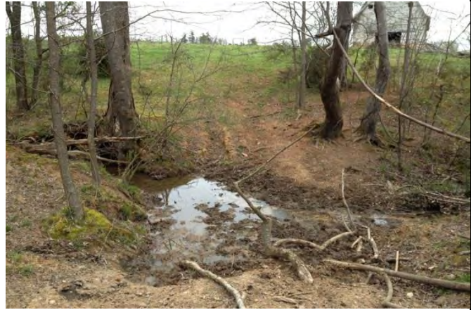
View looking at left stream bank erosion near existing crossing at beginning of proposed restoration (4/5/13)
