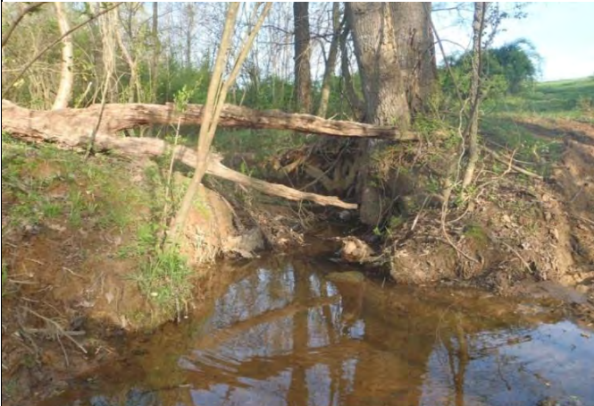
View looking upstream at stream bank erosion and channel incision near upstream end (3/29/12)
