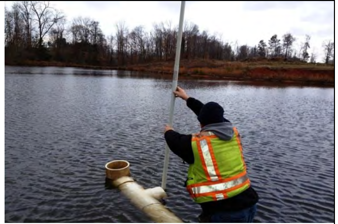
View looking at 8" Dia. PVC inlet for draining man-made farm pond upstream of Reach R1 (1/2/13)
