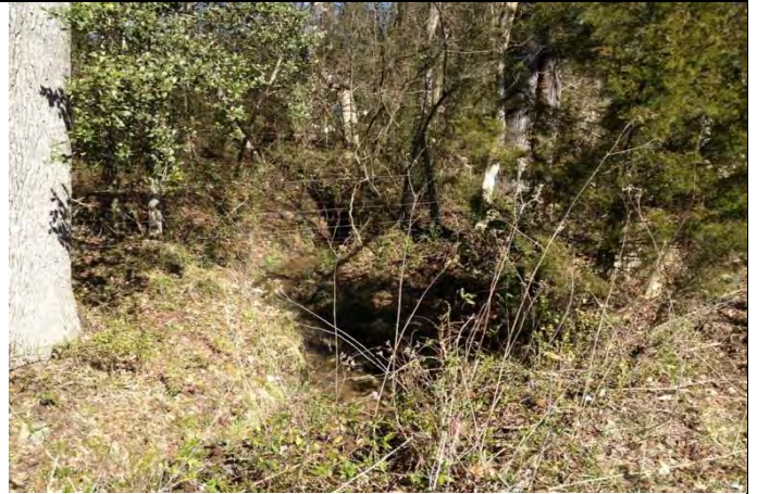
View looking existing hillside seep (2/20/13)
