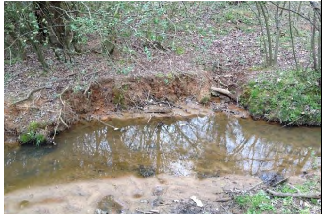
View looking at right stream bank erosion/scour (4/5/13)
