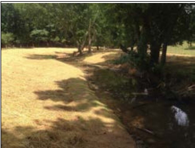
Reach 4, view upstream at 55+00 (June 5, 2014)
