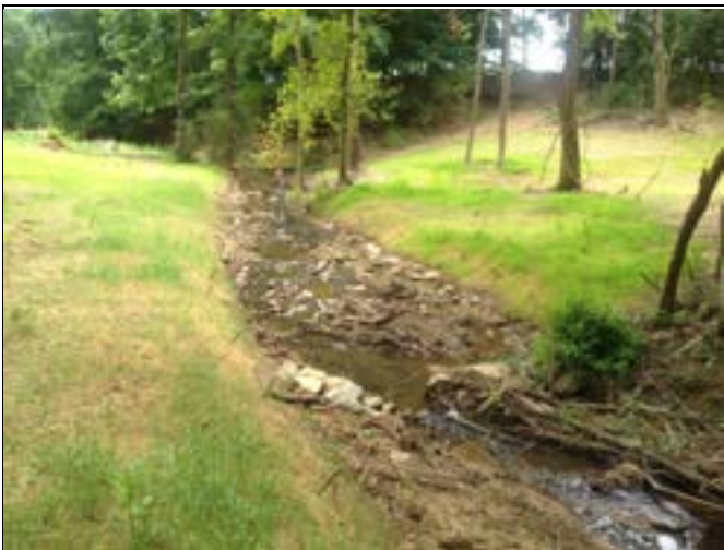
Reach 5, view downstream at station 28+00 (June 5, 2014)
