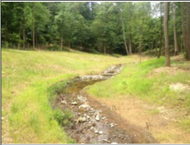
Reach 3, view upstream at station 12+50 (June 5, 2014)
