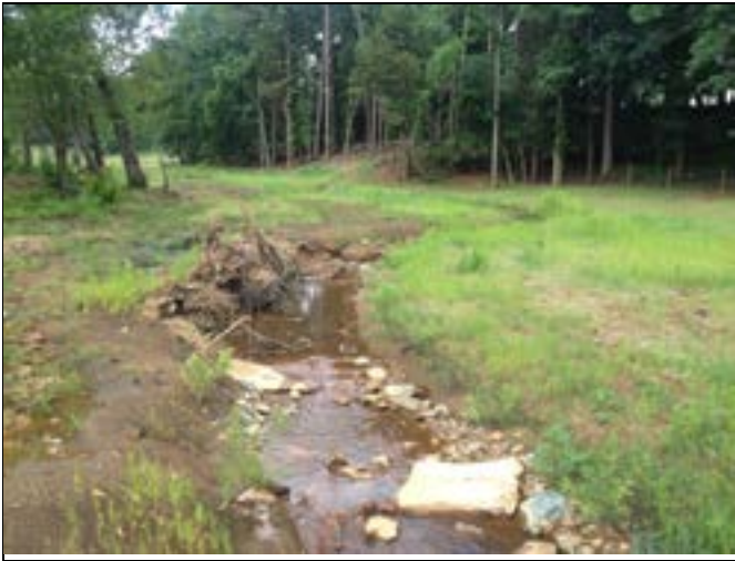
Reach 5, view upstream at station 24+25 (June 12, 2014)
