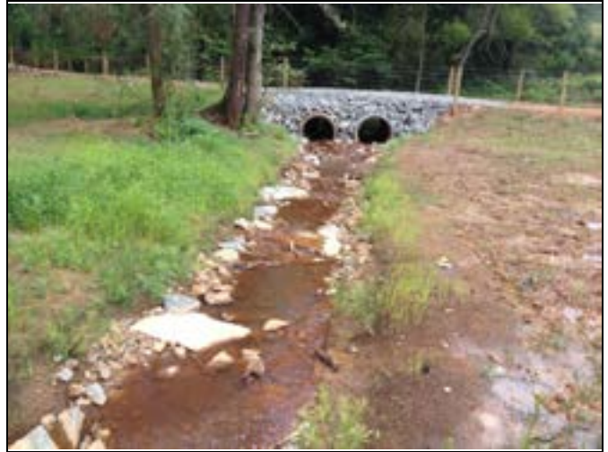
Reach 5, view downstream at station 24+00 (June 12, 2014)
