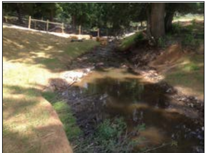
Reach 4, rock J-Hook, view upstream at station 53+75 (June 5, 2014)
