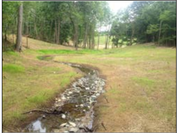
Reach 3, view downstream at station 10+90 (June 5, 2014)
