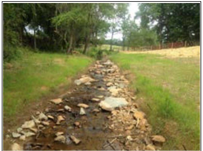
Reach 5, view upstream at station 27+75 (June 5, 2014)
