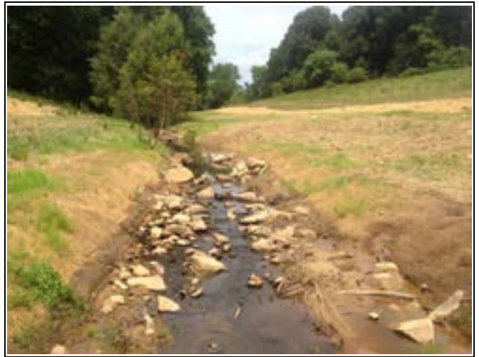
Reach 4, view upstream at station 32+00 (June 5, 2014)
