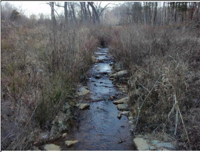
Reach R5 – View upstream of culvert, Station 24+75
