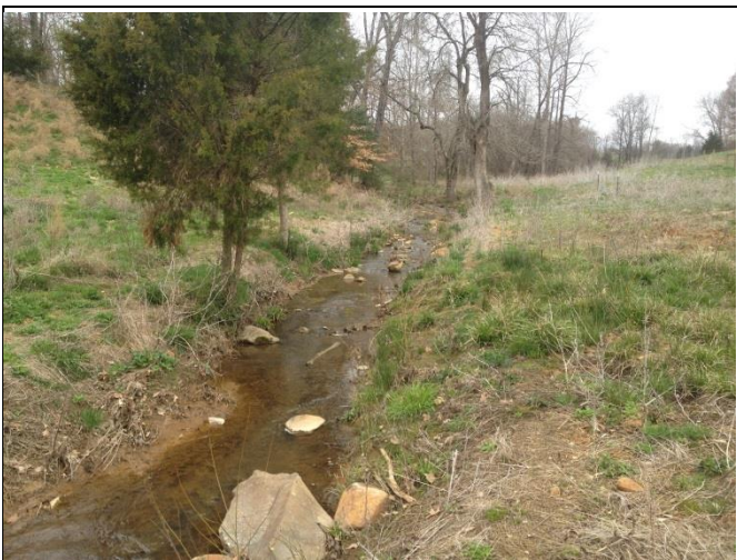
Reach R4 – View upstream, Station 32+50
