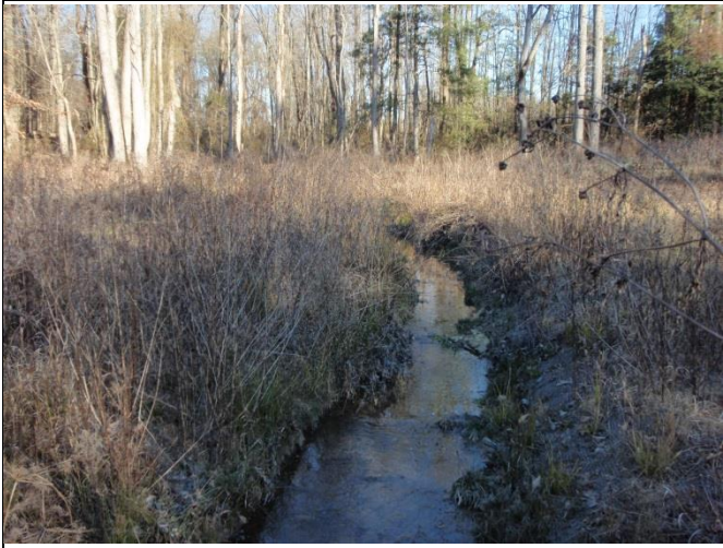
Reach R5 – View upstream, Station 12+00
