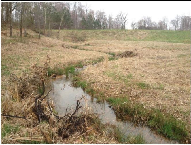
Reach R1 – View upstream, Station 12+25
