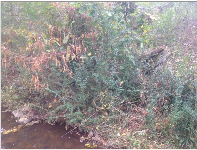
3) Vegetation Problem Area #1 – Vicinity of Reach 5 Station 28+50, October 2015
