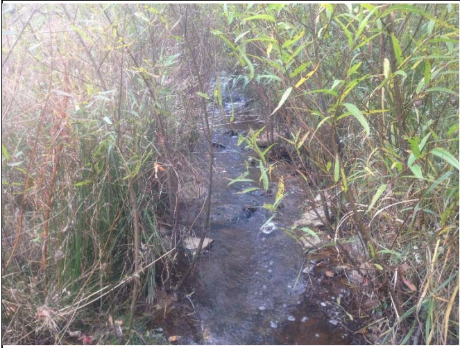
Reach R5 – View upstream of culvert, Station 24+75
