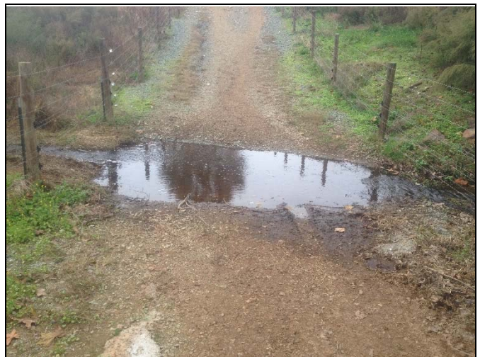
Reach R4 – View of stream crossing, Station 33+00
