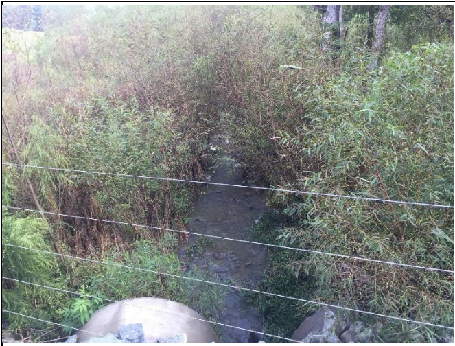
Reach R5 – View upstream of culvert, Station 24+75
