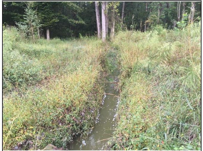
Reach R5 – View upstream, Station 11+50
