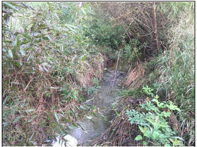
Reach R5 – View upstream, Station 17+25
