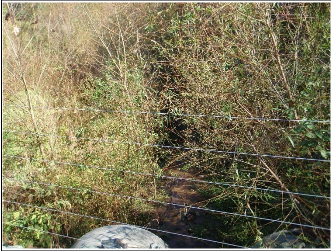
Reach R5 – View upstream of culvert, Station 24+75
