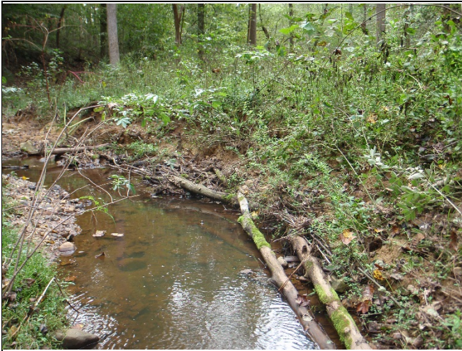
SPA: Bank scour along Reach R4 (~43+50), looking downstream
