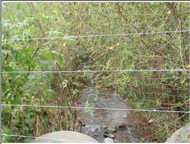
Reach R5 – View upstream of culvert, Station 24+75
