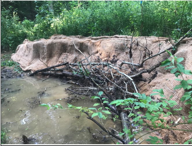
Reach R4 Station 43+50: Additional bank repair with seed and matting (June 2018)
