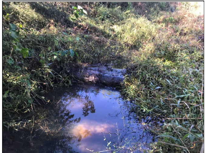
PP-24: Reach R1, view upstream, Station 20+00
