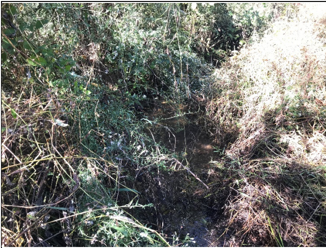
PP-23: Reach R1, view upstream, Station 19+25
