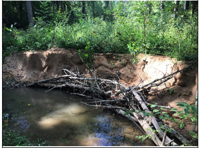
Reach R4 Station 43+50: Bank repair (Sept 2019)
