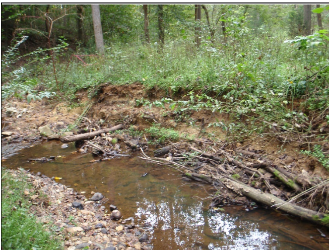
Reach R4 Station 43+50: Previously documented stream bank scour from Hurricane Florence in Sept 2018
