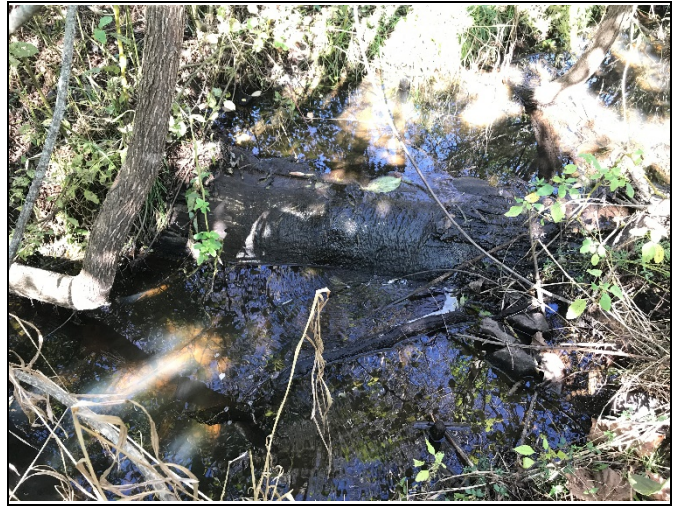
PP-4: Reach R5, view upstream, Station 16+50
