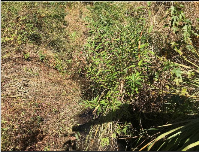
PP-3: Reach R5, view upstream, Station 13+75
