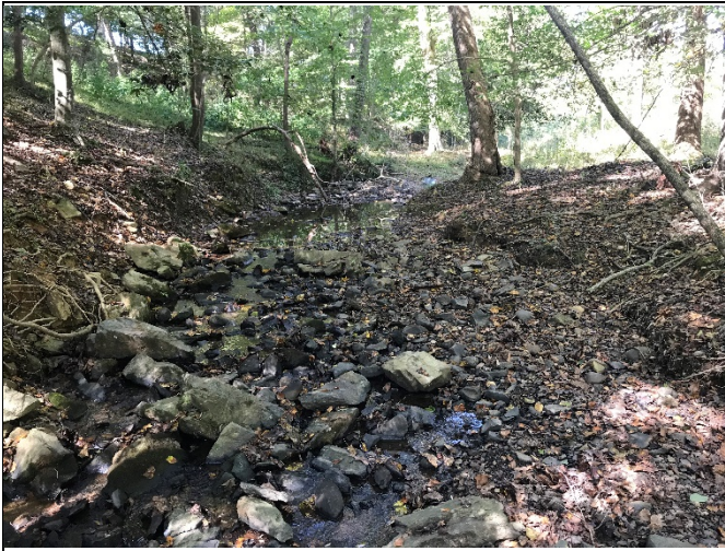
PP-13: Reach R4, view upstream, Station 38+50
