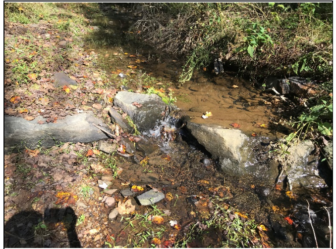
PP-14: Reach R4, view upstream, Station 43+50
