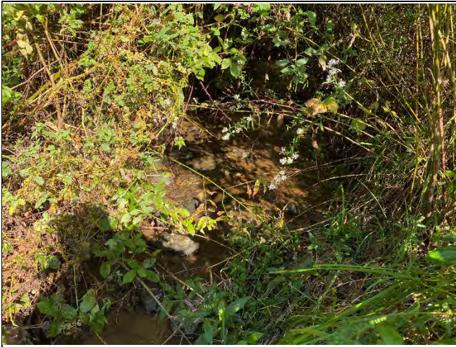
PP-3: Reach R5, view upstream, Station 13+75
