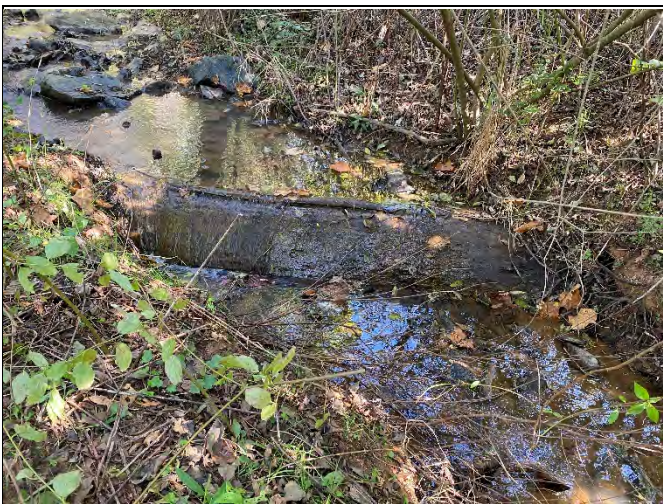
PP-5: Reach R5, view upstream, Station 17+25
