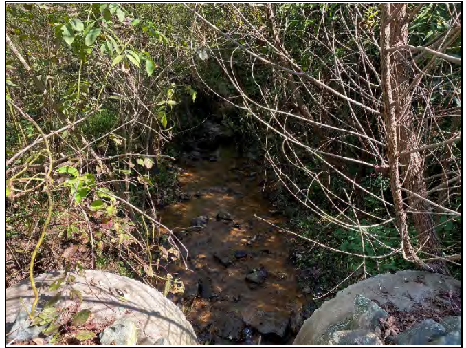
PP-8: Reach R5, view upstream of culvert crossing, Station 24+75
