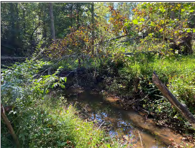
Reach R4 Station 43+50: Stabilizing and vegetating from previously documented bank scour from Hurricane Florence in Sept 2018 (photo from Oct 2020)
