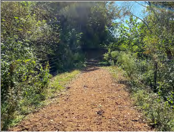
Pipe culvert crossing on lower Reach R5
