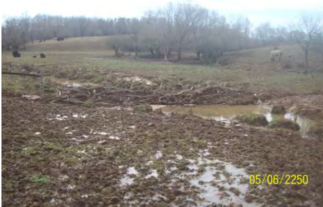
Looking downstream from farm crossing at debris hung up on fence line crossing.
