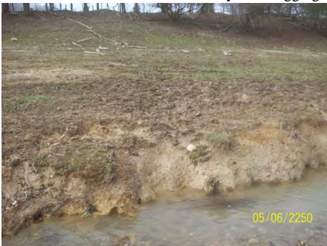
Looking at raw right bank along lower half of Reach 1
