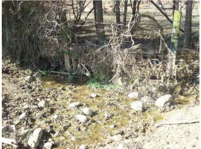
Looking upstream at fence line across Reach 7 that has accumulated debris and is holding minor amount of grade
