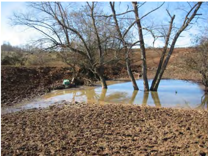
Looking towards Reach 2 from left floodplain. Debris on upstream side of culvert crossing has created backwater
