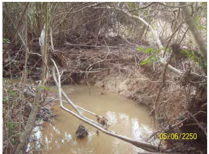
Looking downstream at raw outer meander bank of existing Reach 1
