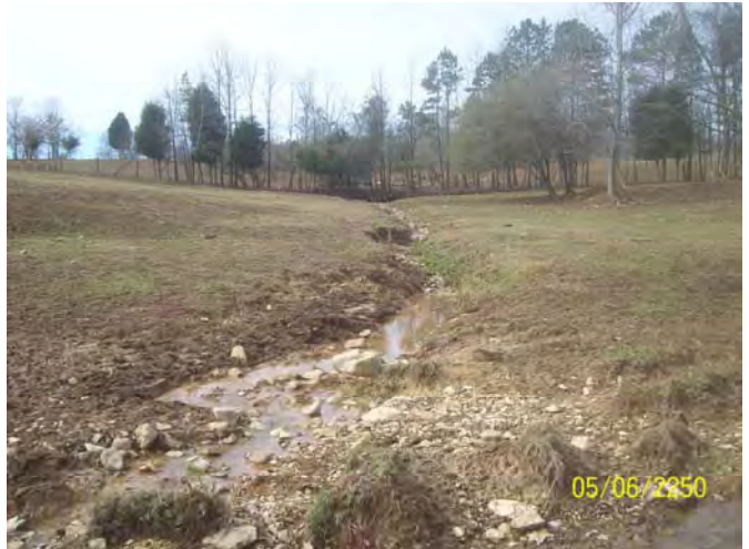
Looking upstream at downstream section of Reach 7 from the top of Reach 2
