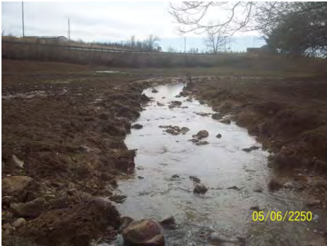
Looking downstream near top of Reach 2, channel is overwide
