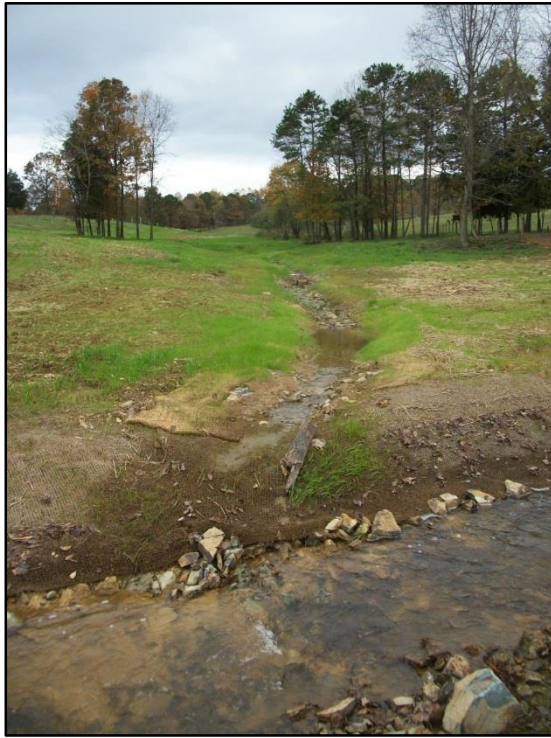
PID 9: Station 13+99 – Upstream (11/5/15)
