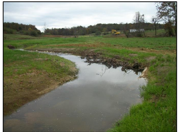
PID 21: Station 28+75 – Downstream (11/5/15)
