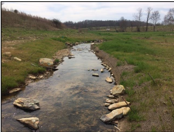
PID 20: Station 26+40 – Downstream (3/11/16)
