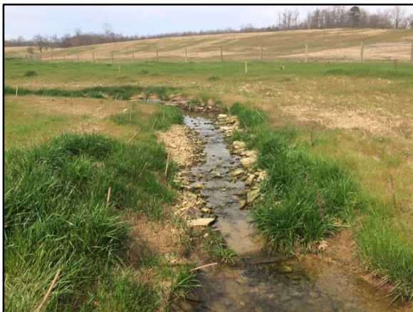
PID 23: Station 26+50 – Upstream (3/11/16)
