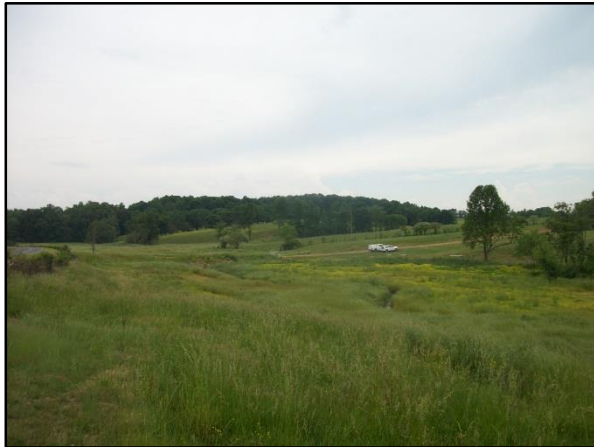
PID 23: Station 29+50 – Downstream Project View from Floodplain Knoll (5/11/16)
