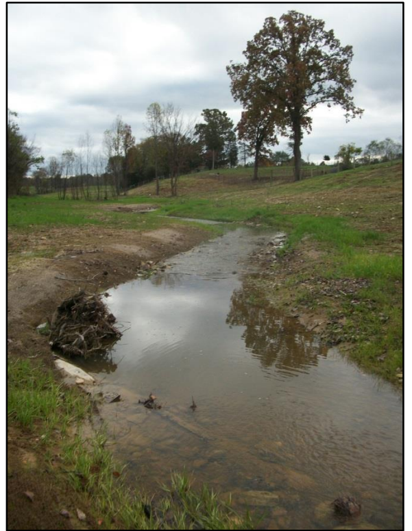
PID 4: Station 11+90 – Downstream (11/5/15)
