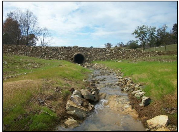
PID 15: Station 21+00 – Upstream (11/5/15)
