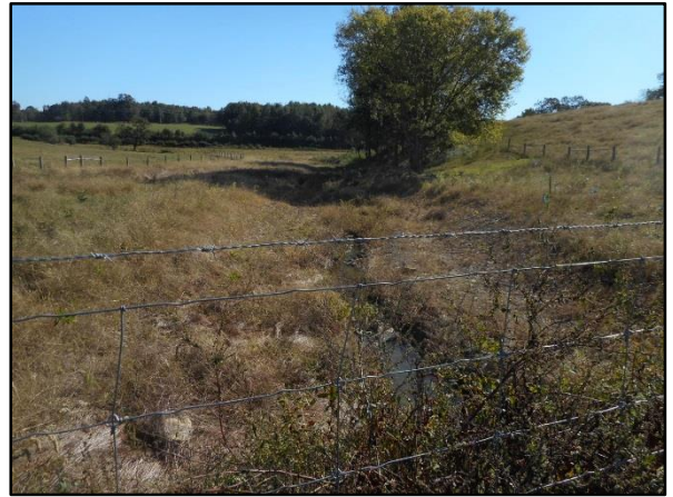
PID 14: Station 20+50 - Downstream (10/11/16)
