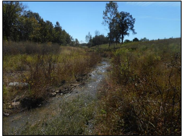
PID 2: Station 10+50 – Downstream (10/11/16)
