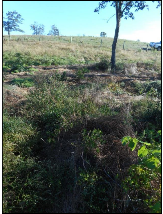
PID 2: Station 10+75 – Downstream (10/11/16)
