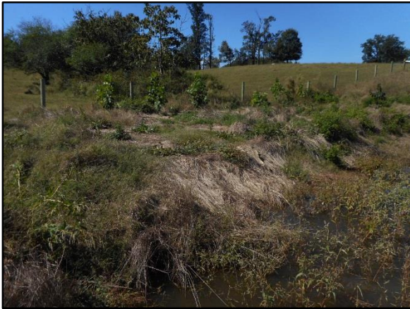
PID 1: Station 09+40: Upstream (10/11/16)
