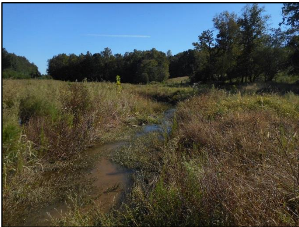
PID 31: Station 40+25 – Downstream (10/11/16)
