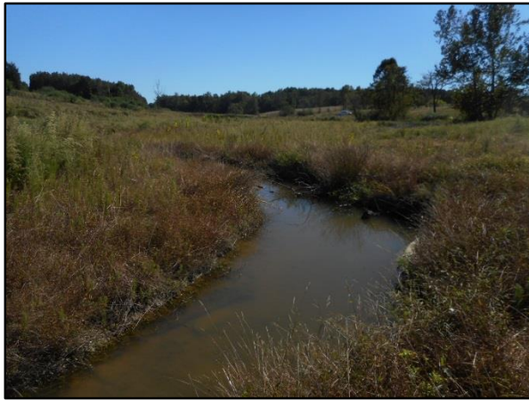
PID 21: Station 28+75 – Downstream (10/11/16)
