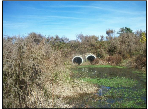
PID 27: Station 35+50 – Upstream (11/08/17)
