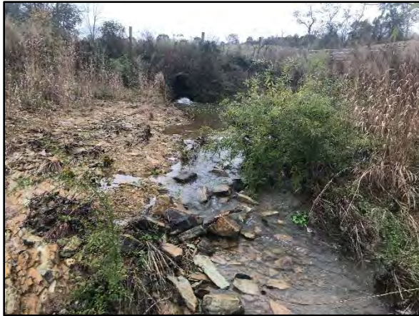
PID 15: Station 21+00 - Upstream (10/11/16)
