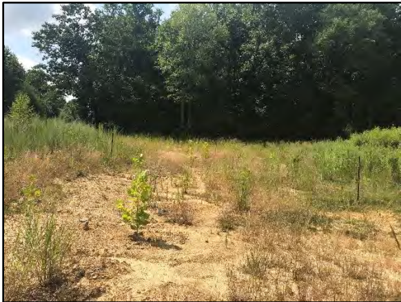
VPA 3-7 – Station 46+50 – Downstream photo of bare areas and areas of poor growth rates, as well as areas where supplemental plantings were installed. (07/17/18)
