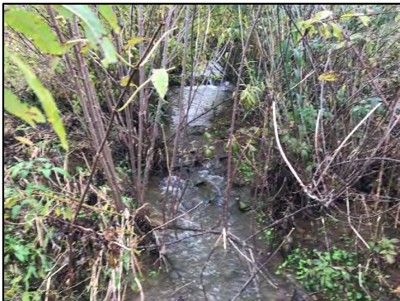
PID 11: Station 19+50 – Upstream (10/11/16)
