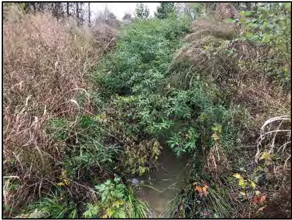
PID 7: Station 12+90 – Upstream (10/11/16)
