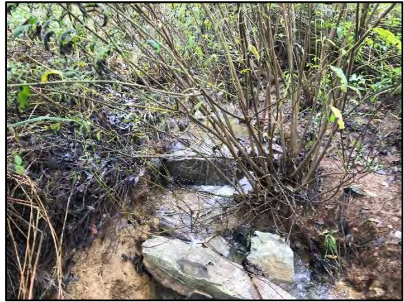
PID 6: Station 12+20 – Upstream (10/11/16)
