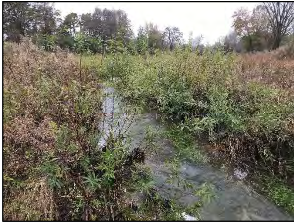
PID 14: Station 22+75 – Upstream (10/11/16)
