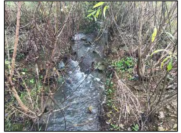
PID 16: Station 22+75 - Upstream (10/11/16)
