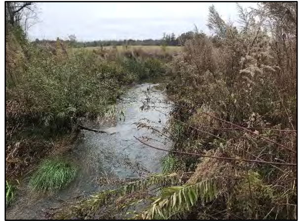
PID 33: Station 41+80 – Upstream (10/11/16)
