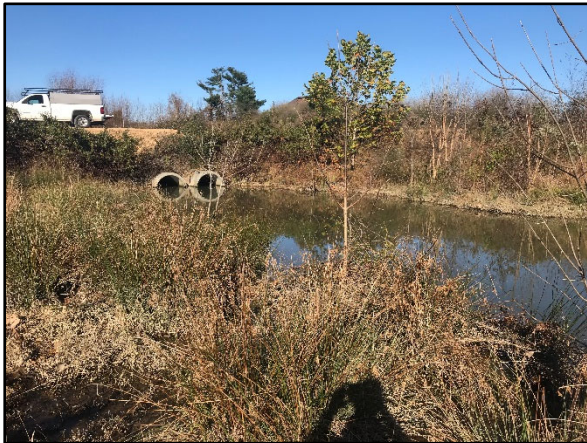
Reach 2 Culvert Downstream (11/18/20)
