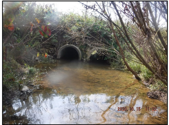
Reach 2 Culvert Upstream (10/15/20)
