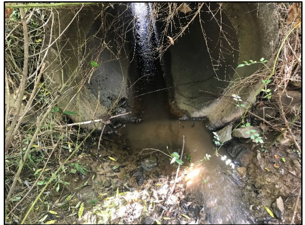
Reach 6 Culvert Upstream (10/15/20)
