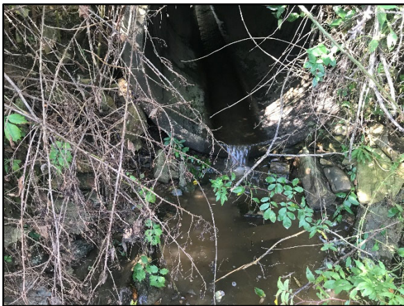
Reach 6 Culvert Downstream (10/15/20)
