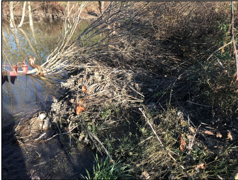
SPA 5-3 - Station 39+50 to 40+20 – Beaver dam caused water to back up and banks to lose vegetation (10/15/20)
