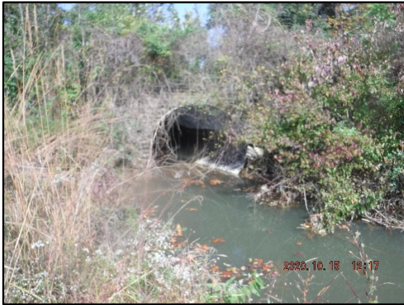
Reach 1 Culvert Downstream (10/15/20)
