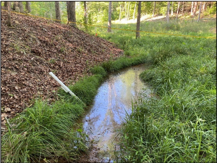
Flow Gauge UT1
