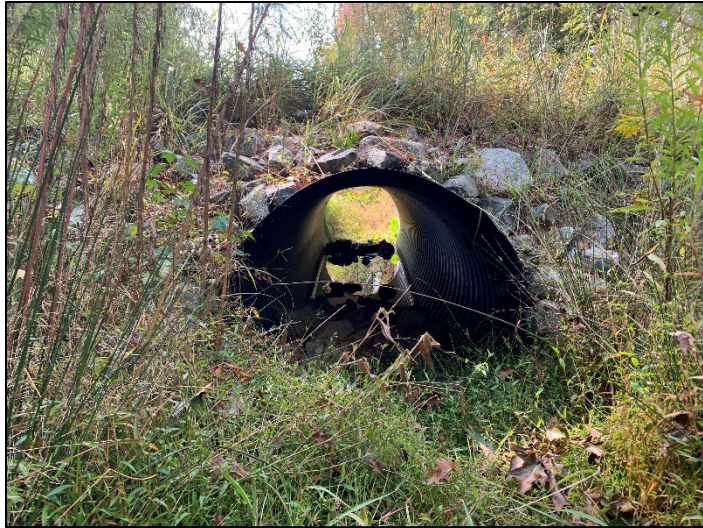
Crossing UTWB2 - Upstream
