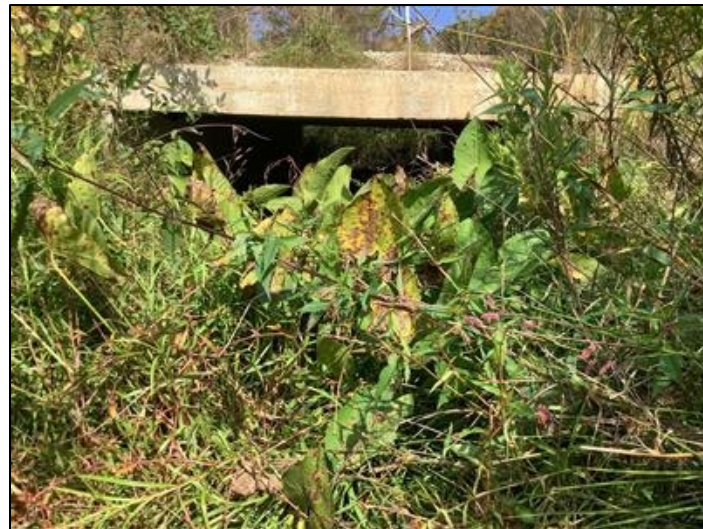
Crossing UTWB3 - Upstream
