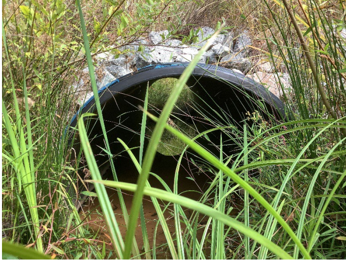
Crossing UT2-2 - Upstream
