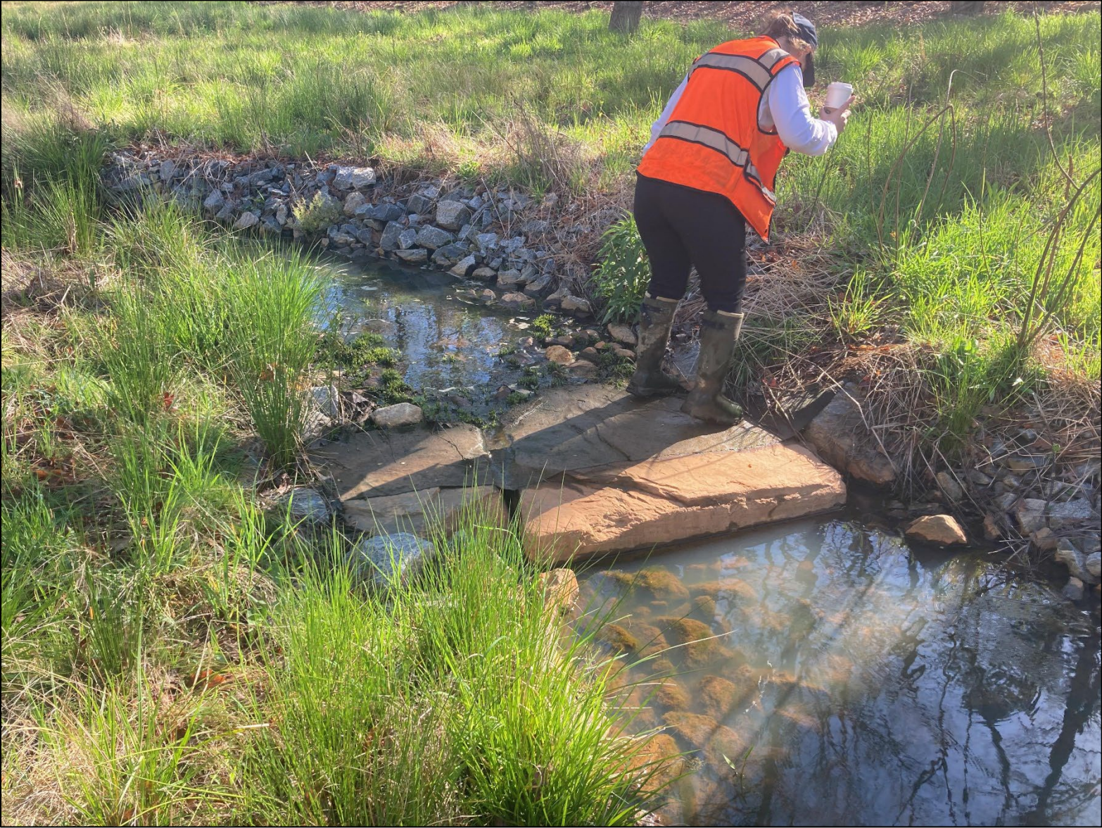
UTWB-2 Station 14+32 piping rock sill (4/4/2022)
