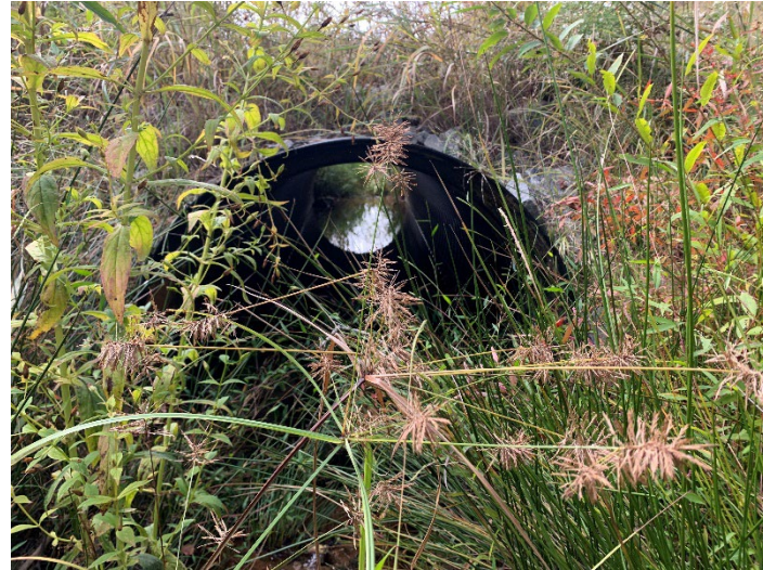
Crossing UT2-2– Downstream
