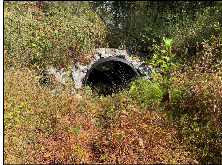
Crossing UTWB2– Downstream
