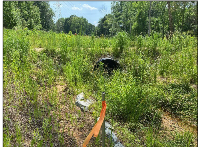
Photo Station 8 Crossing on UT2-2 looking downstream
