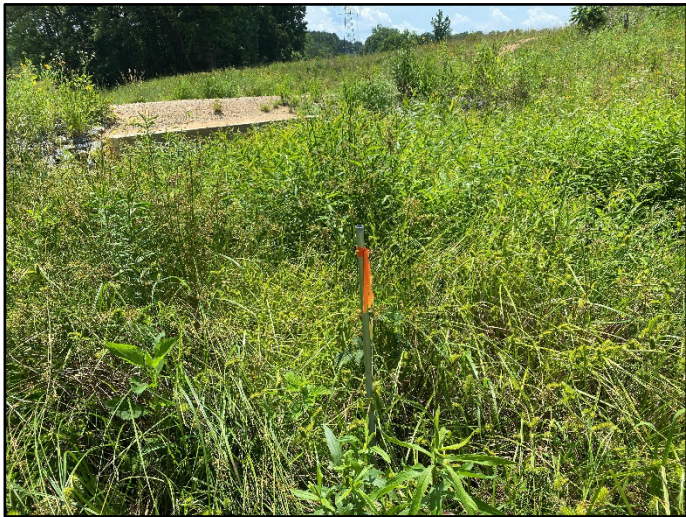
Photo Station 11 Crossing on UTWB-3 looking downstream
