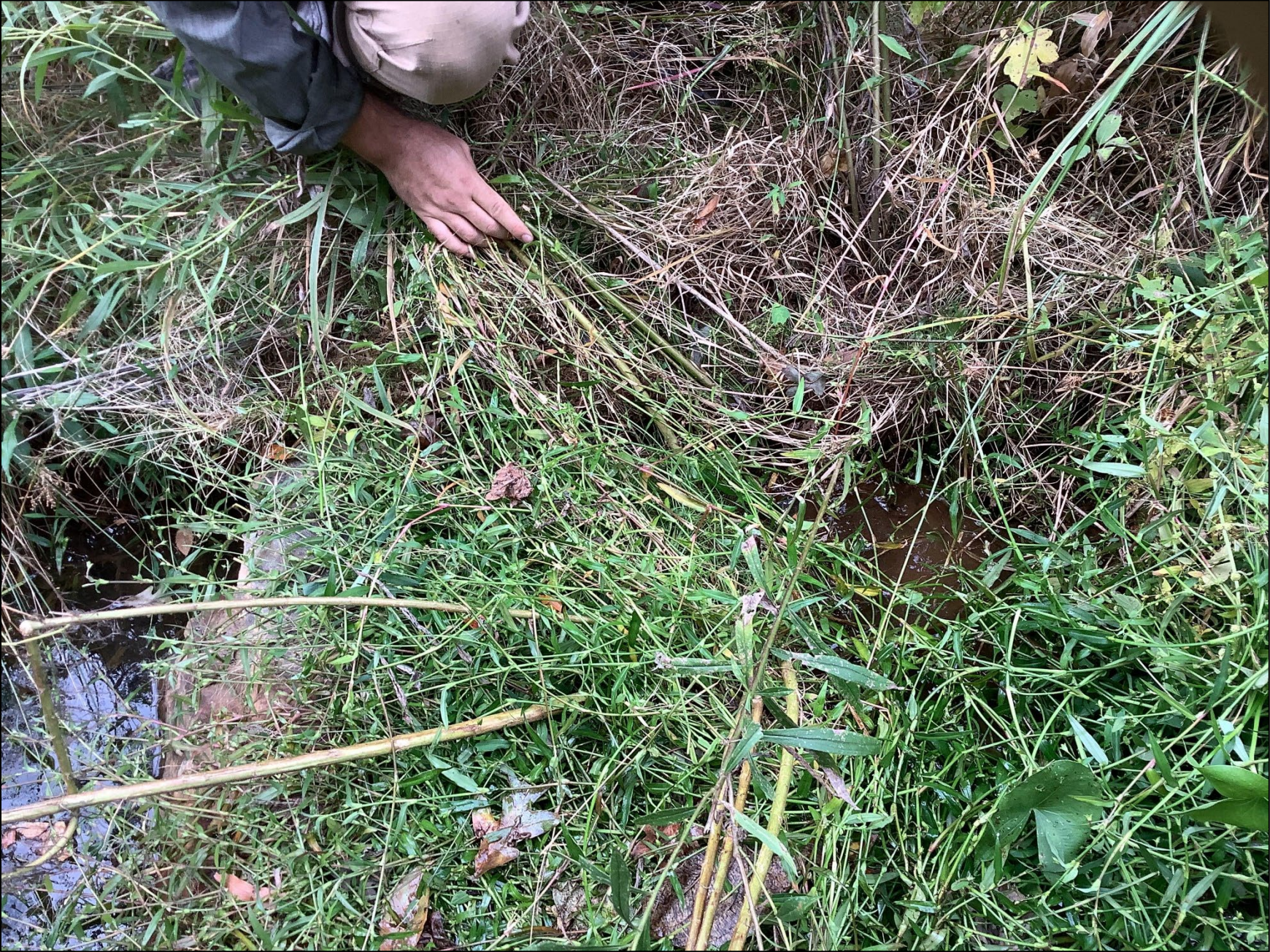
UTWB-2 Station 15+63 piping rock sill (10/10/2022)
