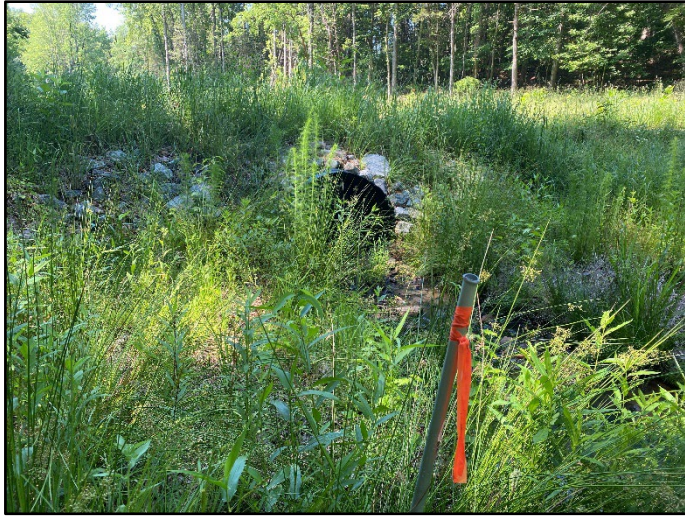
Photo Station 5 Crossing on UTWB-2 looking downstream
