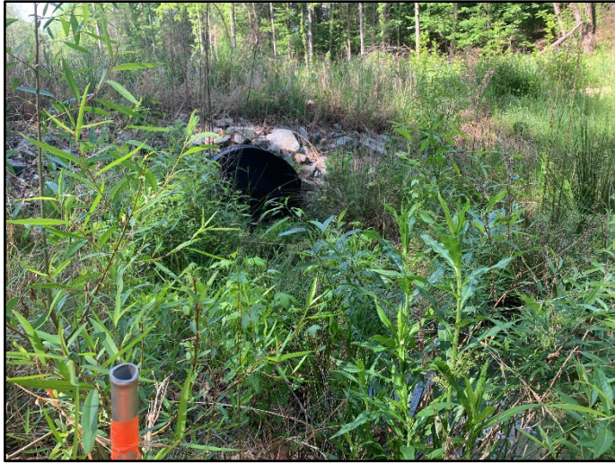
Photo Station 5 Crossing on UTWB-2 looking downstream
