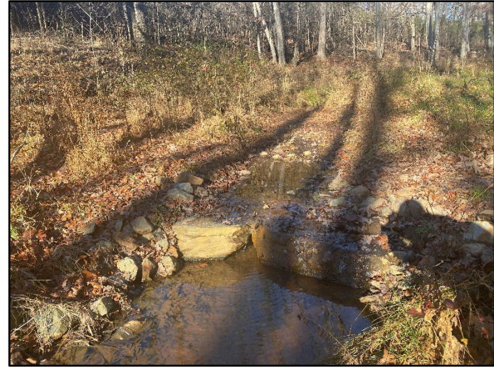
Piping Structure #2 - Repaired (12/3/2023)
