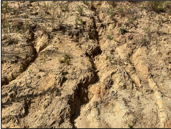
Side Slope Repair Area (10/10/2022)
