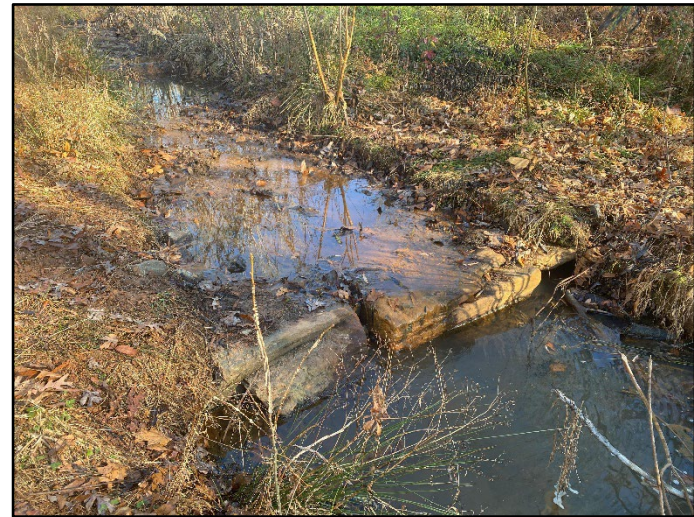
Piping Structure #4 - Repaired (12/3/2023)
