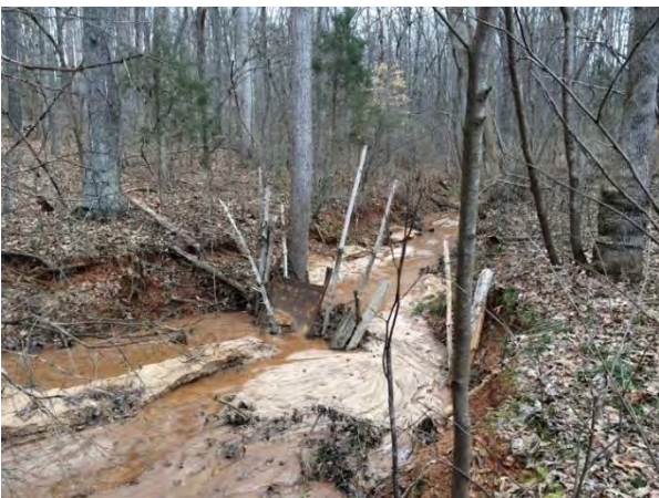
View looking at the upstream limits of UT2 at an existing fence. 1/20/16
