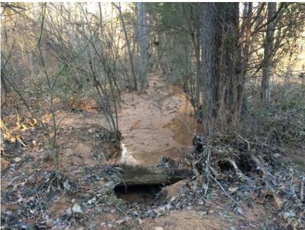
View looking upstream from existing stream crossing along UT2. 1/18/16
