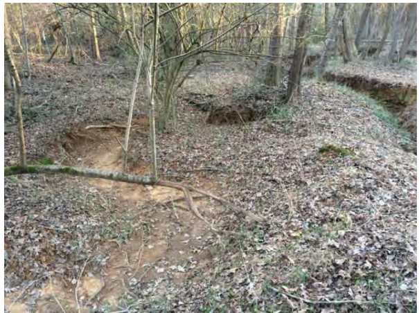
View looking at a secondary channel in the relic floodplain in the upper reach of UTWB. Note the old spoil to the right of secondary channel. 1/18/16
