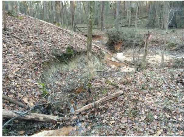
View of degradation along UT1 near the confluence with UTWB. 1/19/16
