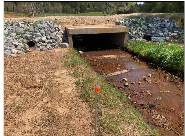
Photo Station 12 Crossing on UTWB-3 looking upstream
