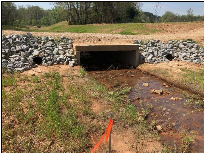
Photo Station 11 Crossing on UTWB-3 looking downstream
