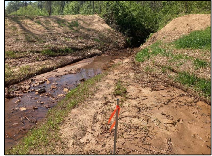
Photo Station 14 UTWB-3 exiting the project area
