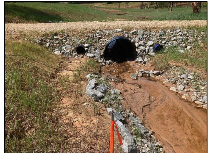
Photo Station 8 Crossing on UT2-2 looking downstream
