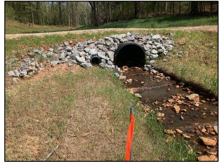
Photo Station 6 Crossing on UTWB-2 looking upstream
