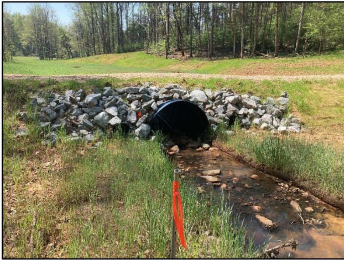
Photo Station 5 Crossing on UTWB-2 looking downstream
