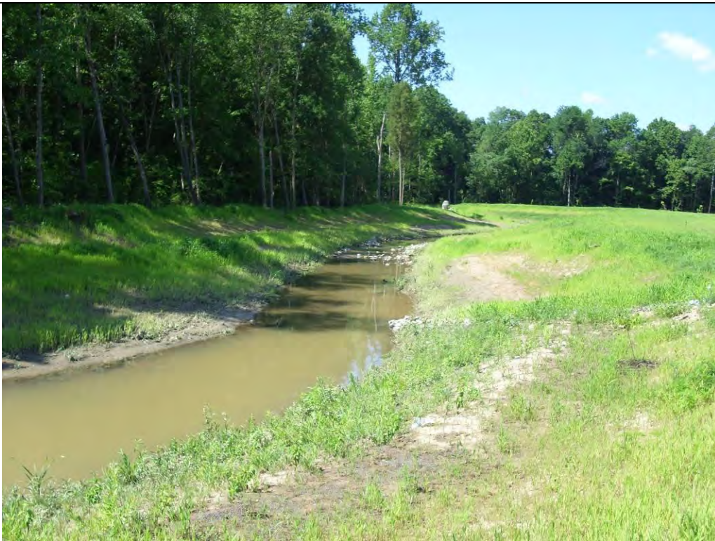
Monitoring Photo PA15: Looking downstream (July 1, 2008)
