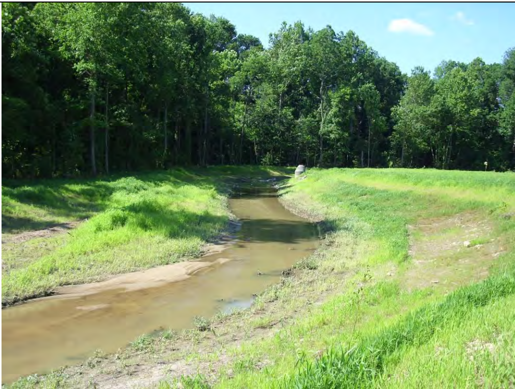
Monitoring Photo PA02: Looking downstream (July 1, 2008)
