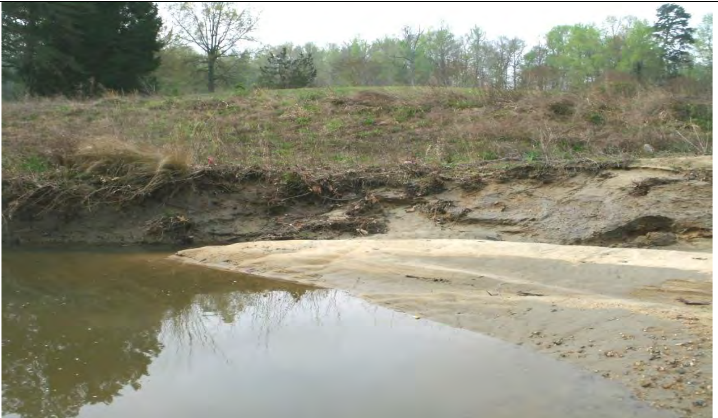
SP03 (2011) - Bank scour on left bank of Reach B (STA 151+475)
