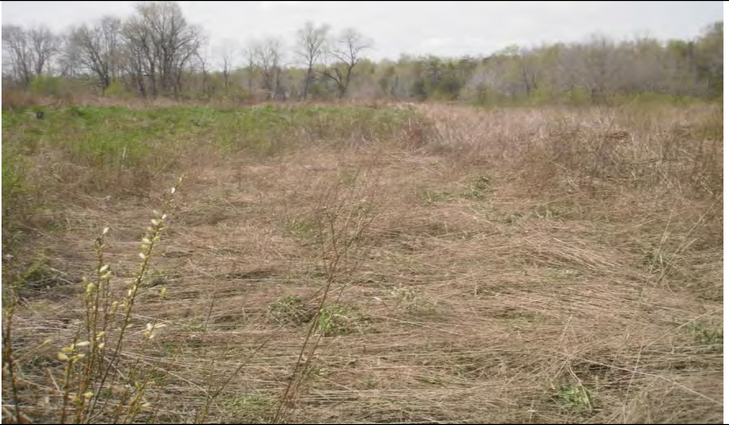
VP05 (2011) - Weak growth on left bank of Reach B (STA 152+450)
