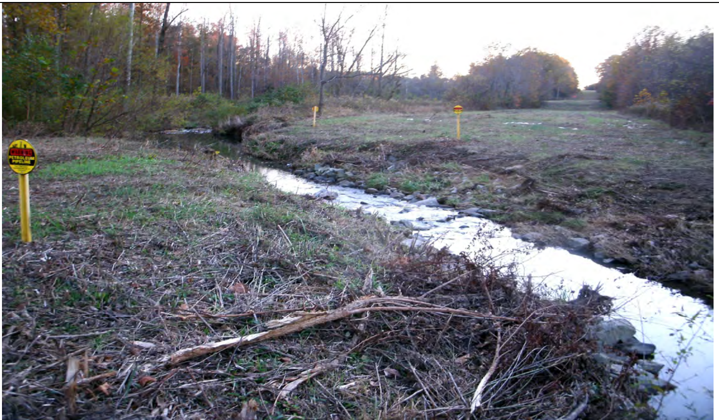
VP12 (2011) - Cleared utility easement at Reach Upper A (STA 61+50)
