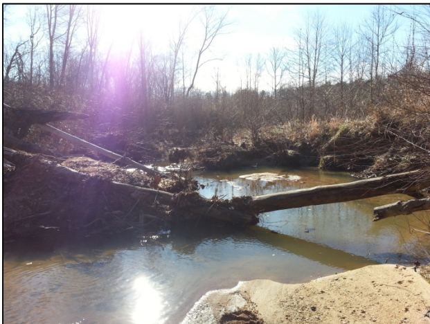
Bank erosion (Station 50+00) – 12/18/2013
