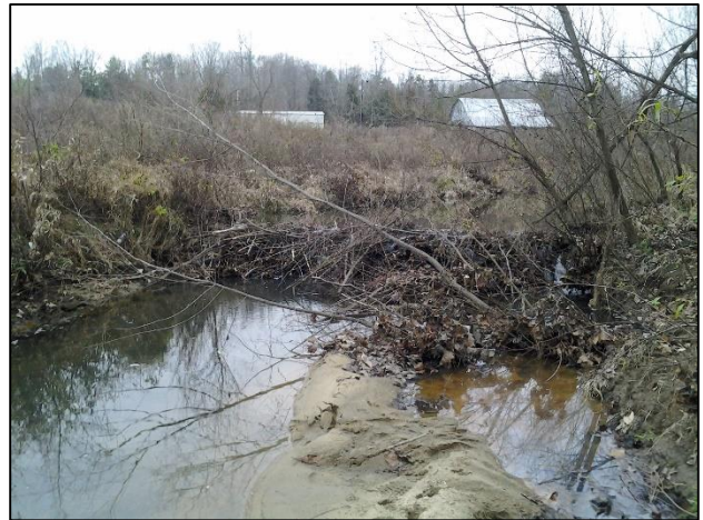
Beaver dam (Station 98+00) – 12/4/2014
