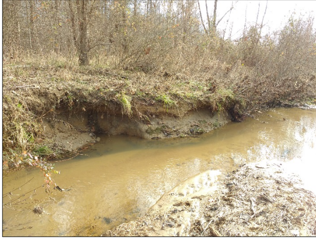
Bank erosion (Station 55+00) – 12/7/2015
