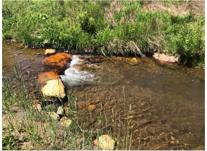
Vile Creek R2: STA 118+80 – J-Hook Repair 05-11-2022
