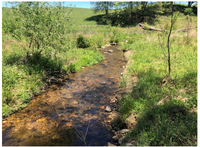
Vile Creek R2: STA 121+00 - 121+25 - Right Bank Repair 05-11-2022
