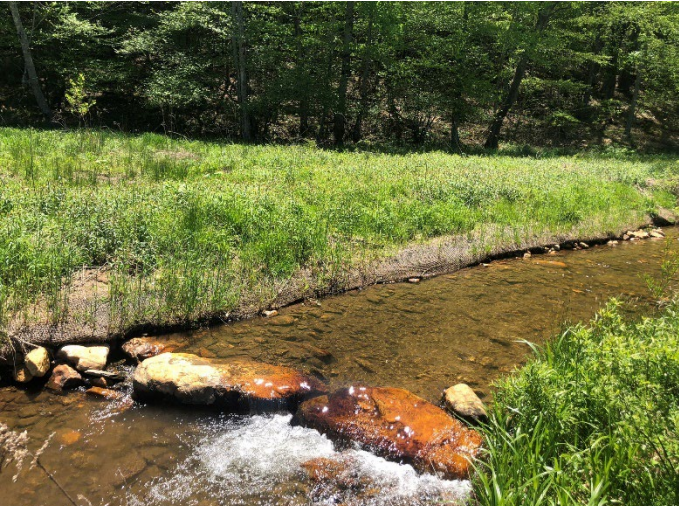
Vile Creek R2: STA 118+50 - 118+80 - Right Bank Repair 05-11-2022
