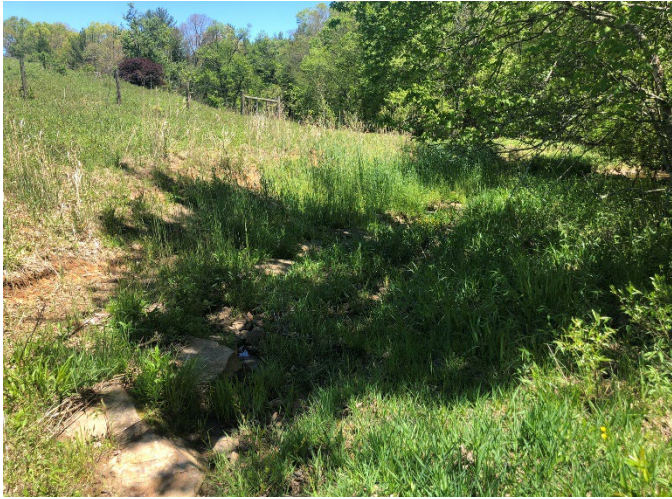
Vile Creek R3: STA 125+00 - 125+60 - Secondary Channel Repair 05-11-2022
