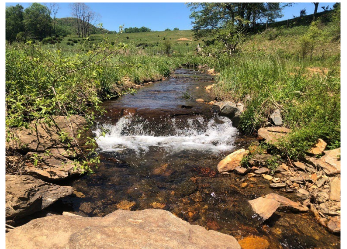
Vile Creek R2: STA 123+00 – Rock Sill Repair 05-11-2022
