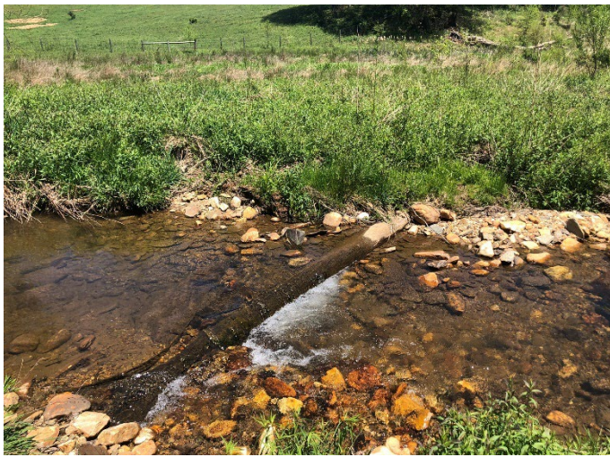
Vile Creek R2: STA 119+50 - 119+70 - Bank Repair 05-11-2022
