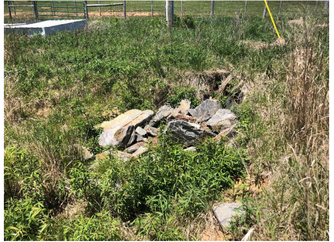
UT2 BMP – Headcut Repair 05-11-2022
