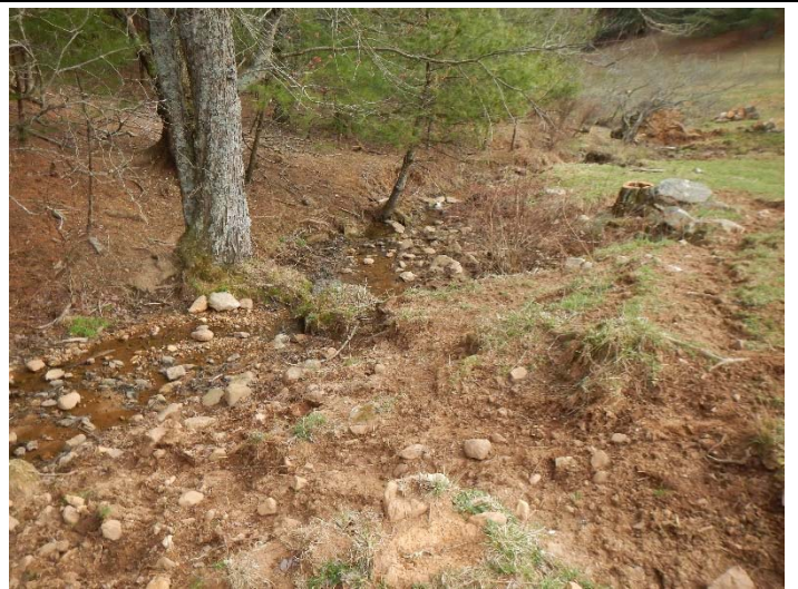
Photo Point 35 – view downstream UT3 (3/6/2017)
