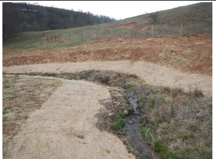
Photo Point 32 – view downstream UT2 (3/6/2017)
